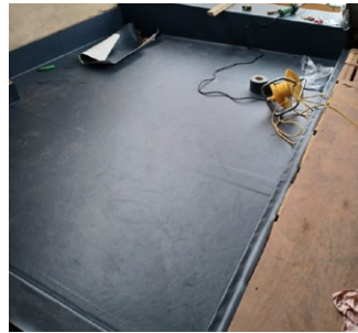
① Single ply membrane flat roof example
