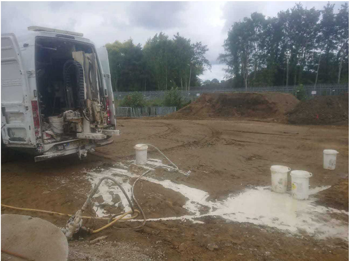
Surfacing of injection fluid at completion of hole
