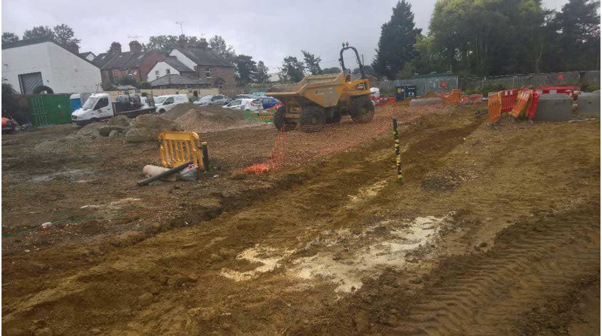
Surfacing of injection fluid at completion of hole
