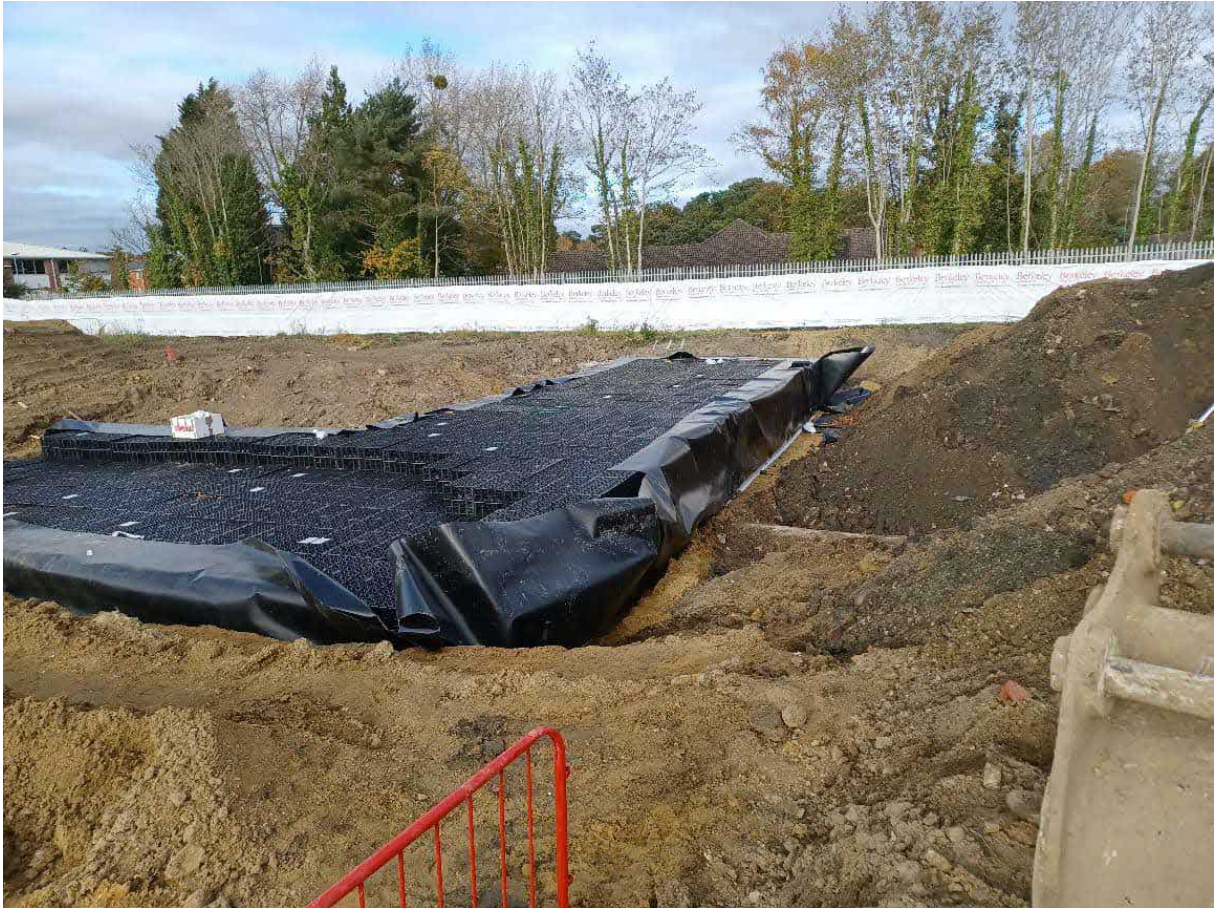
Contaminated soils being excavated from tank location
