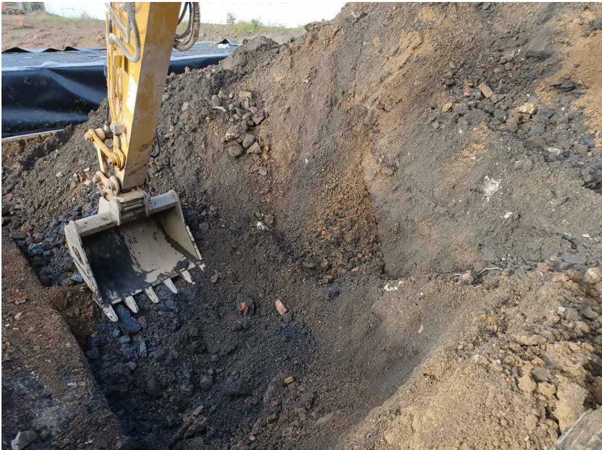
Contaminated soils being excavated from tank location
