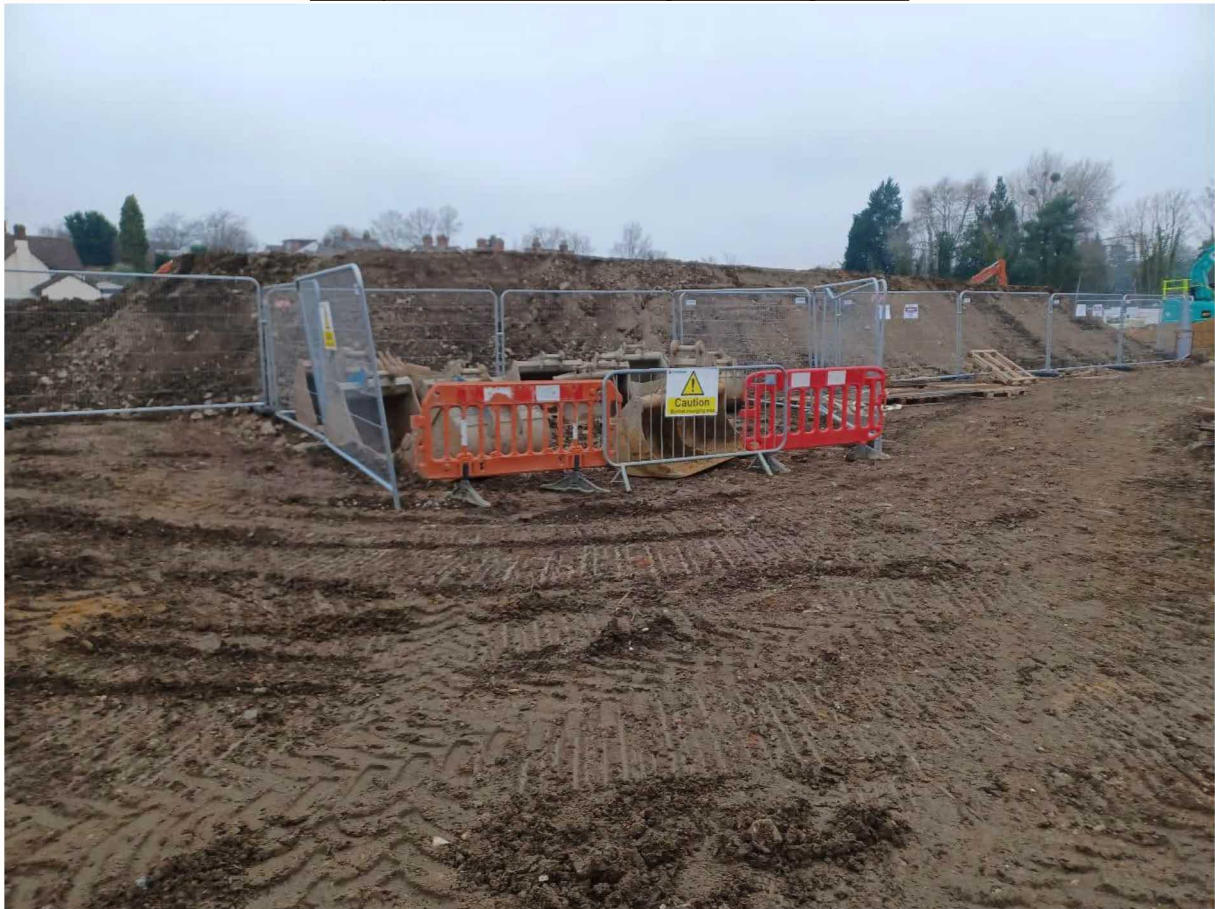
Stockpile of subsoil awaiting re-use in gardens
