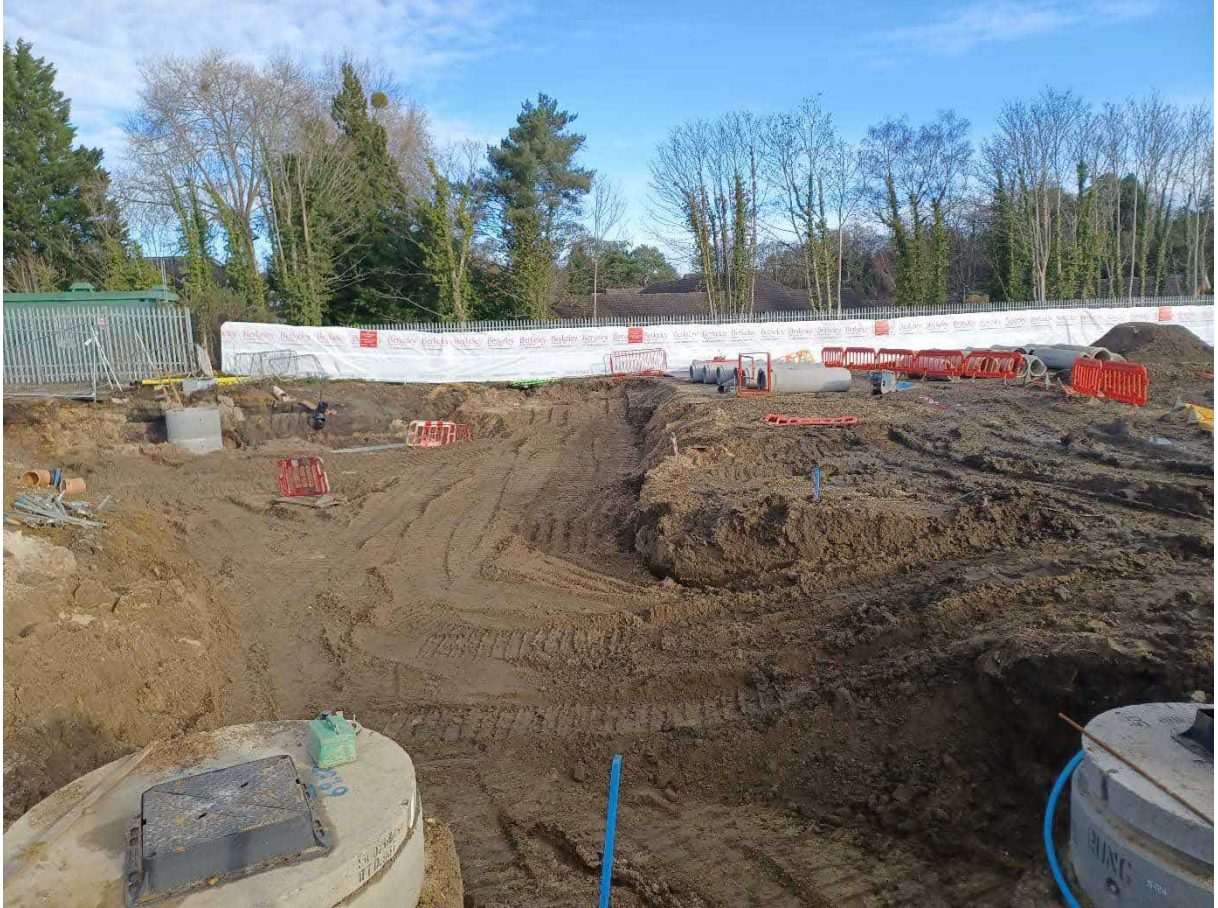
Backfilling of sewer trench, north of the site
