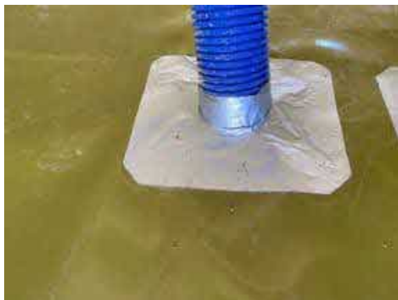
Plot 45 typical pipe penetration seal using SAGM.
