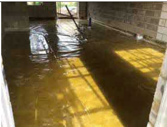
Plot 7 overview of installed membrane.
