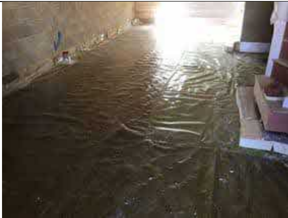
Overview of installed membrane to plot 65.
