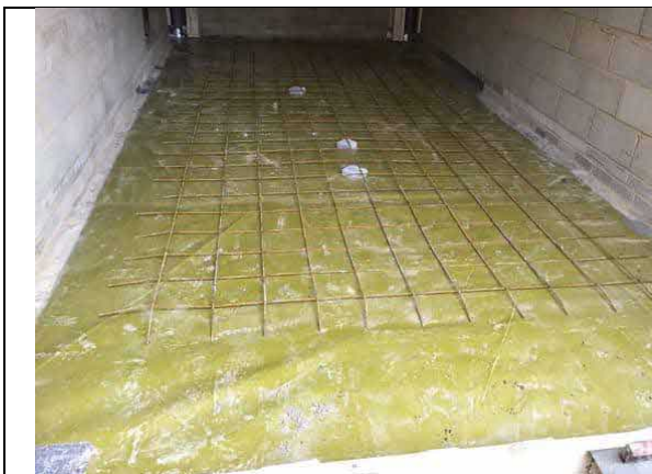
Overview of installed membrane to garage area in plot 45.
