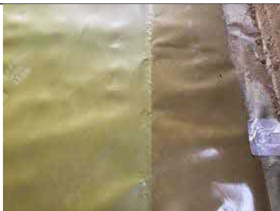
Hand welded membrane lap to plot 36.
