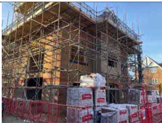
Plot 74 Overview where installation took place.
