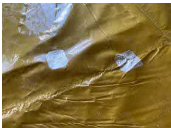
Plot 30 - Patch repairs using SAGM.
