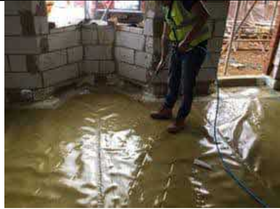
Air lance testing to Plot 10 lap joints.
