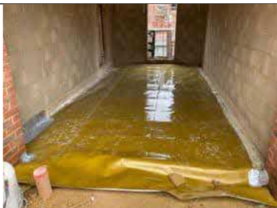
Overview of Visqueen HC Blok infill installation to Plot 35 Garage.
