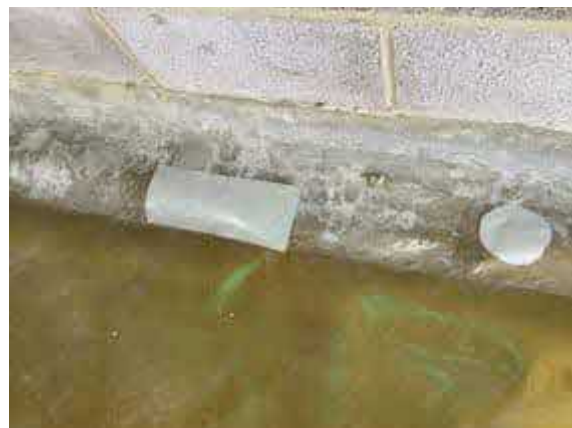
Plot 4 patch repair using SAGM.
