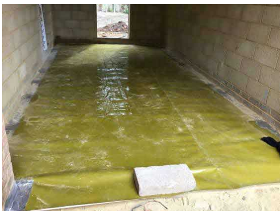
Overview of installed membrane in garage plot 67.
