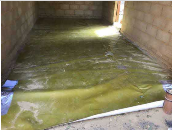
Overview of installed membrane to the garage, as an infill to plot 73.
