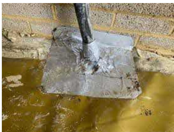
Plot 32 garage. Typical pipe penetration sealed using SAGM.
