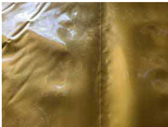
Plot 4 hand welded membrane lap.
