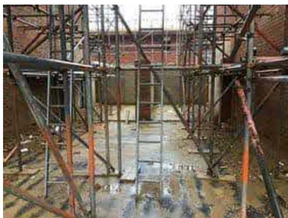
Scaffolding in place in all garages.
