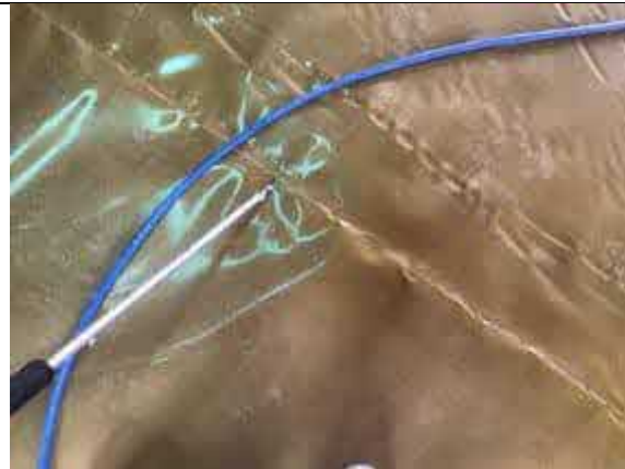
Plot 9 hand welded joint being air lanced
