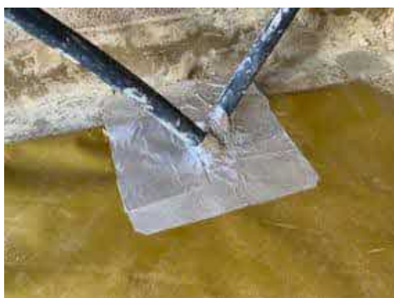
Plot 29 - Pipe penetration's sealed using SAGM.
