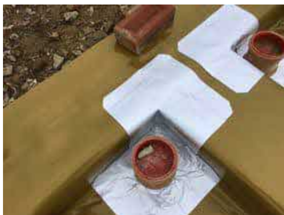
Plot 5 typical corner and pipe penetration seal using SAGM.
