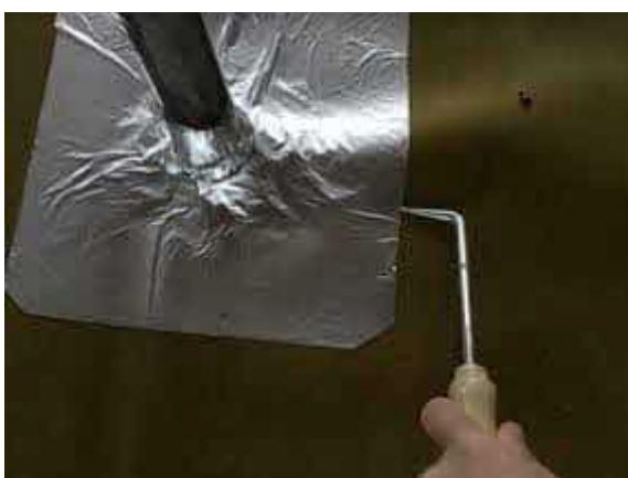
Pick testing all SAGM detailing to plot 38.
