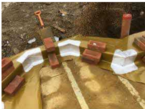
Plot 7 typical bay window corner seals using SAGM.
