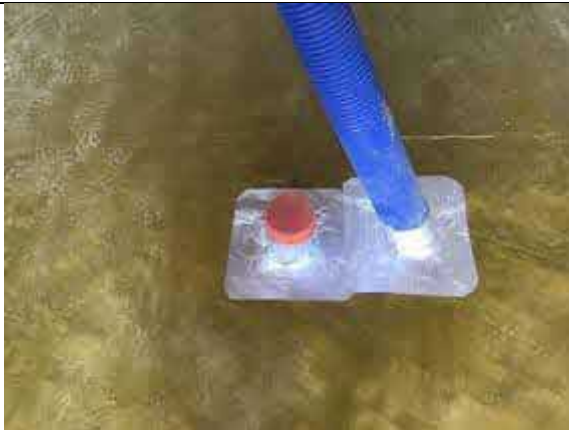
Plot 9 pipe penetrations sealed using SAGM
