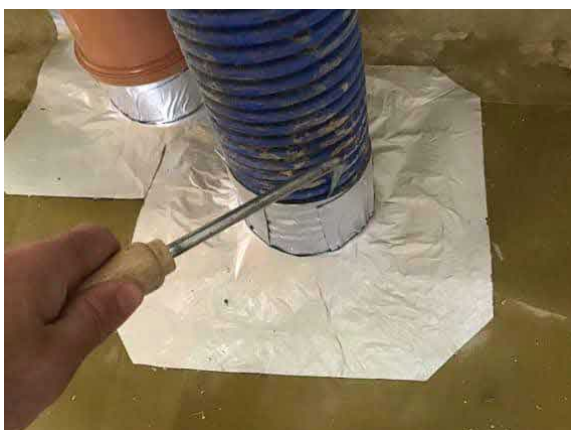
Pick testing all SAGM detailing in plot 52.
