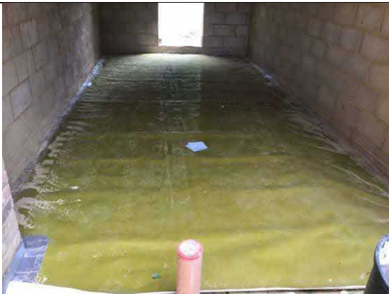
Overview of installed membrane to the garage, as an infill to plot 69.
