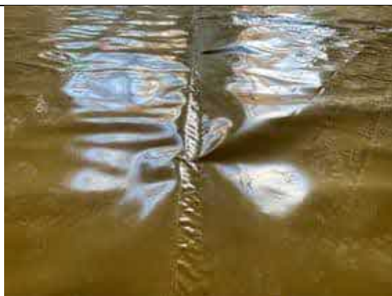
Plot 30 - Hand welded membrane lap joint.
