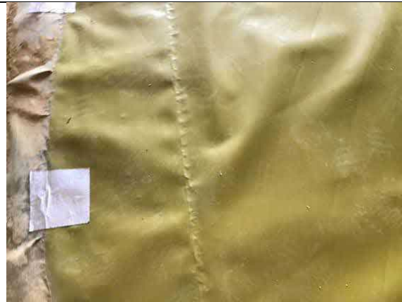
Hand welded membrane lap in garage plot 40.
