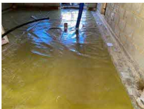
Plot 45 overview of installed membrane.
