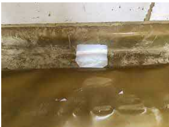
Plot 7 patch repair using SAGM.
