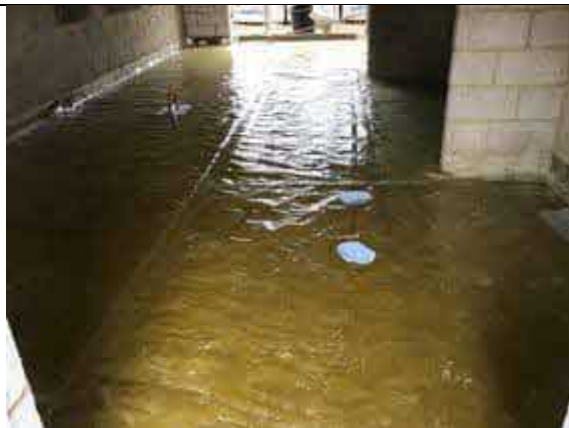
Plot 33 overview of installed Visqueen HC Blok Gas Barrier as an infill.
