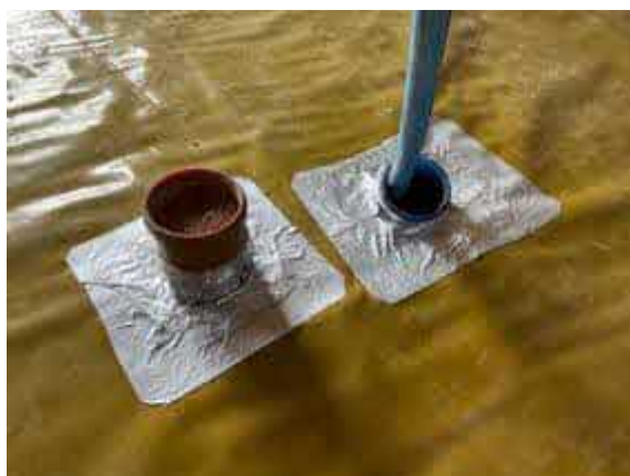
Plot 30 - Typical pipe penetration's sealed using SAGM.
