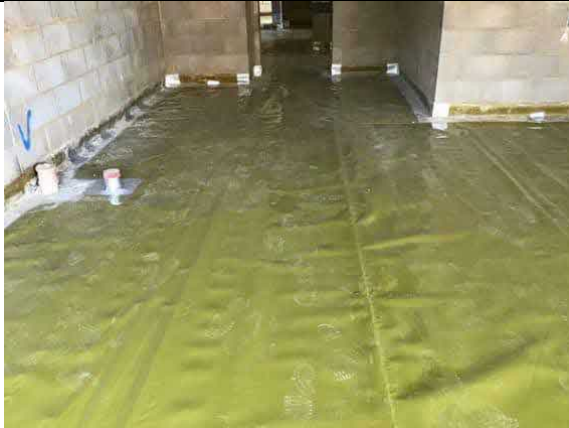
Overview of installed Visqueen HC Blok gas membrane, that has been installed as an infill to Apartment block H.
