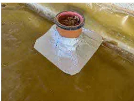
Plot 73. Typical pipe penetration sealed using SAGM.
