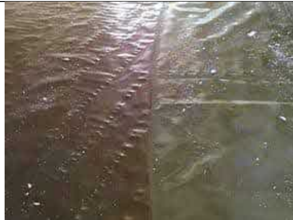
Hand welded membrane lap to plot 65.
