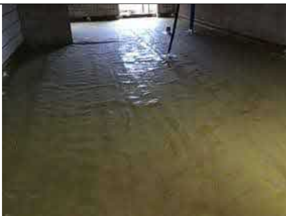
Overview of installed membrane to plot 37.
