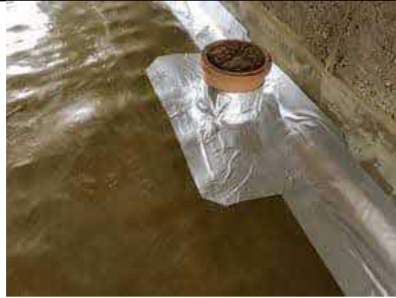
Plot 28 typical pipe penetration seal using SAGM.
