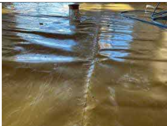
Plot 73. Hand welded membrane lap joint.
