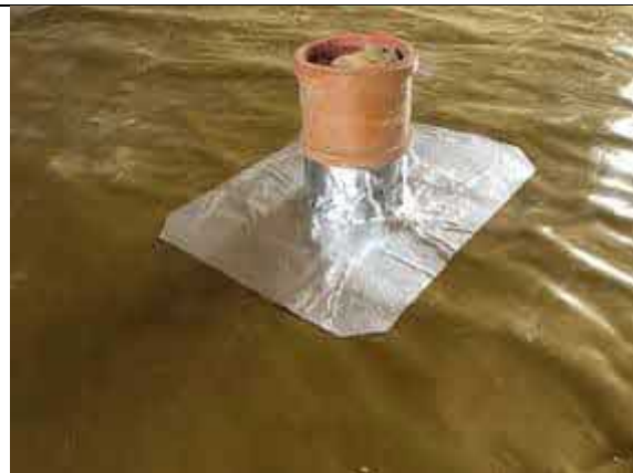
Plot 33 typical pipe penetration seal using SAGM.
