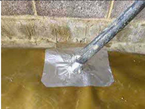
Pipe details within Plot 11 sealed with SAGM.
