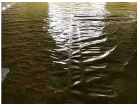
Plot 33 hand welded membrane lap.
