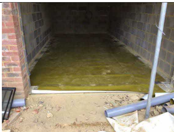
Overview of installed membrane in garage plot 64.
