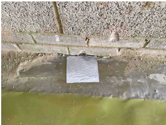
Patch repair using SAGM to damaged perimeter membrane in plot 41 garage.
