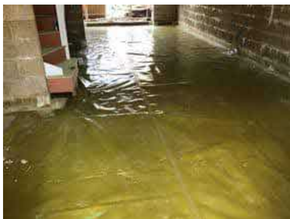
Overview of installed membrane to plot 49.
