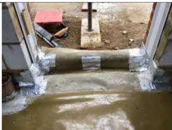
Door threshold seal using SAGM.
