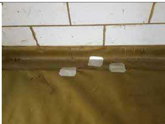
Patch repairs using SAGM to plot 36.
