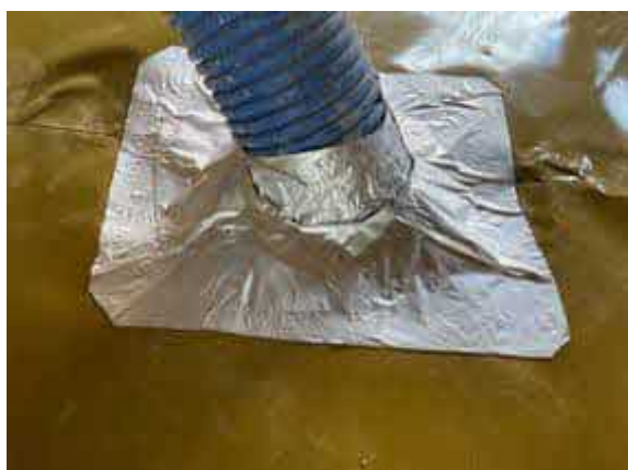
Plot 40. Typical pipe penetration sealed using SAGM.
