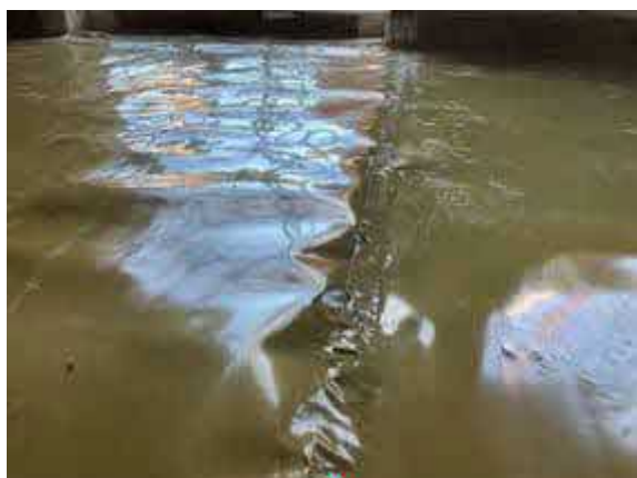
Plot 40. Hand welded membrane lap joint.
