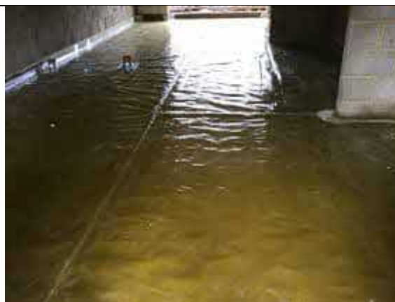
Overview of installed membrane to plot 28.
