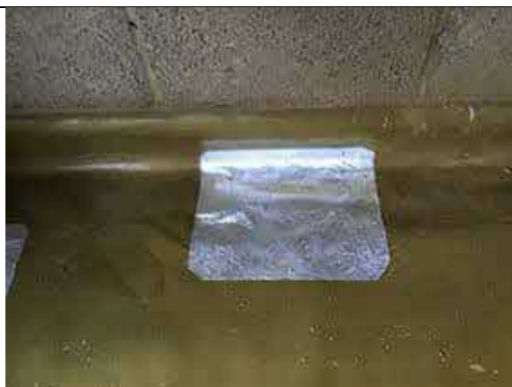
Repaired damaged perimeter membrane using SAGM to plot 39.
