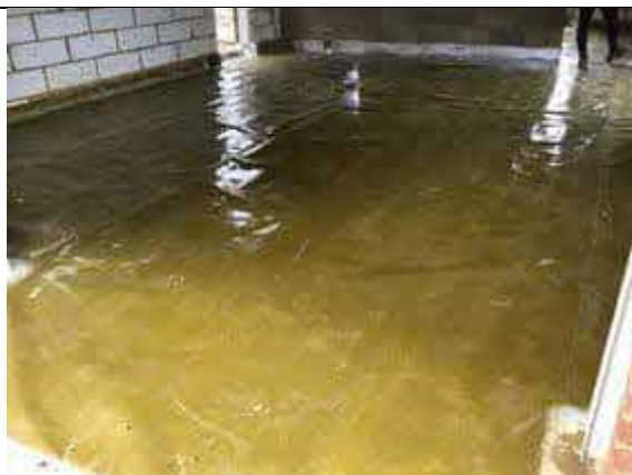
Overview of installed membrane.
