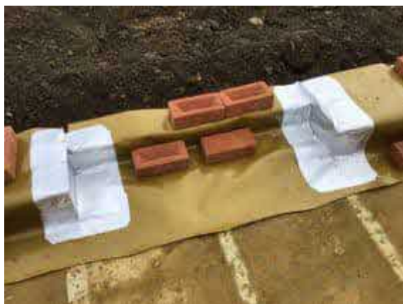
Plot 7 typical door seal using SAGM.
