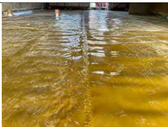
Plot 29 - Successfully hand welded membrane lap joint.
