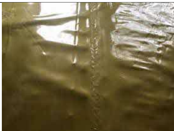
Hand welded membrane lap to plot 64.
