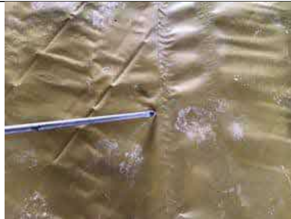
Plot 34 air lancing all welded membrane laps.
