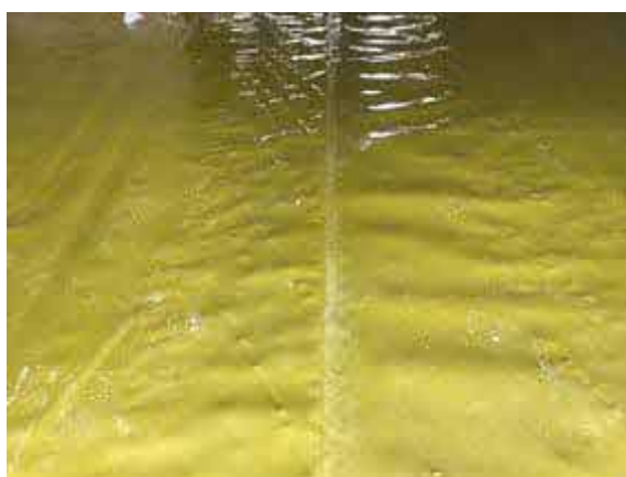
Hand welded membrane lap to plot 48.
