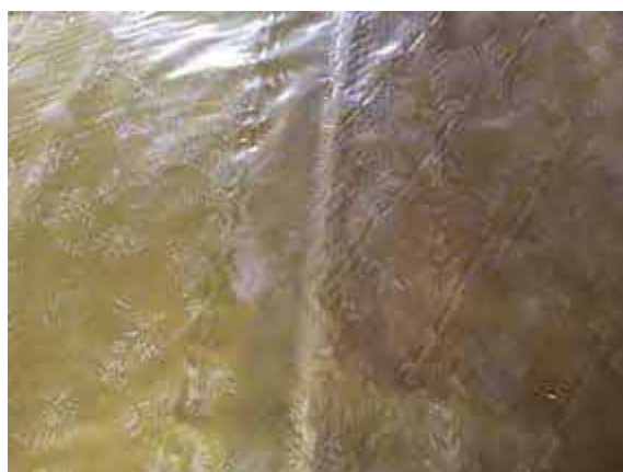
Plot 35 hand welded membrane laps.
