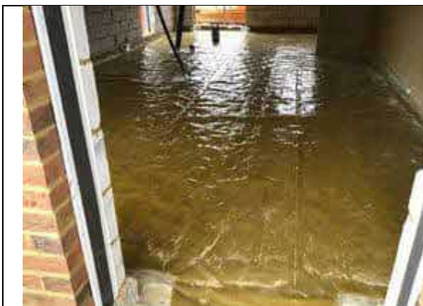
Overview of installed membrane to plot 27.
