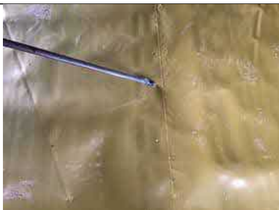
Air lancing all welded membrane laps.
