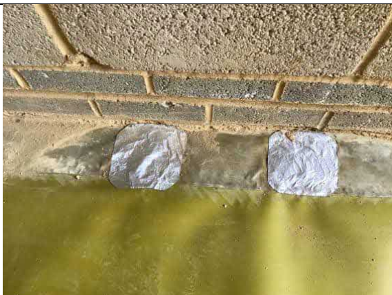
Patch repairs using SAGM to damaged perimeter membrane.
