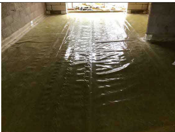
Hand welded membrane lap in plot 51.
