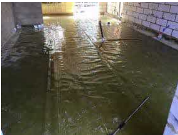
Overview of installed membrane to plot 67.
