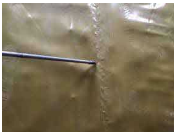
Air lancing all hand welded membrane laps to plot 64.
