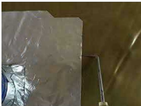
Pick testing all SAGM detailing to plot 64.
