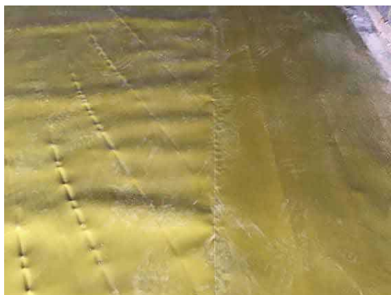
Typical hand welded membrane lap.
