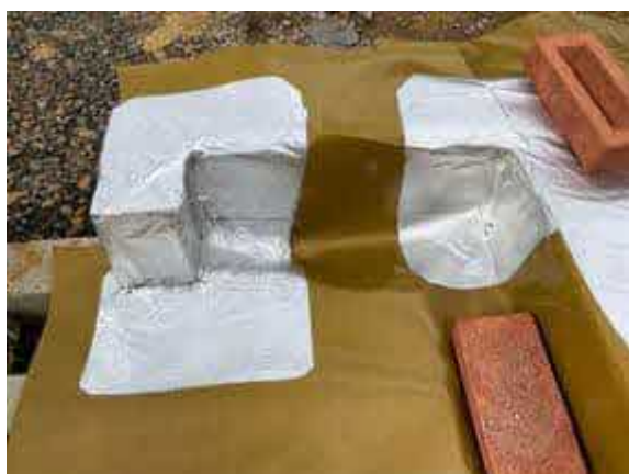
Plot 63 FOG Unit - Corner detailing sealed using SAGM.
