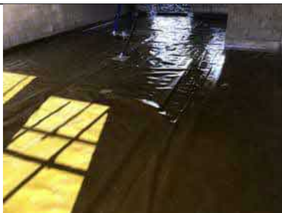
Plot 3 overview of installed membrane.
