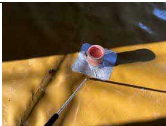
Plot 74. Air lance integrity test conducted upon sealed pipe penetration.
