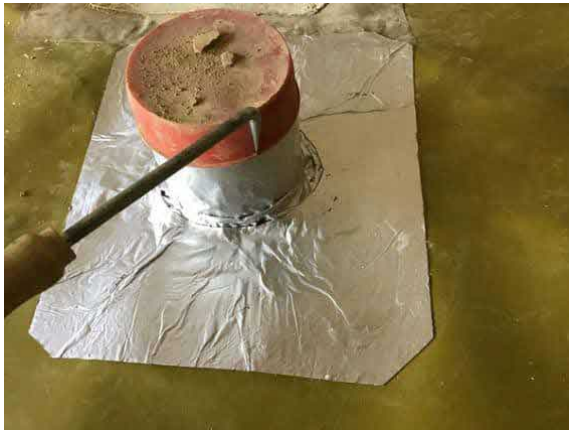
Pick testing all SAGM detailing in apartment block H.
