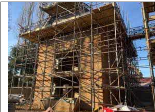
Plot 73 Overview where Visqueen HC Blok was installed.
