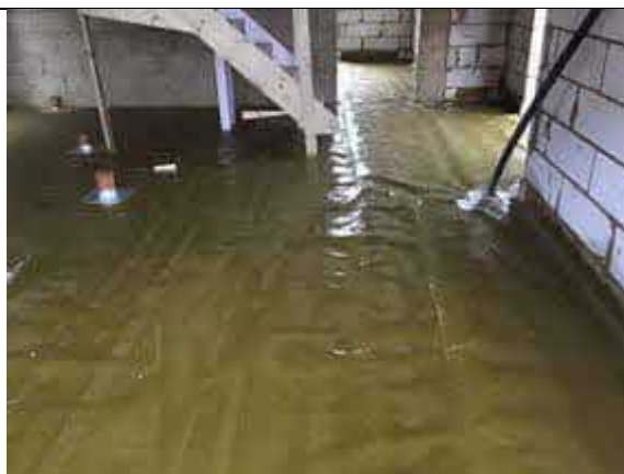
Overview of installed membrane to plot 36.
