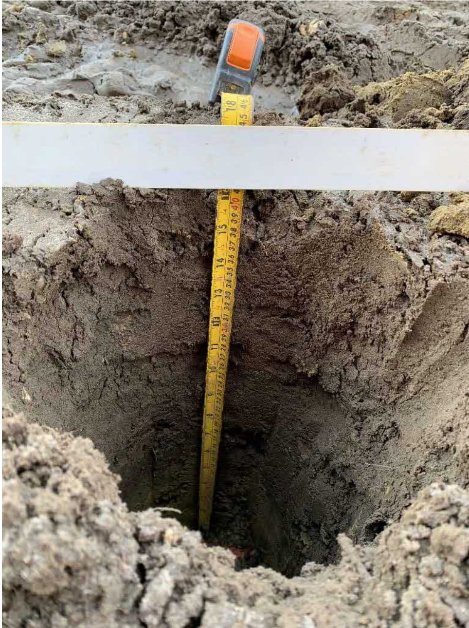
Block H Landscaping area capping layer with geotextile visible
