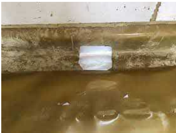
Plot 7 patch repair using SAGM.
