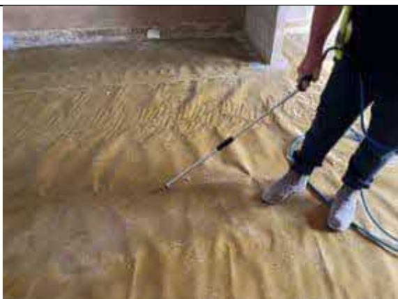
Plot 30 - Air lance test conducted upon all membrane lap joints.
