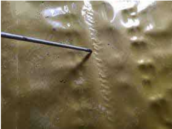
Plot 32 air lancing all welded membrane laps.
