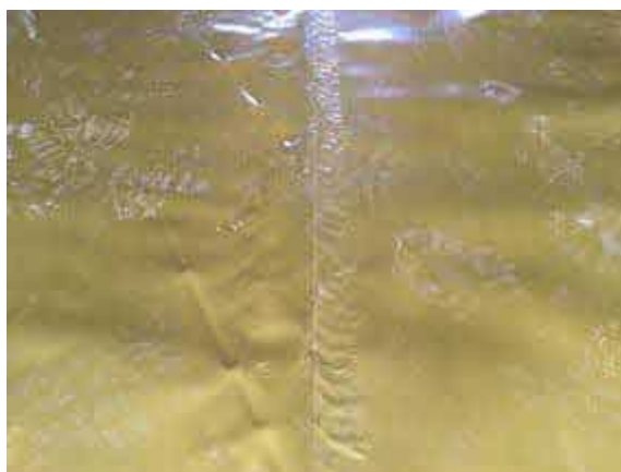
Overview looking down the hand welded lap joint.
