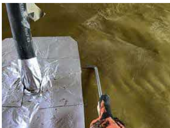
Plot 35 pick testing all SAGM detailing.
