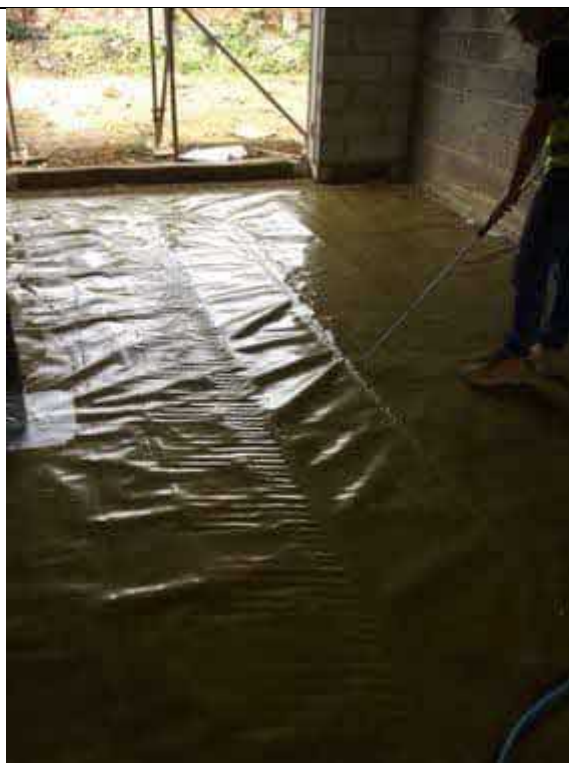
Overview to the air lance test in process to Plot 11.
