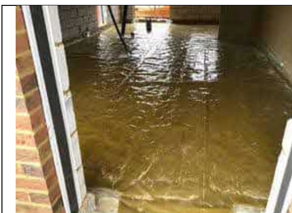
Overview of installed membrane to plot 27.
