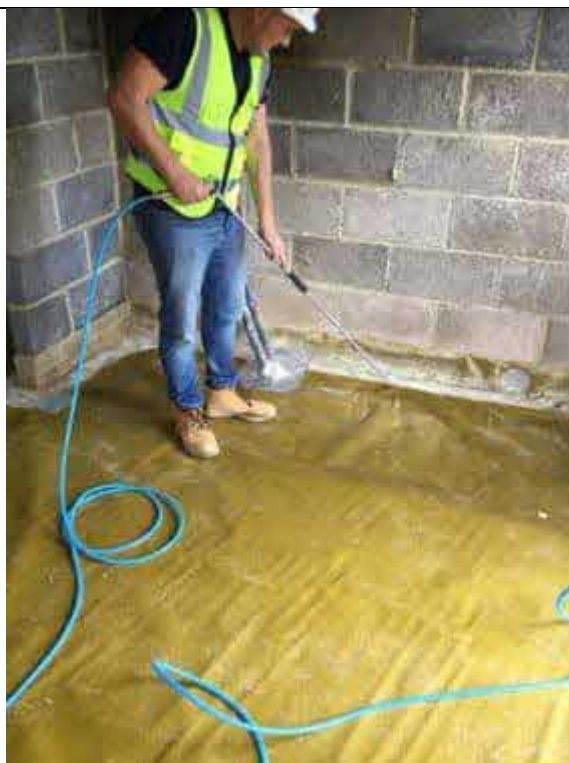
Lance testing to the perimeter hand welded lap joints.
