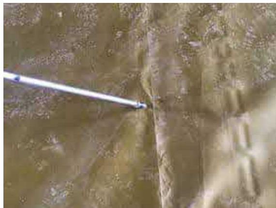
Plot 7 air lancing all welded membrane laps.
