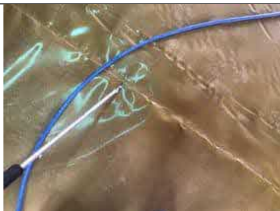
Plot 9 hand welded joint being air lanced
