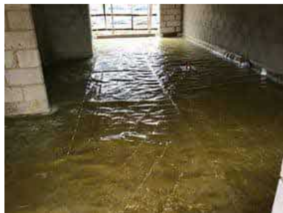
Plot 34 overview of installed Visqueen HC Blok Gas Barrier.
