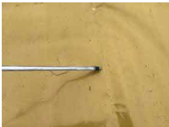
Air lancing all weld laps and SAGM detailing.
