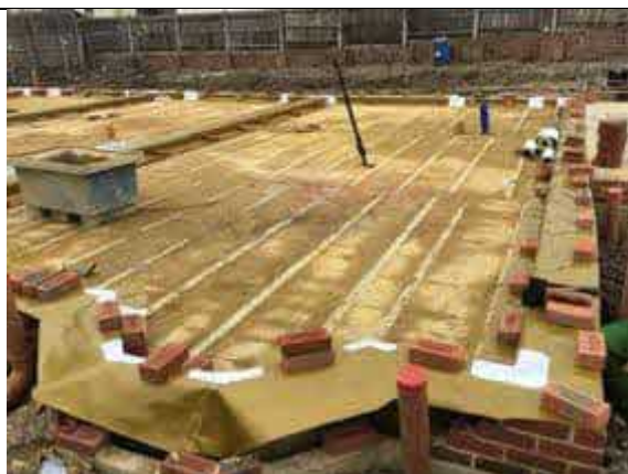
Plot 7 overview of installed membrane.
