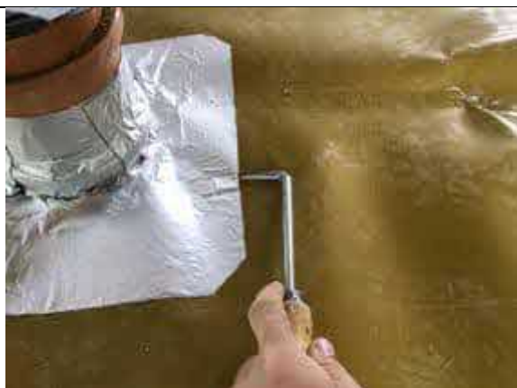
Pick testing all SAGM detailing.
