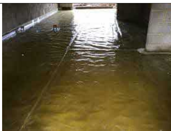
Overview of installed membrane to plot 28.
