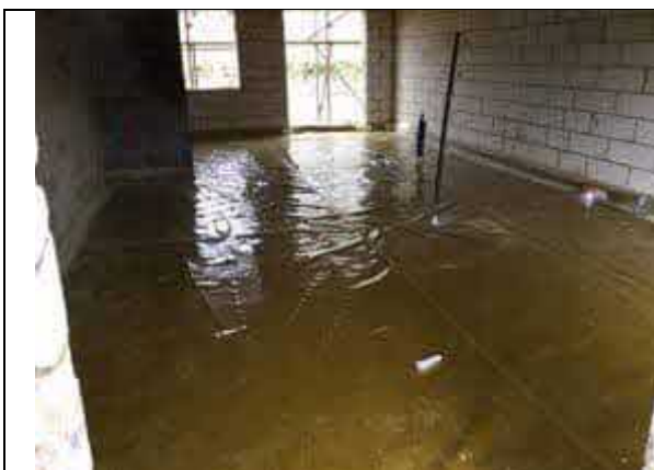
Overview to Plot 12 infill lined out using Visqueen HC Bloc.
