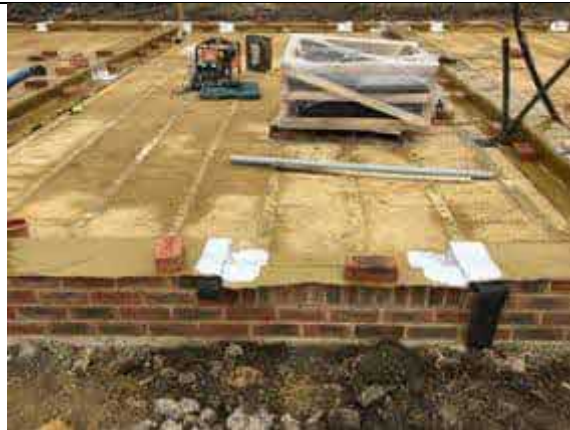
Plot 5 overview of installed membrane to the perimeter and party walls.
