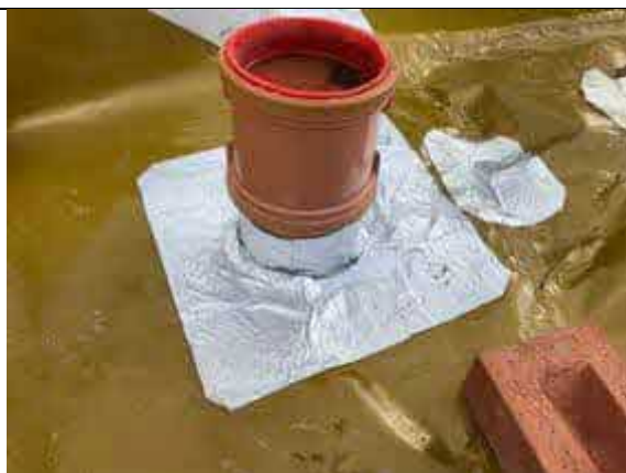
Plot 63 FOG Unit - Typical pipe penetration sealed using SAGM.
