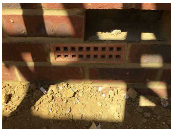
Plot 5 air brick in place at the time of our inspection.
