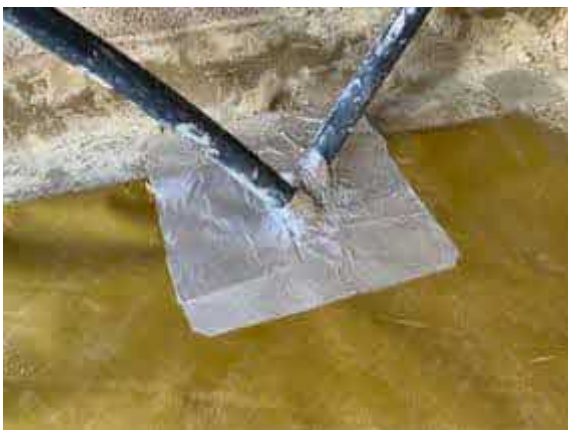
Plot 29 - Pipe penetration's sealed using SAGM.
