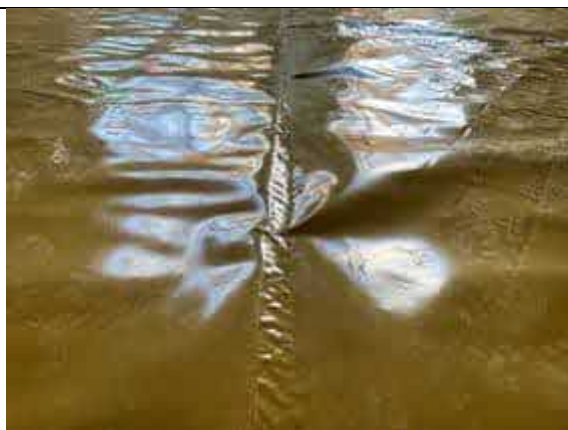
Plot 30 - Hand welded membrane lap joint.
