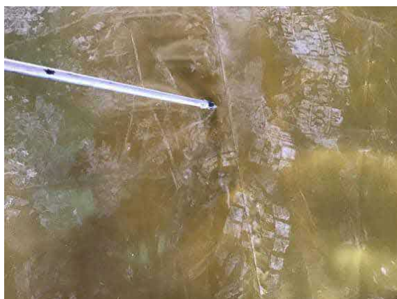
Plot 5 air lancing all SAGM detailing and welded membrane laps.
