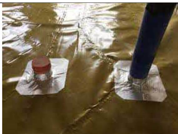
Two typical pipe details sealed with SAGM to Plot 12.
