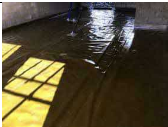
Plot 3 overview of installed membrane.
