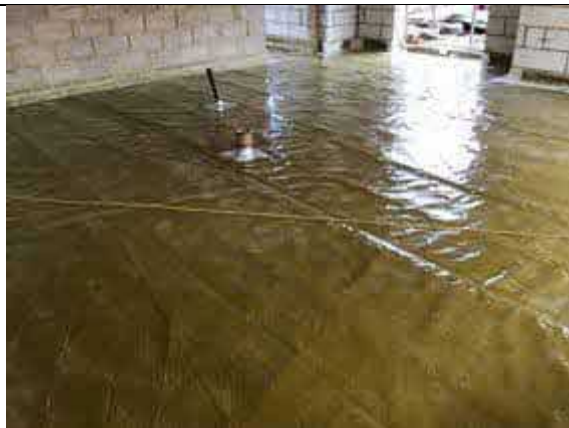
Plot 75 overview of installed membrane.
