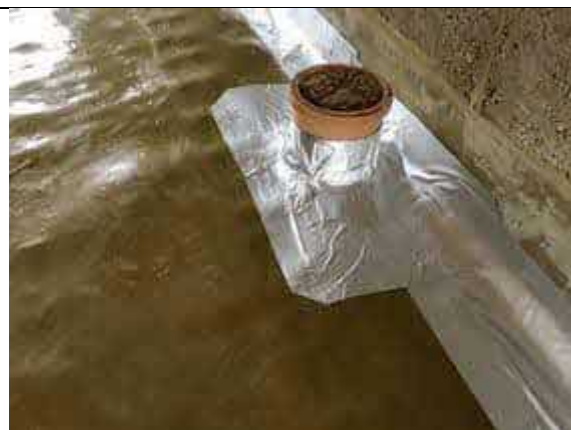
Plot 28 typical pipe penetration seal using SAGM.
