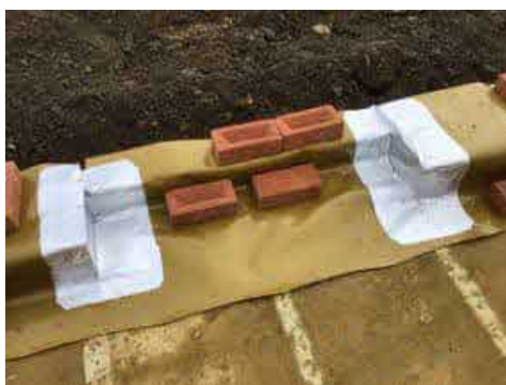
Plot 7 typical door seal using SAGM.
