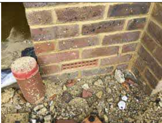
Plot 76 air brick in place at the time of our inspection.
