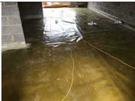
Plot 6 overview of installed membrane.
