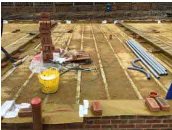
Plot 6 overview of installed membrane.
