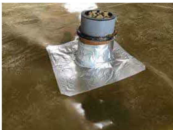
Typical pipe penetration seal using SAGM.
