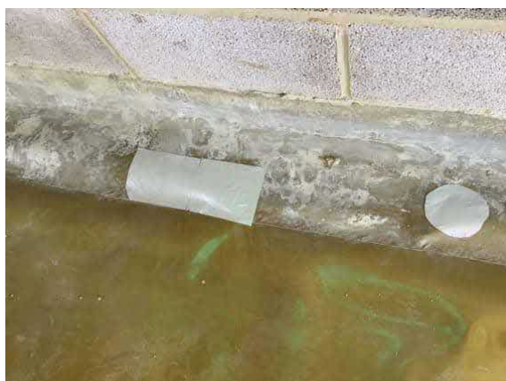
Plot 4 patch repair using SAGM.
