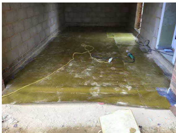
Overview of installed membrane in garage plot 68.
