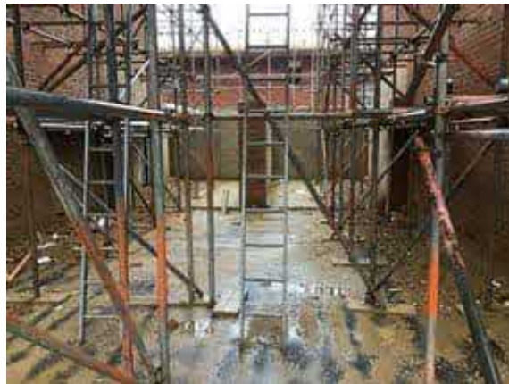
Scaffolding in place in all garages.
