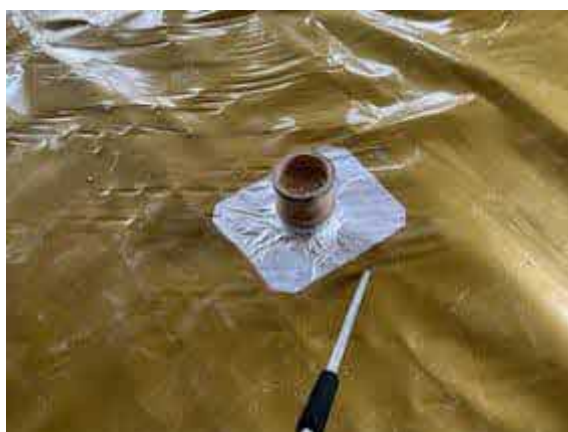
Plot 72. Air lance integrity test upon sealed pipe penetration.
