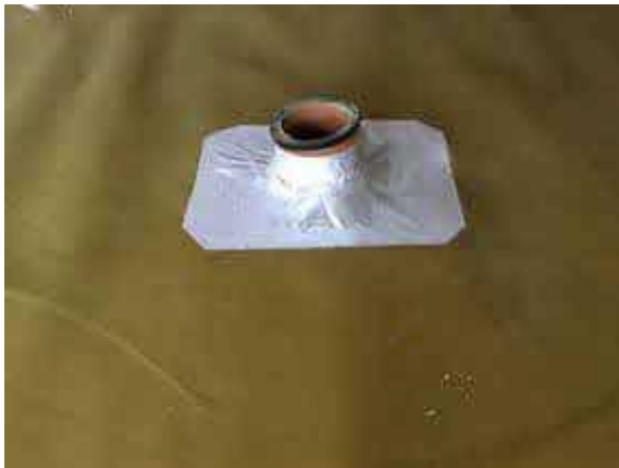
Typical pipe penetration seal to plot 41.
