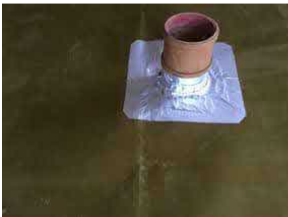
Typical pipe penetration seal using SAGM to plot 36.
