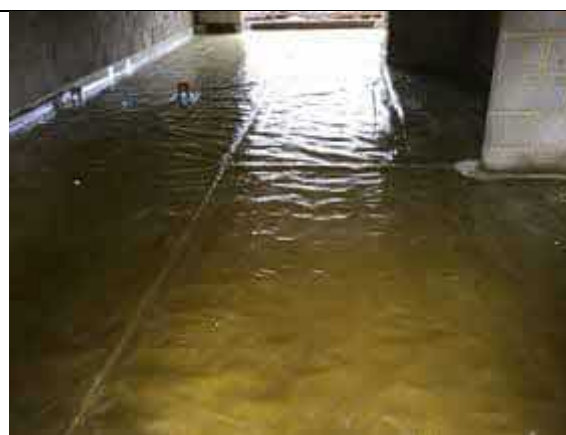
Overview of installed membrane to plot 28.
