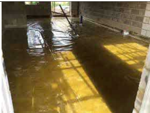
Plot 7 overview of installed membrane.
