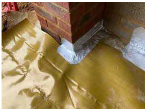
Plot 35 garage. Corner detailing sealed using SAGM.
