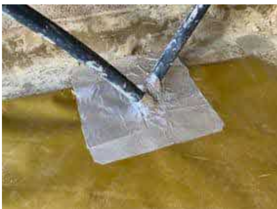
Plot 29 - Pipe penetration's sealed using SAGM.
