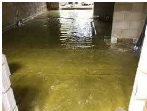
Overview of installed membrane to plot 48.
