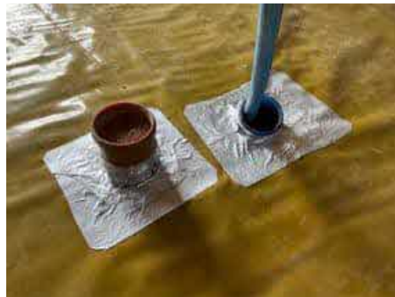
Plot 30 - Typical pipe penetration's sealed using SAGM.
