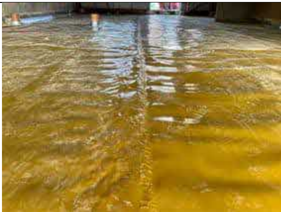
Plot 29 - Successfully hand welded membrane lap joint.
