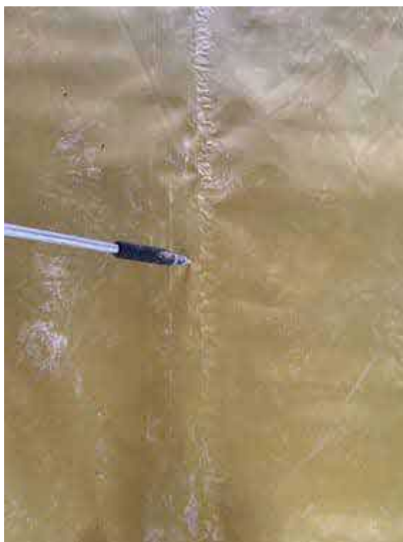
Plot 43 air lancing all hand welded membrane laps.
