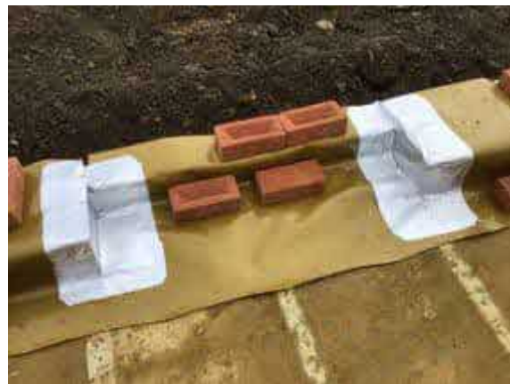
Plot 7 typical door seal using SAGM.
