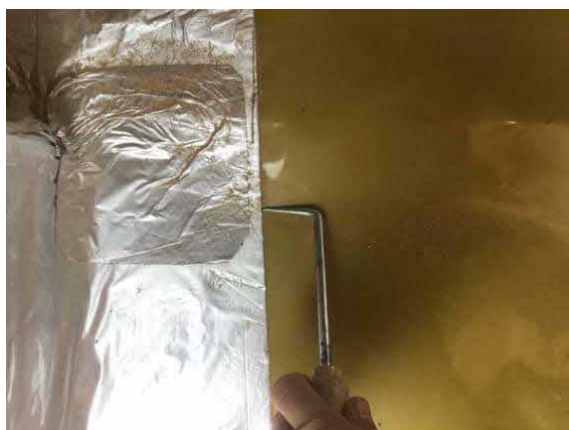
Pick testing all SAGM detailing.
