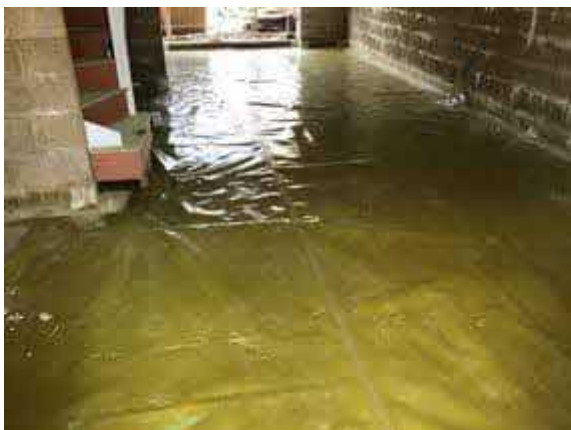
Overview of installed membrane to plot 49.
