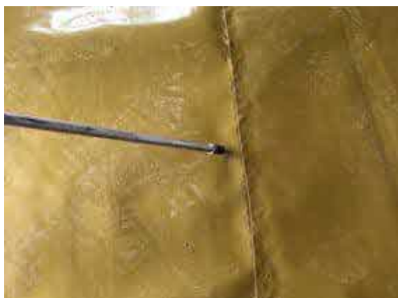
Air lancing all welded membrane laps.
