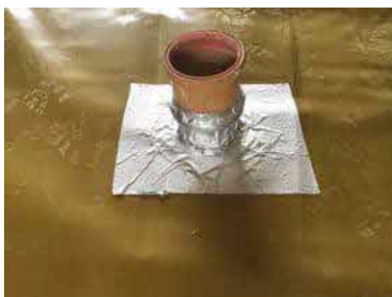
Plot 6 typical pipe penetration seal using SAGM.
