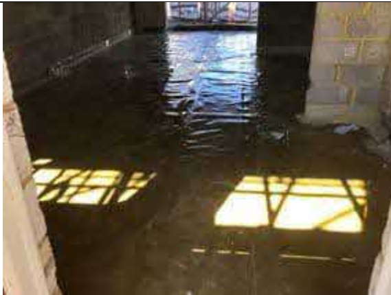
Plot 5 overview of installed membrane.
