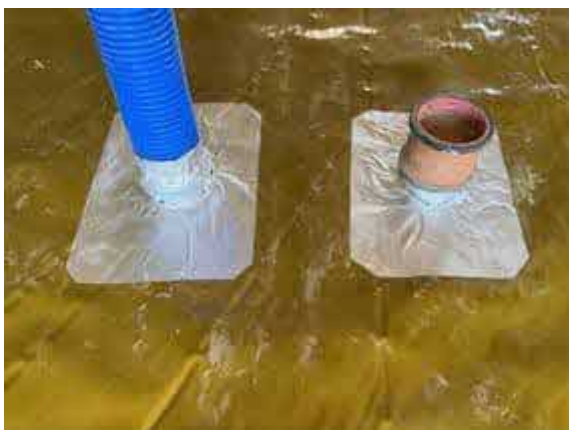
Plot 70. Typical pipe penetration's sealed using SAGM.
