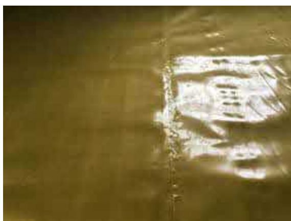
Hand welded membrane lap.
