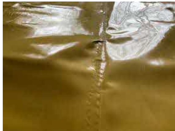
Plot 70. Overview of a hand welded membrane lap joint.
