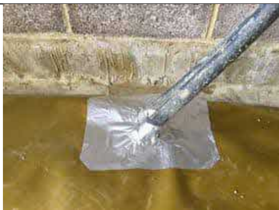
Pipe details within Plot 11 sealed with SAGM.
