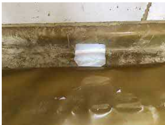
Plot 7 patch repair using SAGM.
