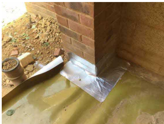
Sealed front of garage using SAGM.
