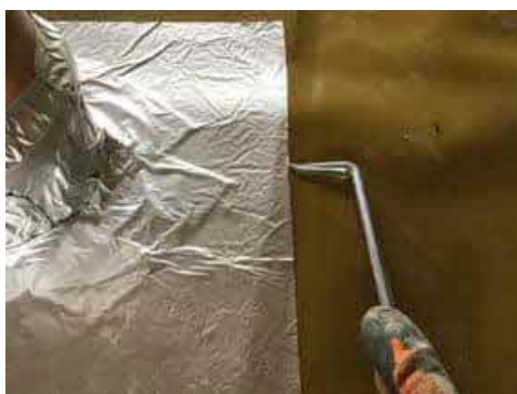
Plot 6 pick testing all SAGM detailing.
