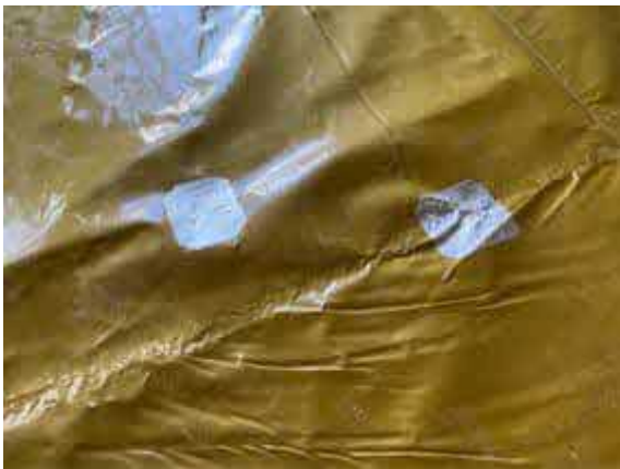
Plot 30 - Patch repairs using SAGM.
