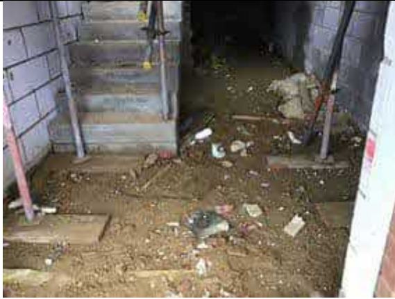
Incomplete stair lobby.
