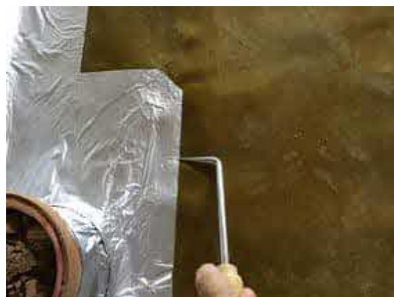
Plot 28 pick testing all SAGM detailing.
