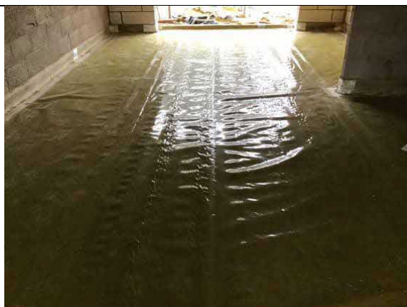
Hand welded membrane lap in plot 51.
