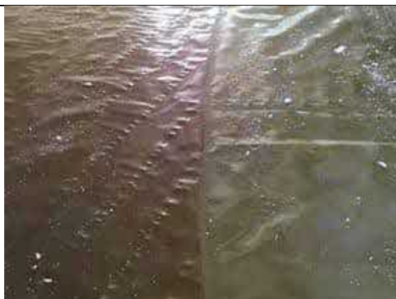
Hand welded membrane lap to plot 65.
