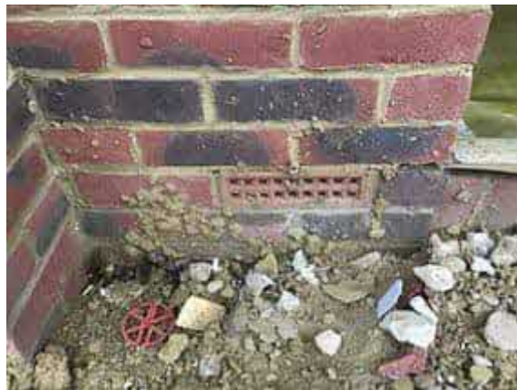
Air brick in place to plot 41.
