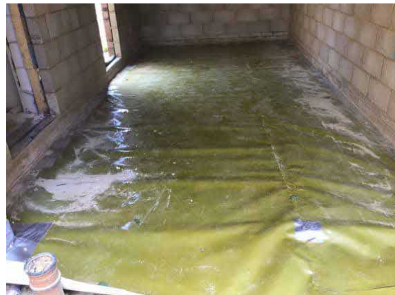
Overview of installed membrane to the garage, as an infill to plot 72.
