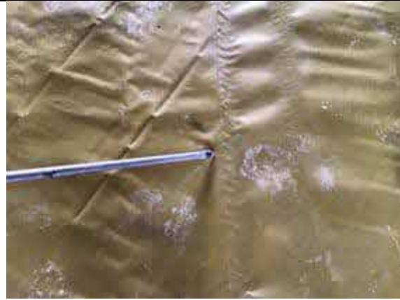
Plot 34 air lancing all welded membrane laps.
