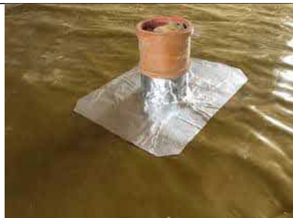
Plot 33 typical pipe penetration seal using SAGM.
