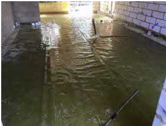
Overview of installed membrane to plot 67.
