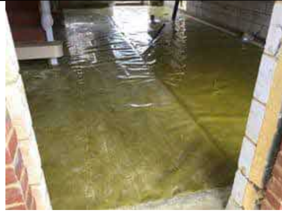
Overview of installed membrane to plot 50.
