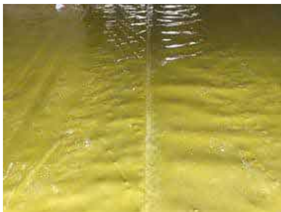
Hand welded membrane lap to plot 48.
