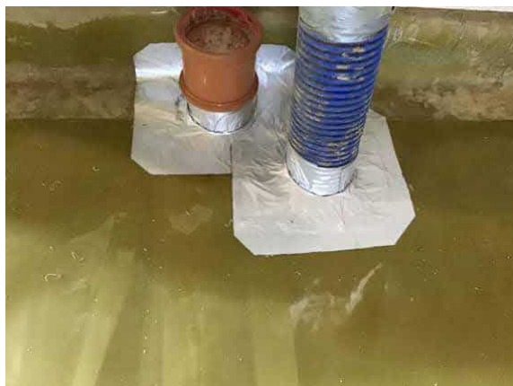
Sealed double pipe penetration using SAGM to plot 53.
