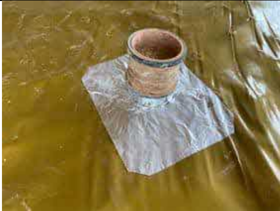
Plot 72. Typical pipe penetration sealed with SAGM.
