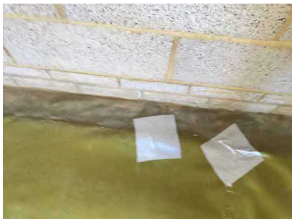
Patch repairs using SAGM to damaged membrane.
