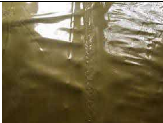
Hand welded membrane lap to plot 64.
