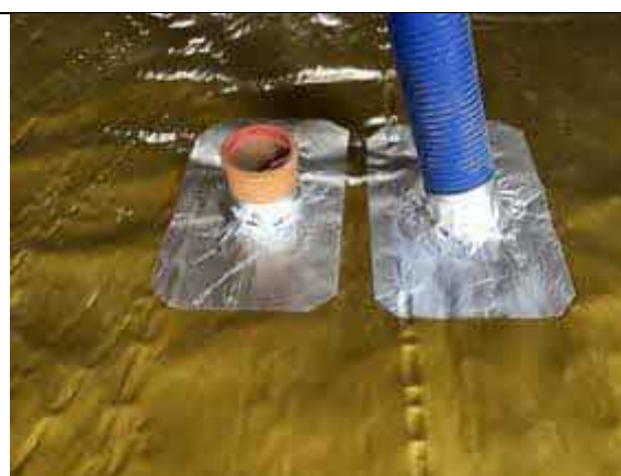
Plot 27 typical double pipe penetration seal using SAGM.
