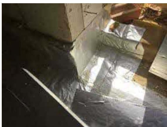
Re sealed door threshold detail using SAGM to plot 65.
