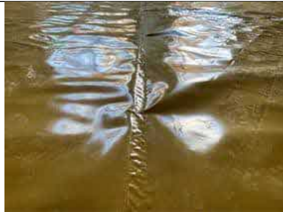
Plot 30 - Hand welded membrane lap joint.
