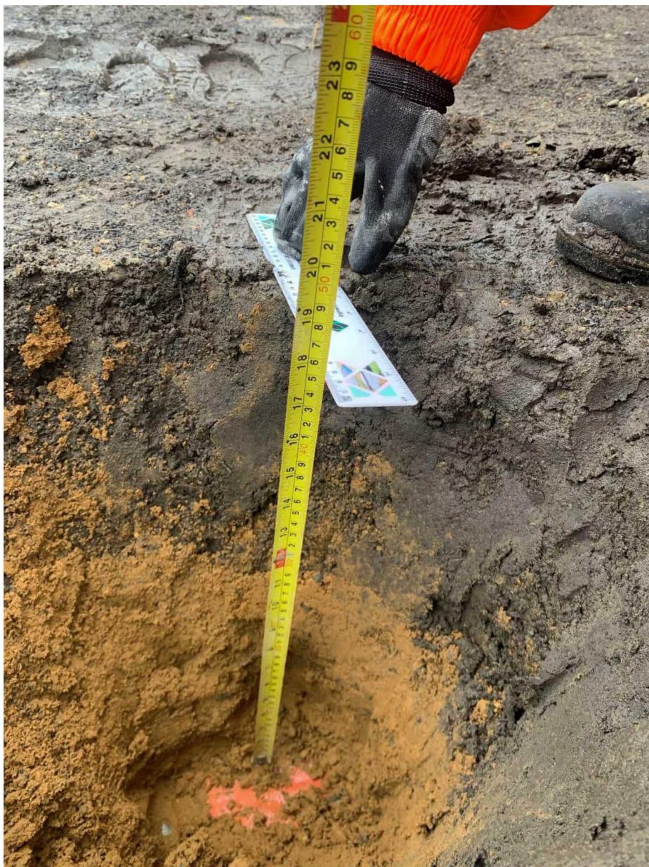
Photo 1: Plot 12 Front Garden showing topsoil, subsoil and geotextile.
