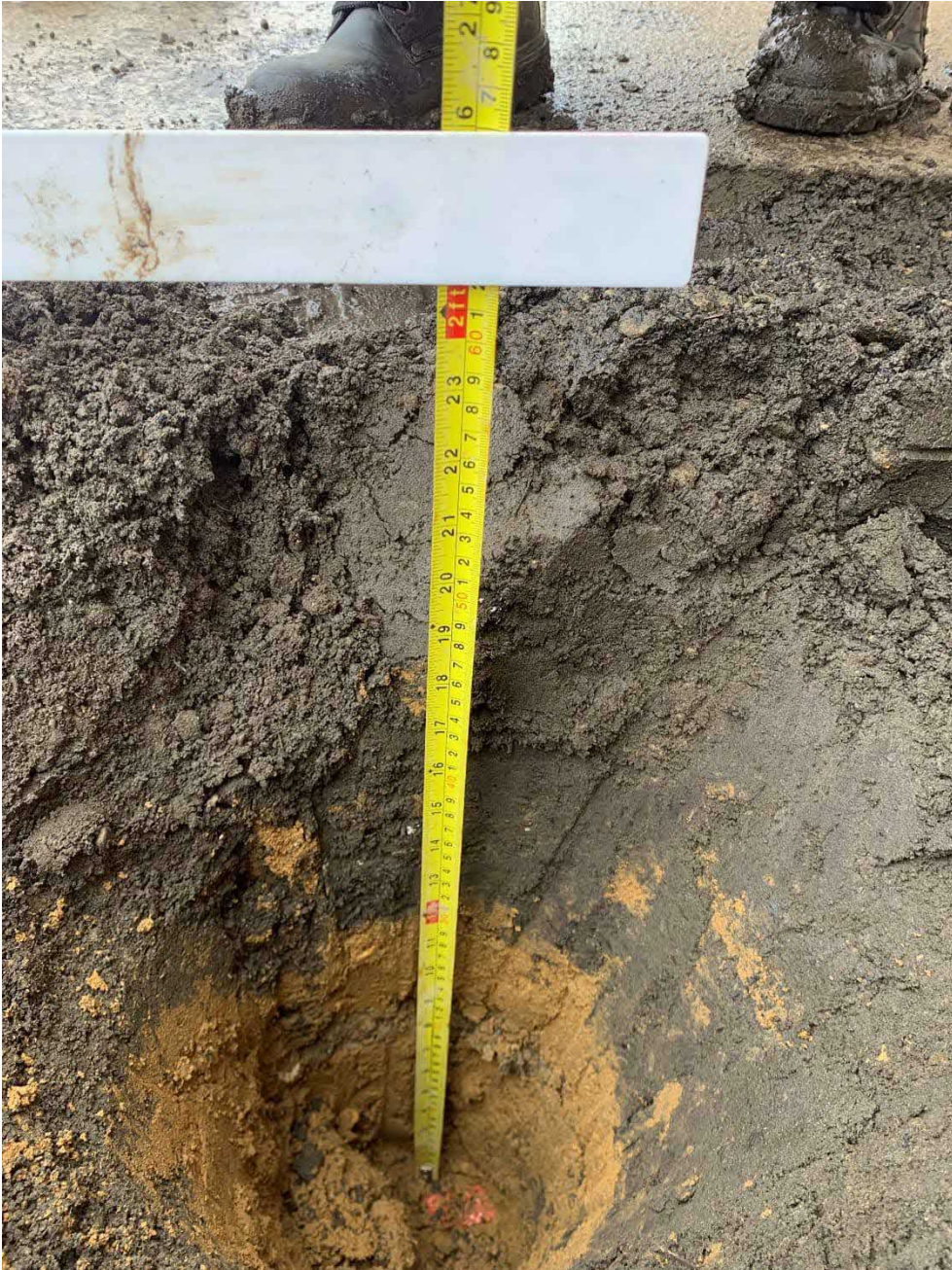
Photo 3: Plot 34 Front garden showing topsoil, subsoil and geotextile.
