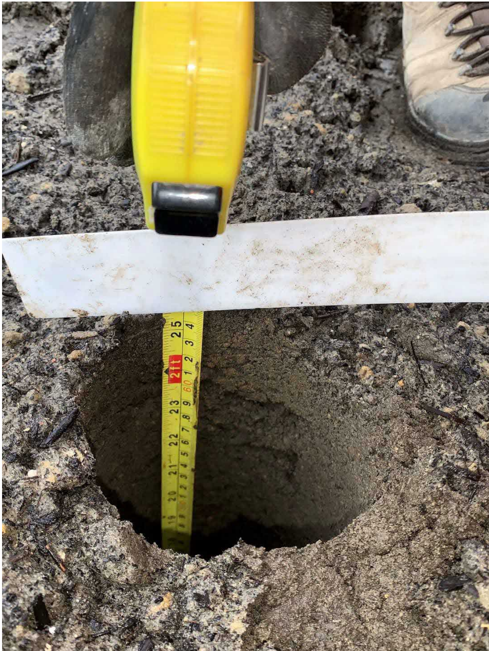
Photo 5a: Plot 33 rear garden showing depth to geotextile.
