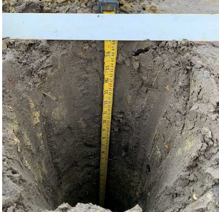
Photo 4: Plot 53 rear garden showing depth to geotextile.
