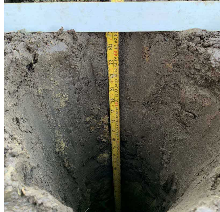
Photo 3: Plot 52 rear garden showing depth to geotextile.
