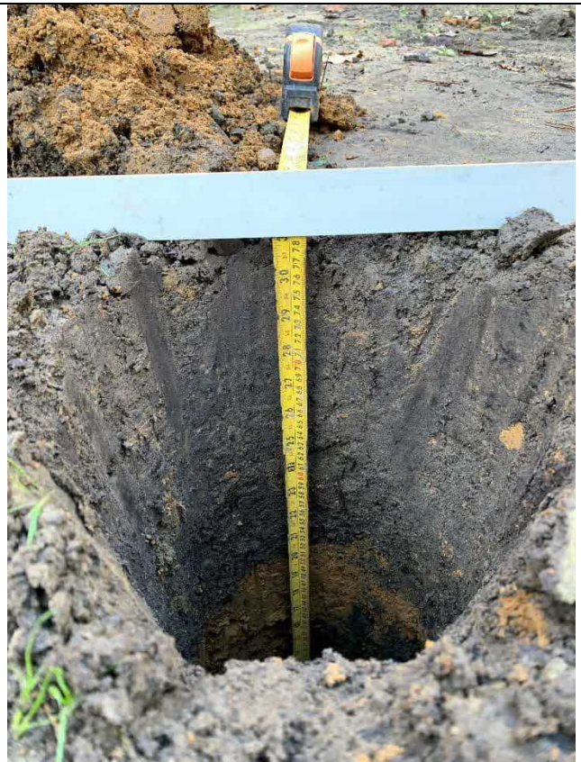
Photo 10: Plot 66 rear garden showing depth to geotextile.
