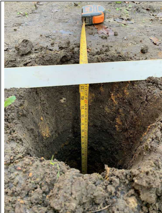
Photo 9: Plot 64 rear garden showing depth to geotextile.
