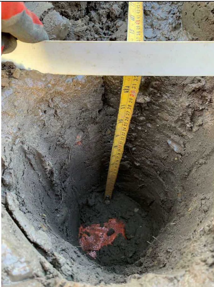
Photo 5: Block G landscaping area showing depth to geotextile.
