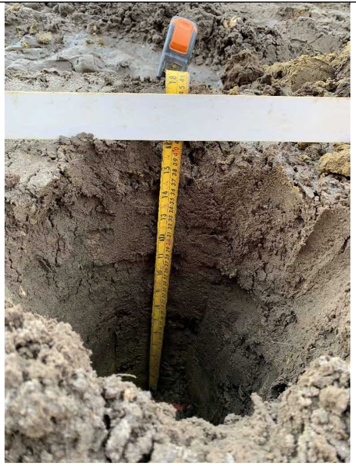
Photo 6: Block H landscaping area showing depth to geotextile.
