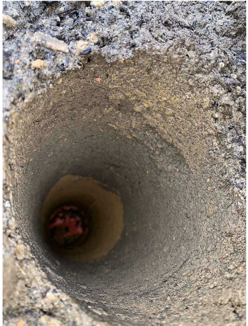
Photo 5b: Plot 33 rear garden showing the topsoil, subsoil and geotextile.
