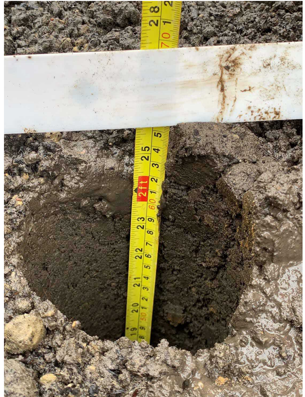
Photo 4: Plot 35 Front garden showing the depth of pit. Geotextile visible on site.
