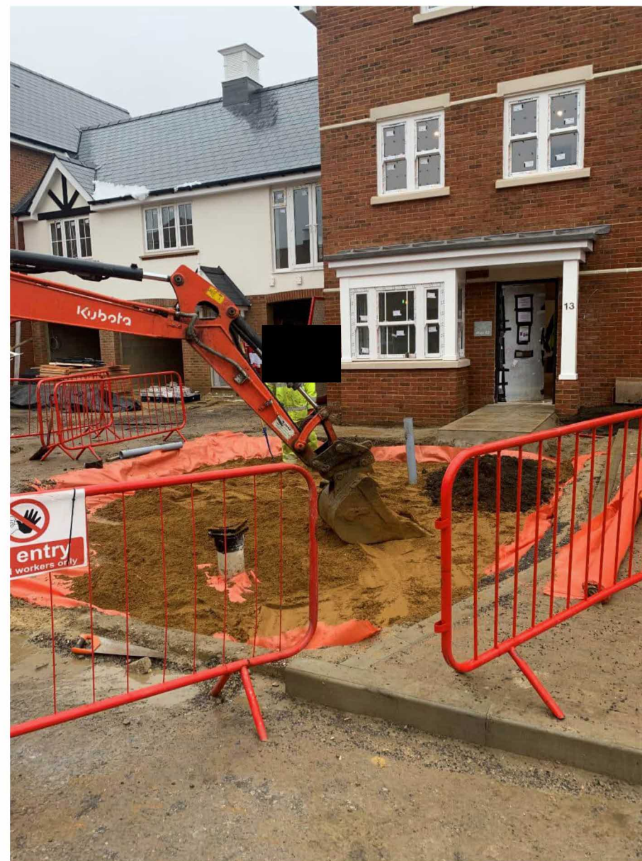
Photo 2: Plot 32 Front garden showing subsoil deposition over orange geotextile.
