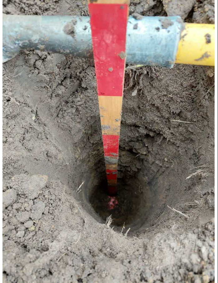
1a Base of Inspection Pit
