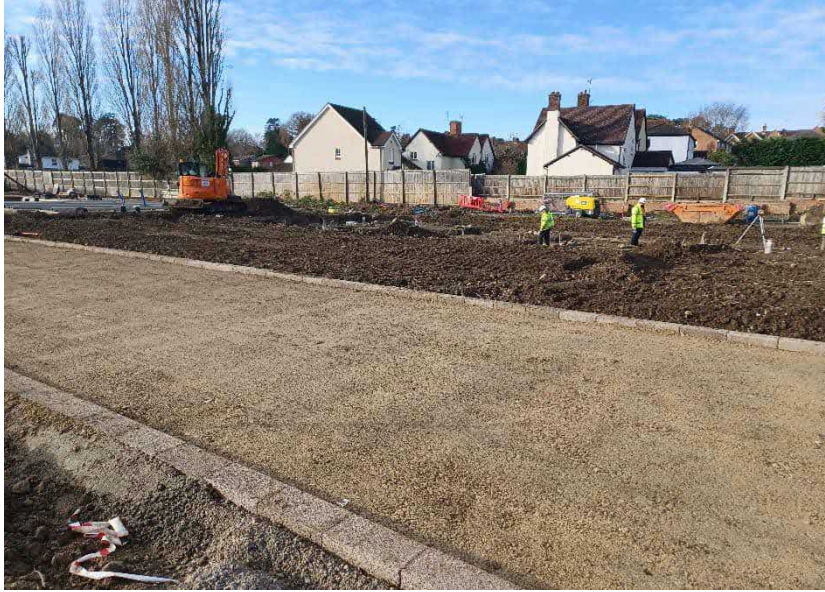
09 December 2021 On Going Infrastructure Works
