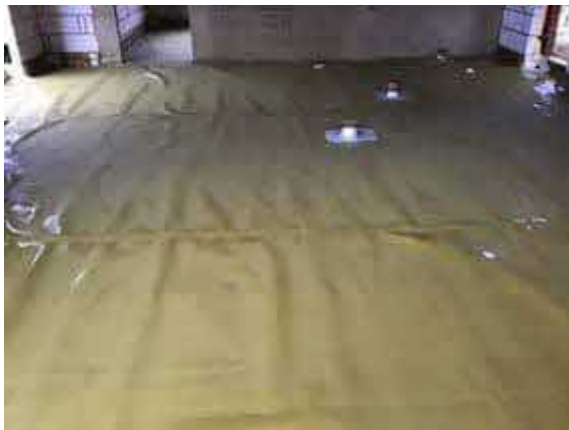
Overview of installed membrane to plot 41.
