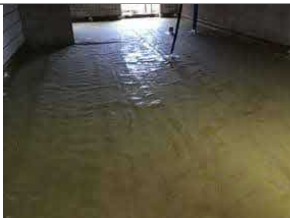
Overview of installed membrane to plot 37.
