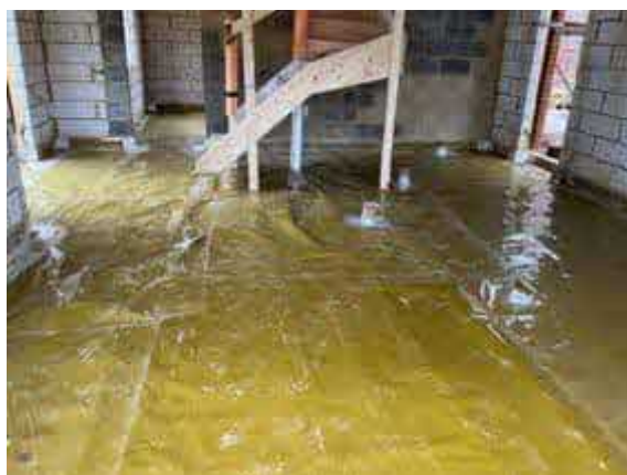
Overview of Visqueen HC Blok infill installation to Plot 72.
