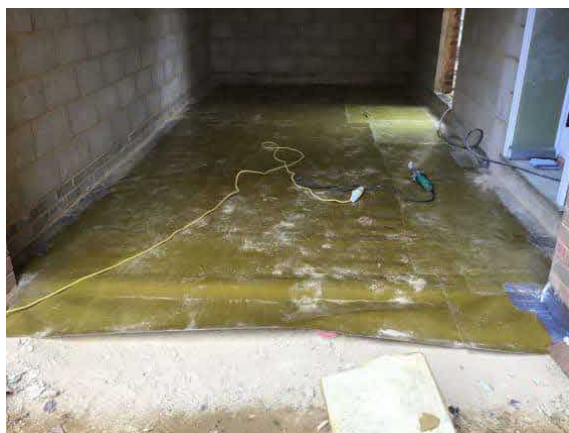
Overview of installed membrane in garage plot 68.
