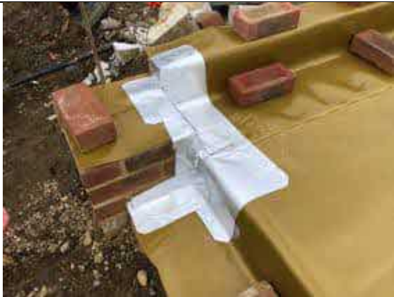
Plot 4 seal using SAGM to the front of the garage.
