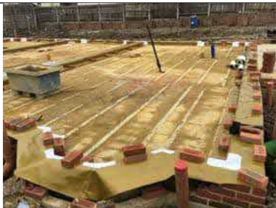
Plot 7 overview of installed membrane.
