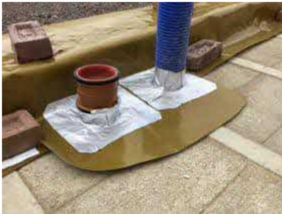
Plot 74 typical double pipe penetration seal using SAGM.
