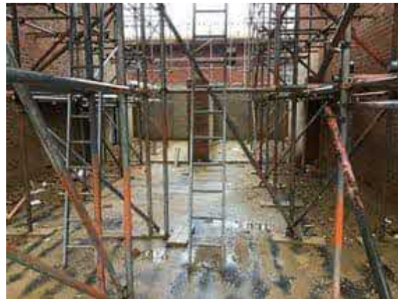
Scaffolding in place in all garages.
