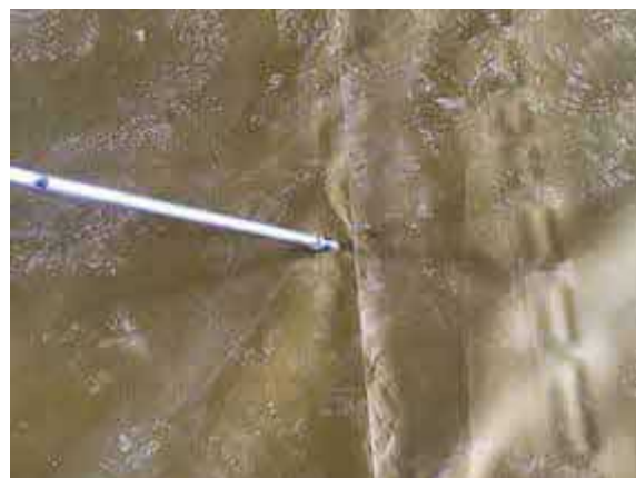
Plot 7 air lancing all welded membrane laps.
