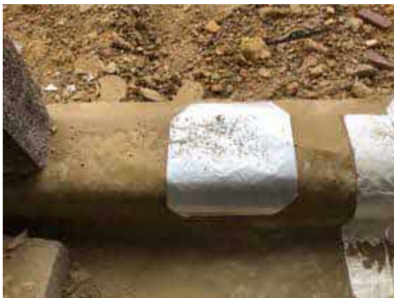
Patch repair using SAGM to damaged perimeter membrane.
