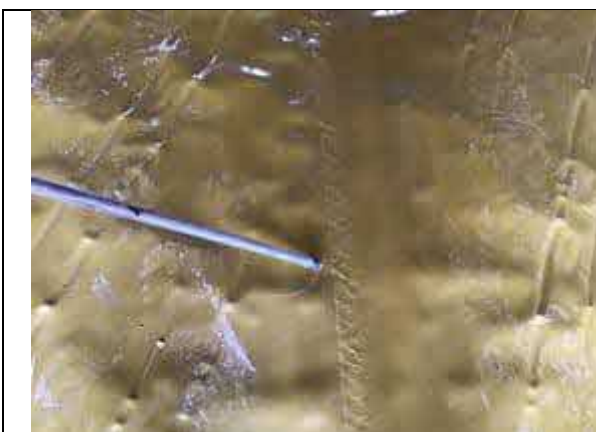
Plot 27 air lancing all weld laps.
