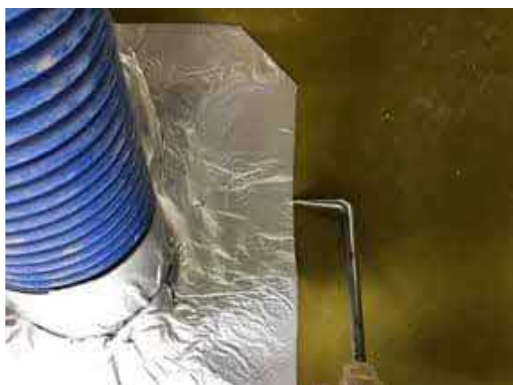
Pick testing all SAGM detailing in plot 50.
