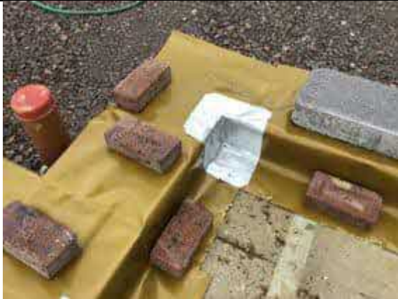
Plot 73 typical corner seal using SAGM.
