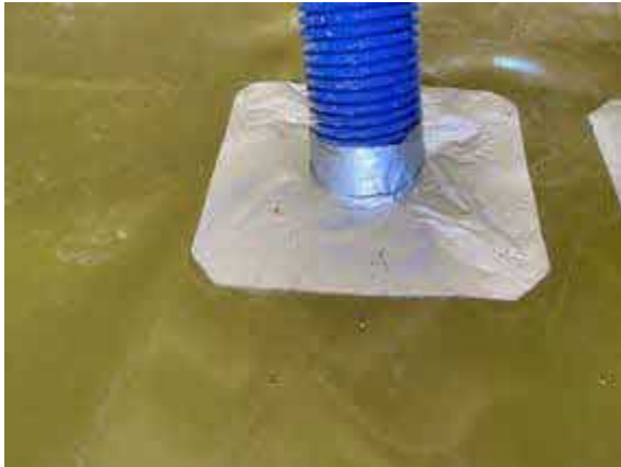
Plot 45 typical pipe penetration seal using SAGM.
