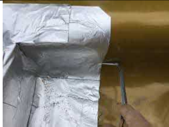
Plot 74 pick testing all SAGM detailing.
