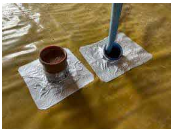
Plot 30 - Typical pipe penetration's sealed using SAGM.
