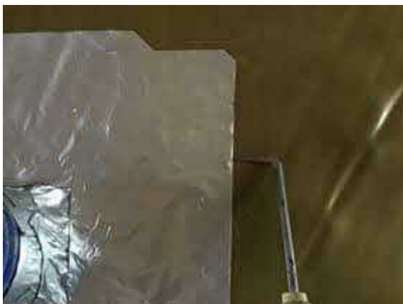
Pick testing all SAGM detailing to plot 64.
