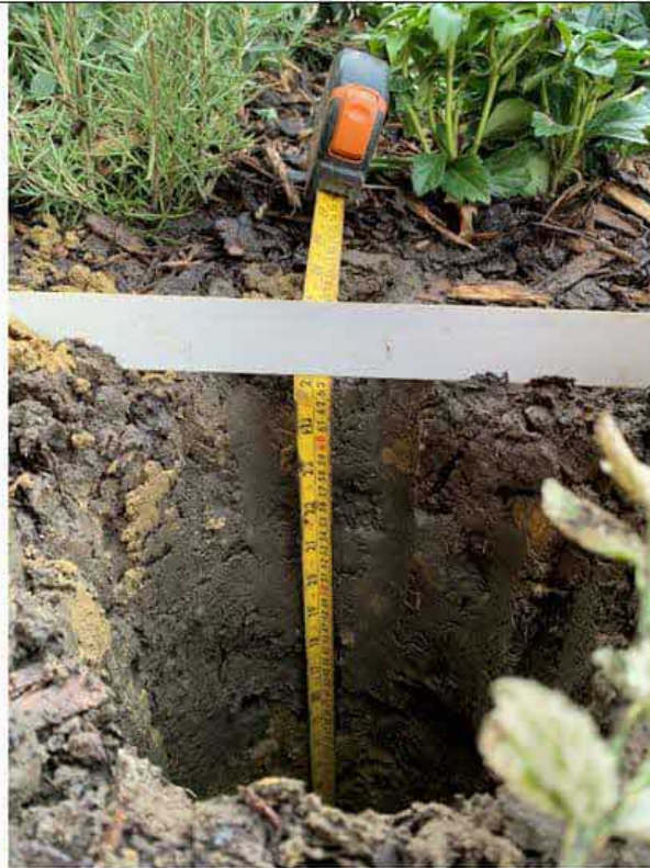
Photo : Plot 67 front garden showing depth to geotextile.
