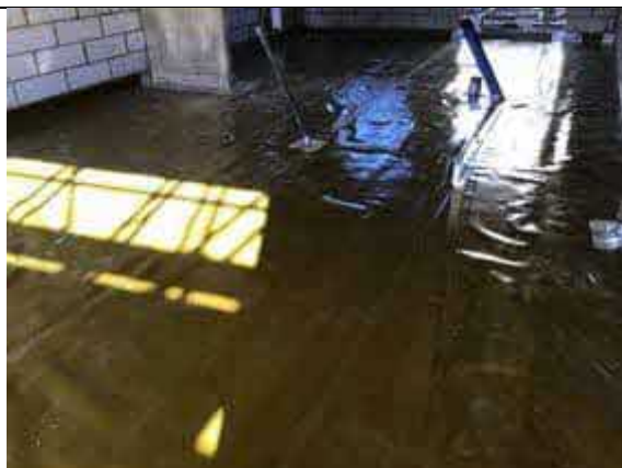
Plot 2 overview of installed membrane.
