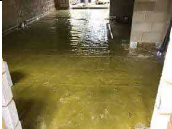
Overview of installed membrane to plot 48.
