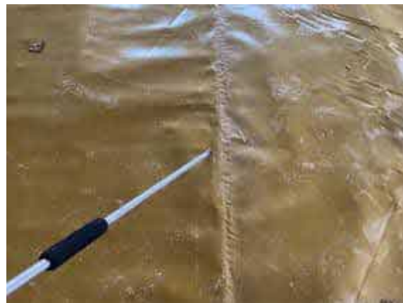
Plot 70. Air lance integrity testing along hand welded lap joint.
