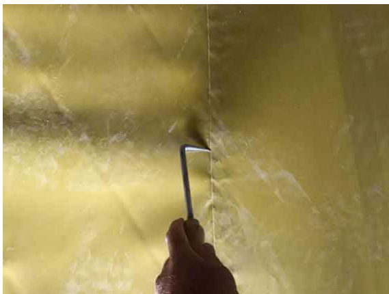
Pick testing all hand welded membrane laps.
