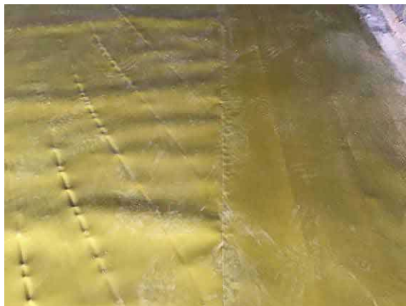
Typical hand welded membrane lap.
