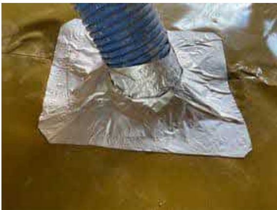
Plot 40. Typical pipe penetration sealed using SAGM.
