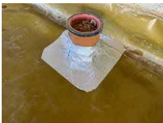
Plot 73. Typical pipe penetration sealed using SAGM.
