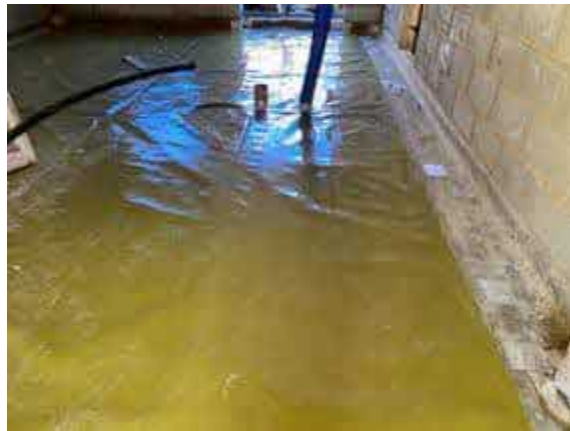
Plot 45 overview of installed membrane.
