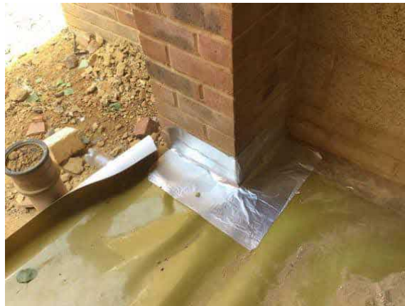
Sealed front of garage using SAGM.
