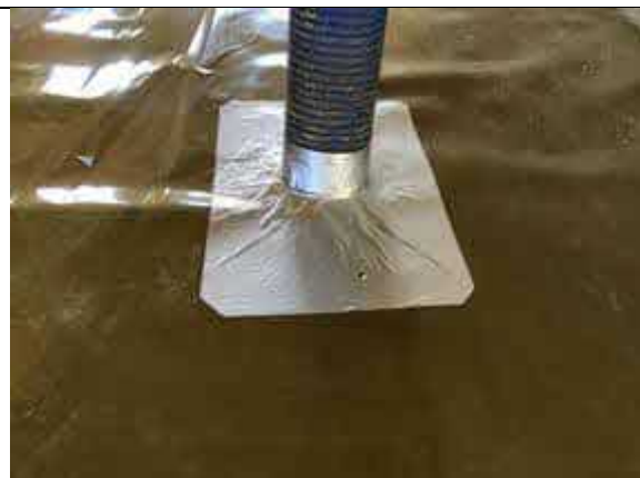
Plot 4 typical pipe penetration seal using SAGM.
