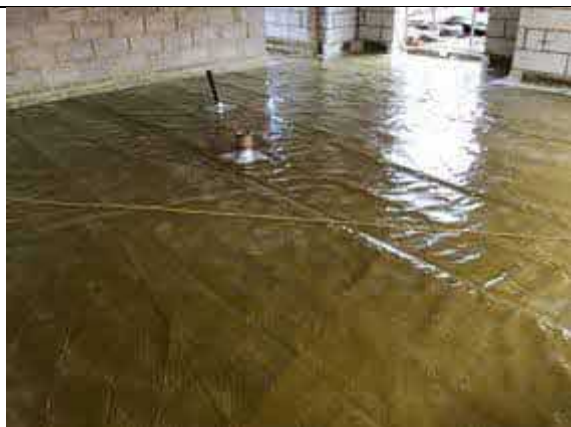
Plot 75 overview of installed membrane.
