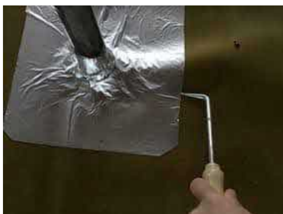
Pick testing all SAGM detailing to plot 38.
