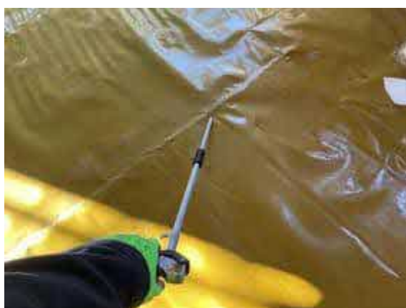
Plot 73. Air lance integrity test conducted upon all hand welded membrane lap joints.
