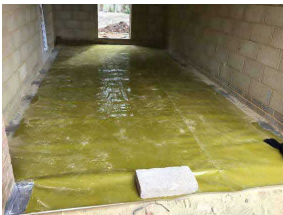
Overview of installed membrane in garage plot 67.
