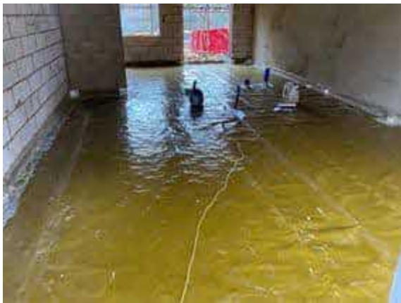
Overview of Visqueen HC Blok infill installation to Plot 70.
