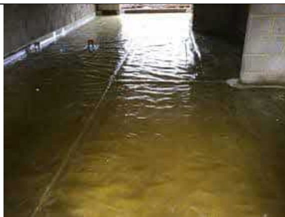
Overview of installed membrane to plot 28.
