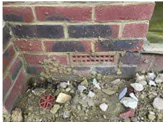
Air brick in place to plot 41.
