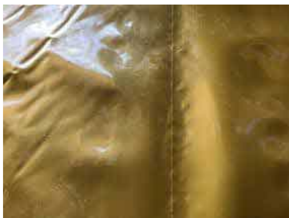
Plot 4 hand welded membrane lap.
