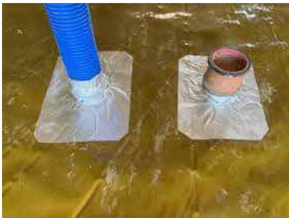
Plot 70. Typical pipe penetration's sealed using SAGM.
