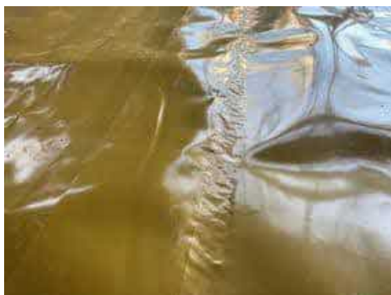
Plot 74. Hand welded membrane lap joint.
