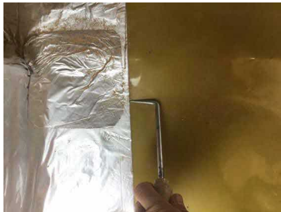
Pick testing all SAGM detailing.
