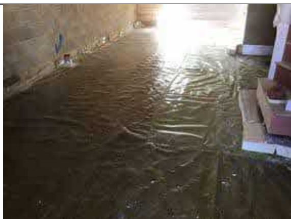
Overview of installed membrane to plot 65.
