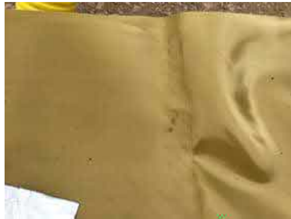
Plot 74 hand welded membrane laps over the cavity wall.
