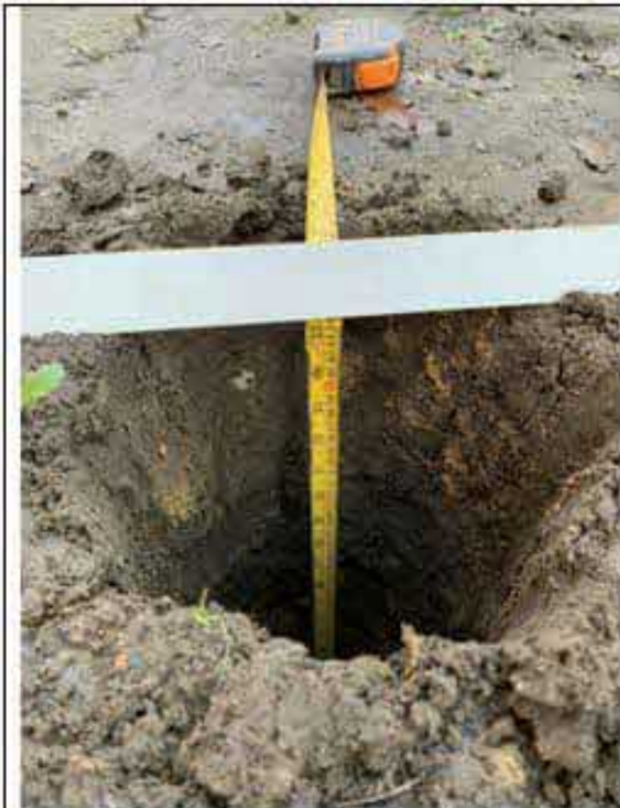
Photo : Plot 64 rear garden showing depth to geotextile.
