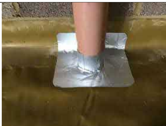
Typical pipe penetration seal using SAGM.
