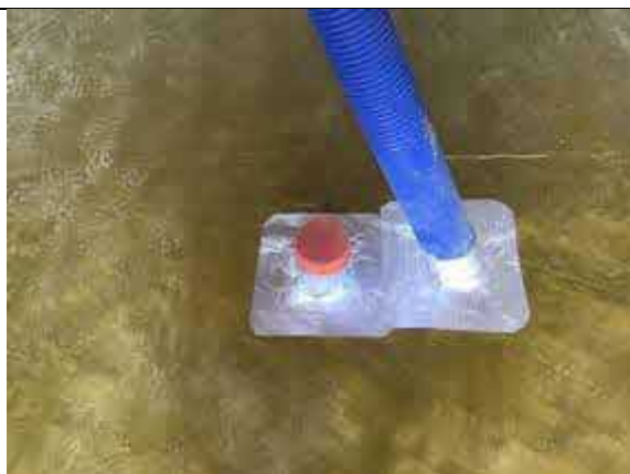
Plot 9 pipe penetrations sealed using SAGM
