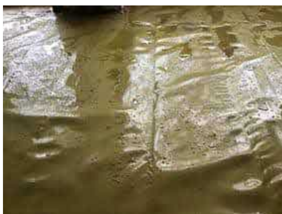
Hand welded membrane lap in plot 38.
