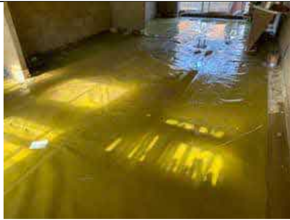
Plot 44 overview of installed membrane.
