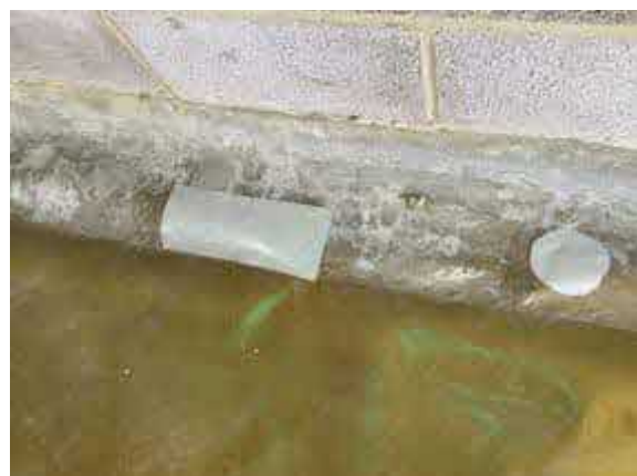
Plot 4 patch repair using SAGM.
