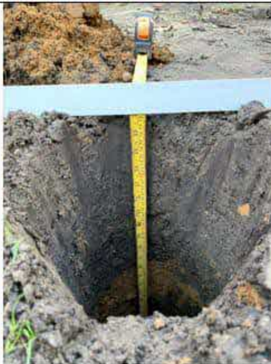
Photo : Plot 66 rear garden showing depth to geotextile.
