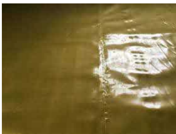
Hand welded membrane lap.
