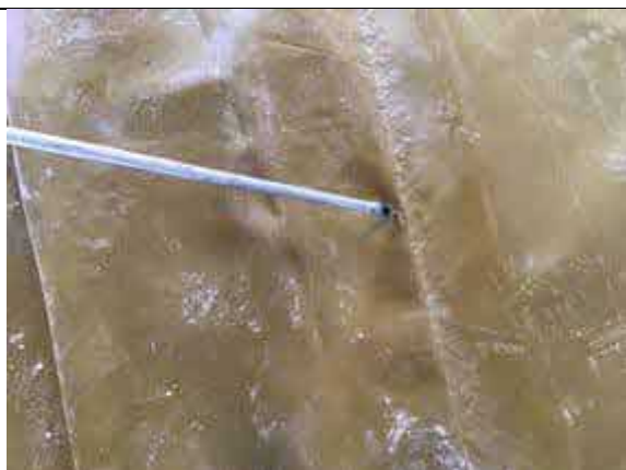
Plot 2 air lancing all weld laps and SAGM detailing.
