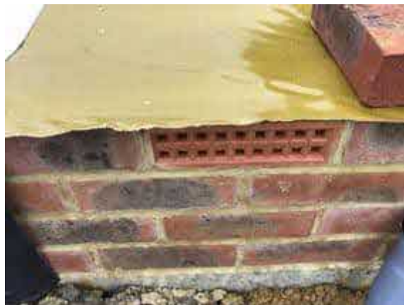
Plot 6 air brick in place.
