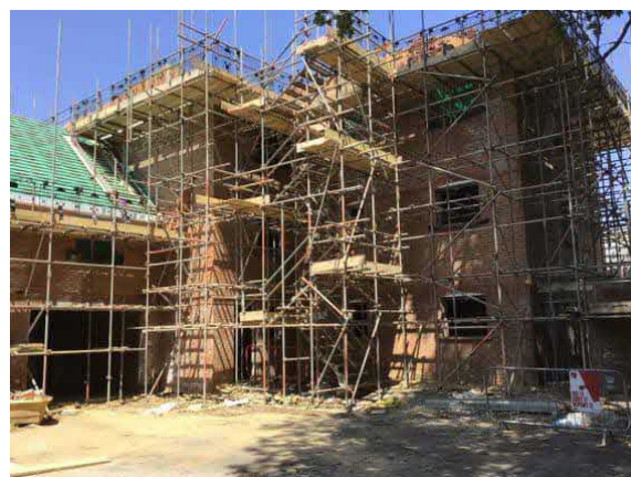
Overview of Apartment Block H. Plots 54-62.
