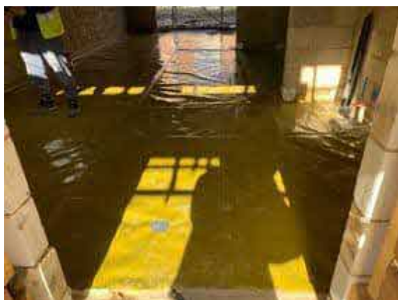
Plot 43 overview of installed membrane.
