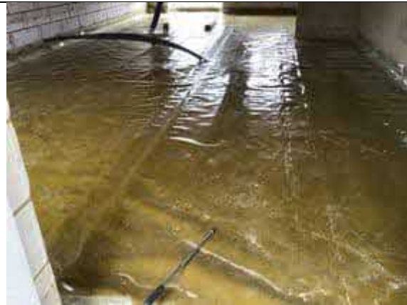
Plot 32 overview of installed Visqueen HC Blok Gas membrane.
