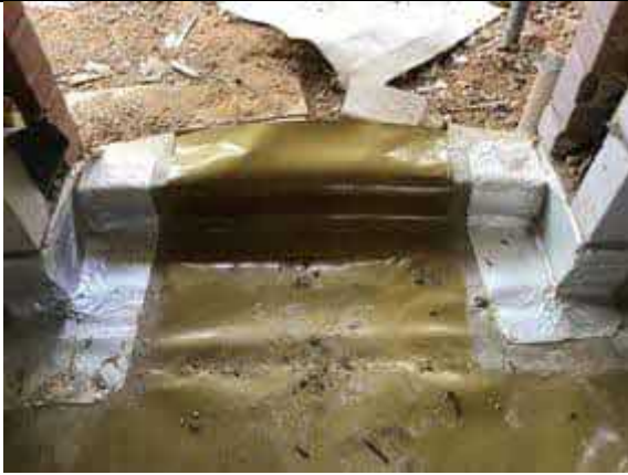
Sealed door threshold using SAGM.
