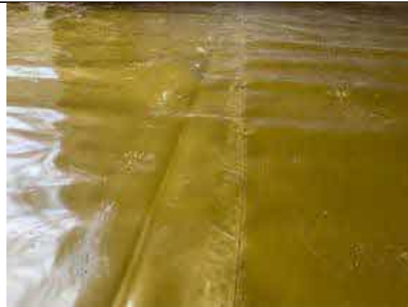
Plot 72. Overview of a hand welded membrane lap joint.
