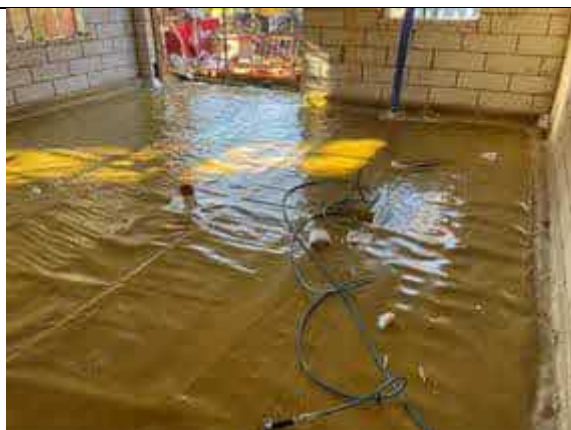
Plot 73. Visqueen HC Blok infill installation.
