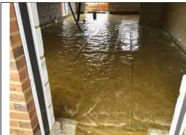
Overview of installed membrane to plot 27.
