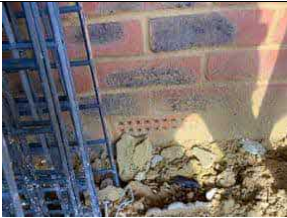
Plot 44 air brick in place at the time of our inspection.
