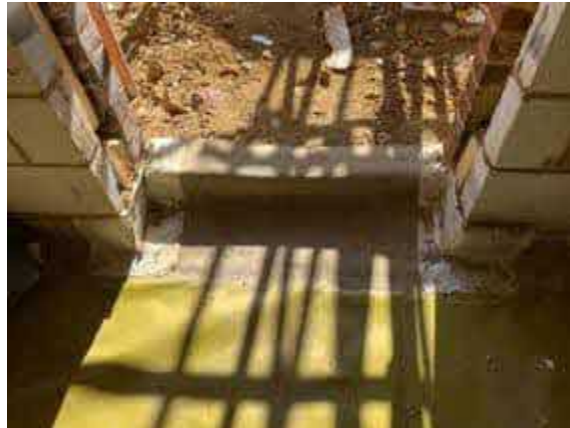
Plot 45 sealed door threshold detail using SAGM.
