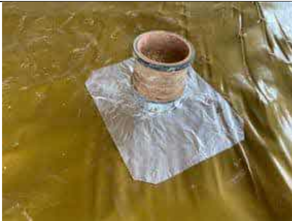
Plot 72. Typical pipe penetration sealed with SAGM.
