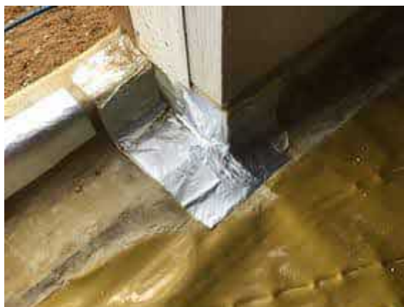
Sealed corner detail using SAGM.
