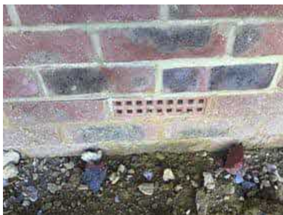
Air brick in place at the time of our inspection.
