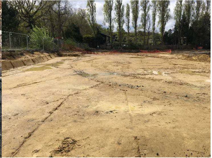
Excavation area in south-east corner, onto natural ground.
