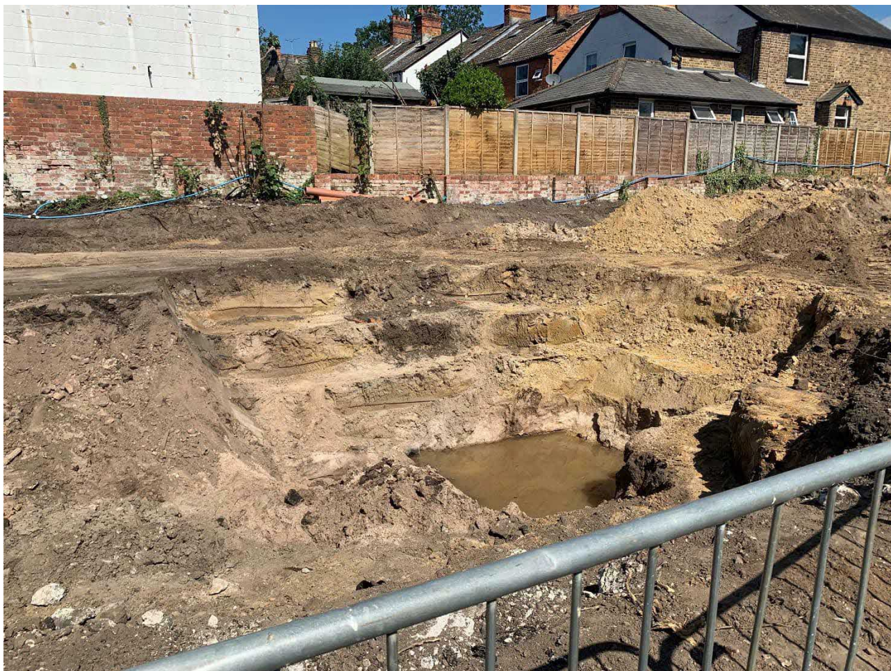
Excavation in north-west of the site
