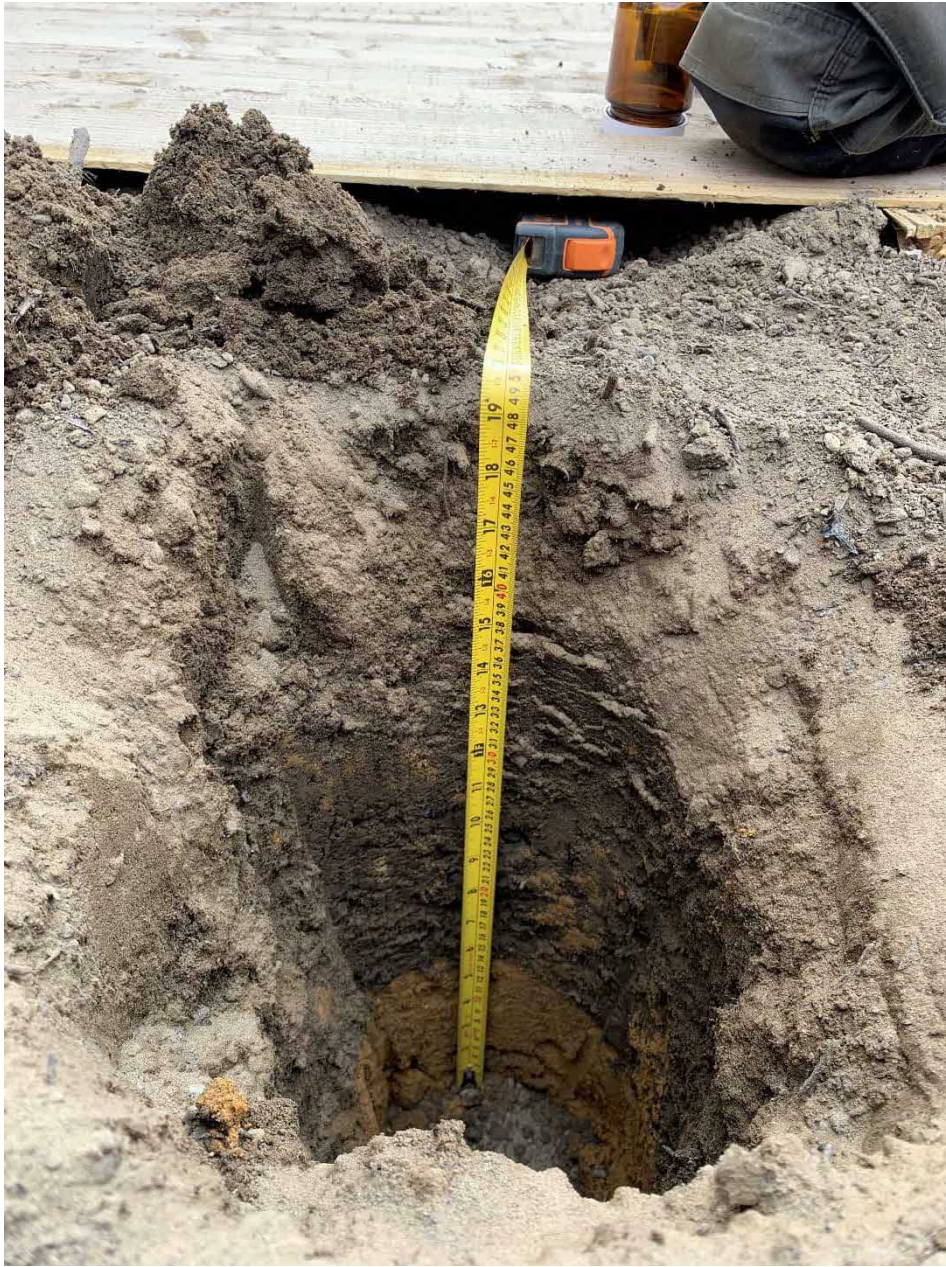
Photo 3: Plot 39 Front garden showing topsoil, subsoil and geotextile.
