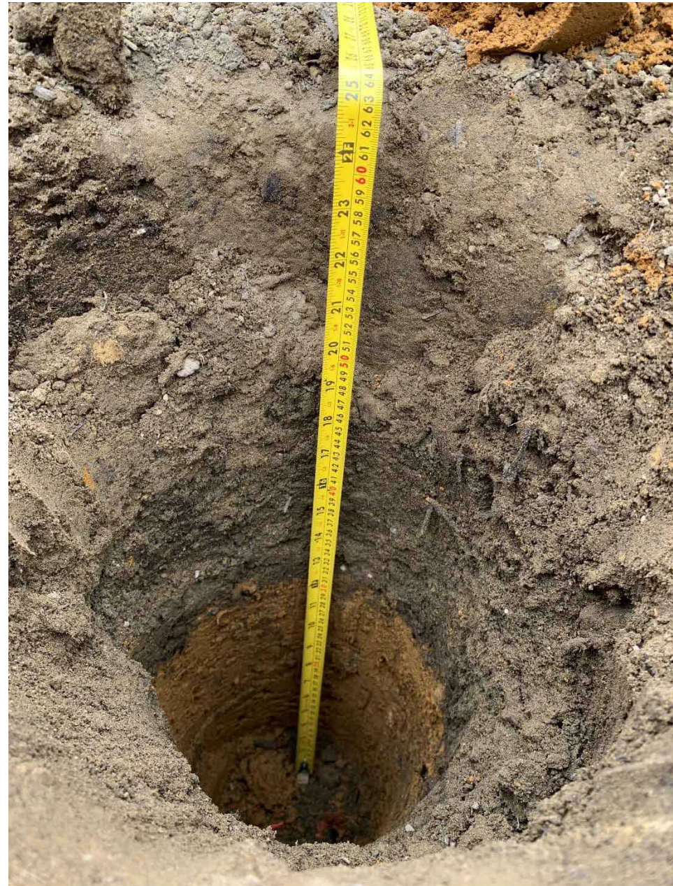
Photo 4: Plot 36 Rear garden showing topsoil, subsoil and geotextile.
