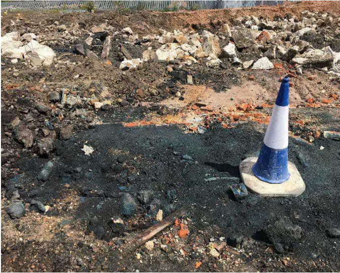
Spent oxide within soils along HV electricity cable route.
