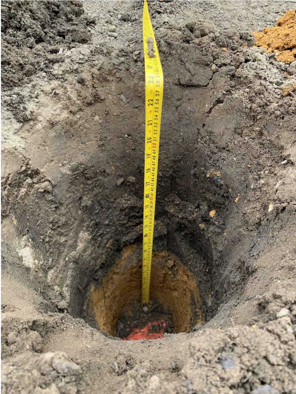
Photo 5: Plot 38 Rear garden showing topsoil, subsoil and geotextile.
