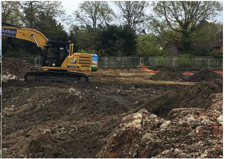
Excavation in central site.
