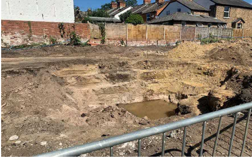
14/06/2021 North-west corner excavations and Post Cottage Demolition
