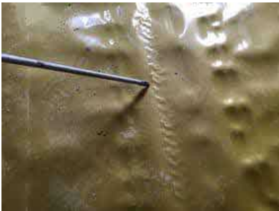
Plot 32 air lancing all welded membrane laps.
