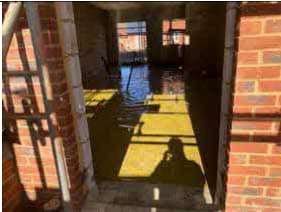
Plot 42 overview of installed membrane.
