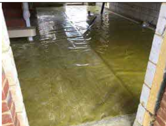
Overview of installed membrane to plot 50.
