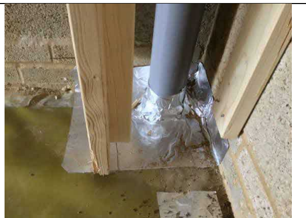
Sealed pipe penetration using SAGM to the rear of the garage plot 45.
