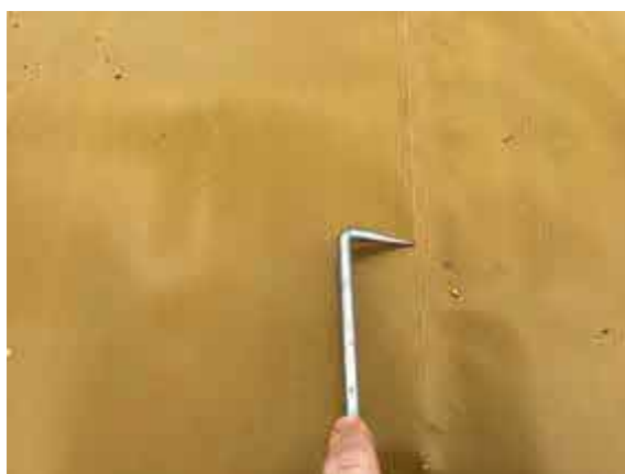
Plot 4 pick testing all weld laps.
