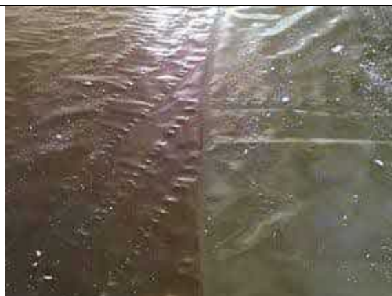
Hand welded membrane lap to plot 65.
