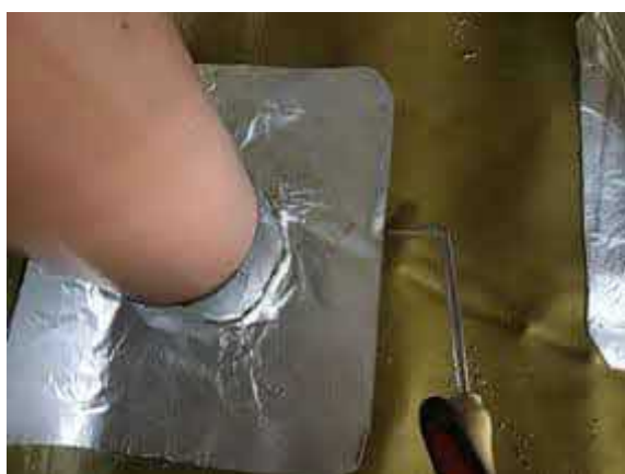
Pick testing all SAGM detailing.
