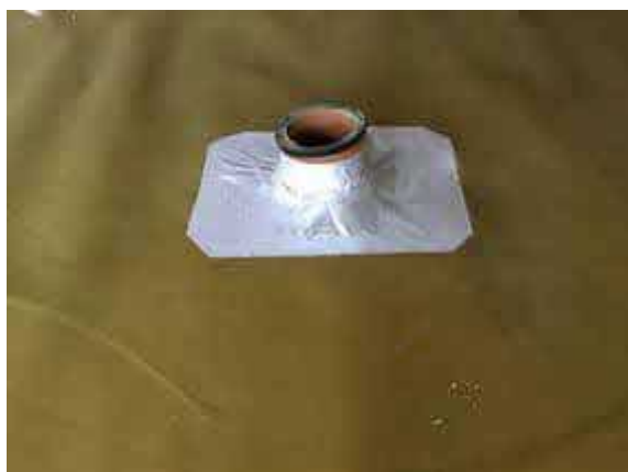
Typical pipe penetration seal to plot 41.
