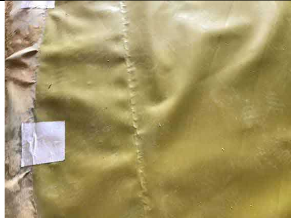
Hand welded membrane lap in garage plot 40.
