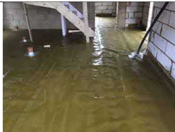
Overview of installed membrane to plot 36.
