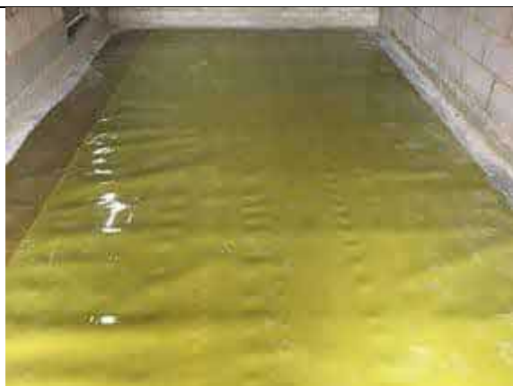
Overview of installed membrane to the garage area in plot 36.
