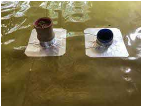
Sealed double pipe penetrations using SAGM to plot 67.
