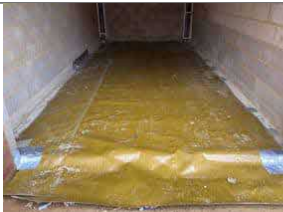
Overview of Visqueen HC Blok infill installation to Plot 30 FOG Unit Garage.
