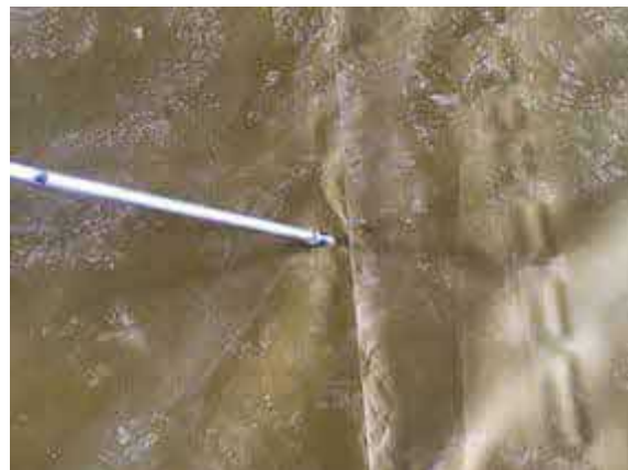
Plot 7 air lancing all welded membrane laps.
