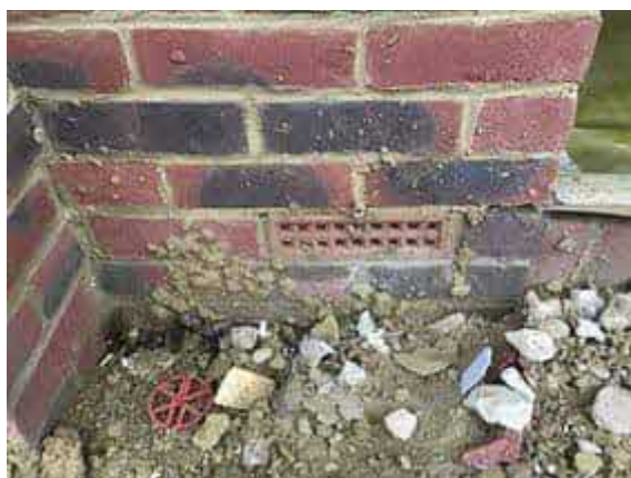
Air brick in place to plot 41.
