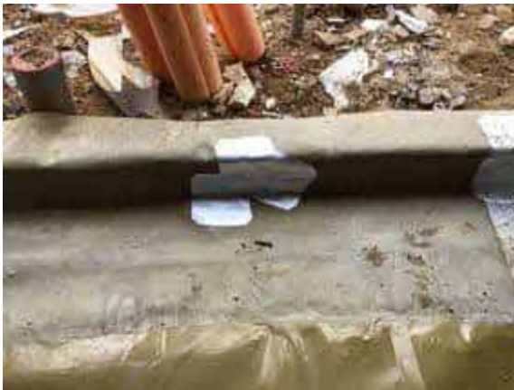
Patch repairs to damaged perimeter membrane using SAGM.
