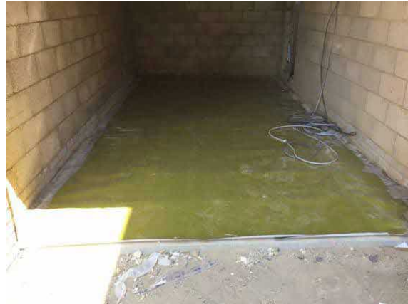
Overview of installed membrane to the garage in plot 41.
