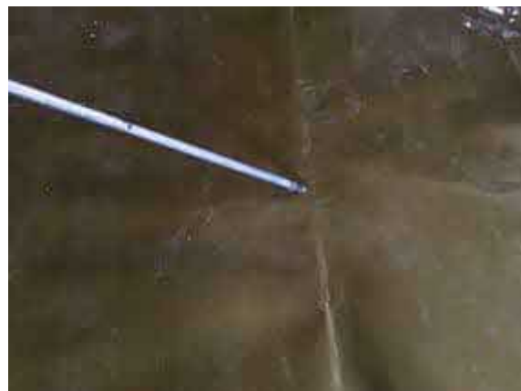
Air lancing all welded membrane laps to plot 37.
