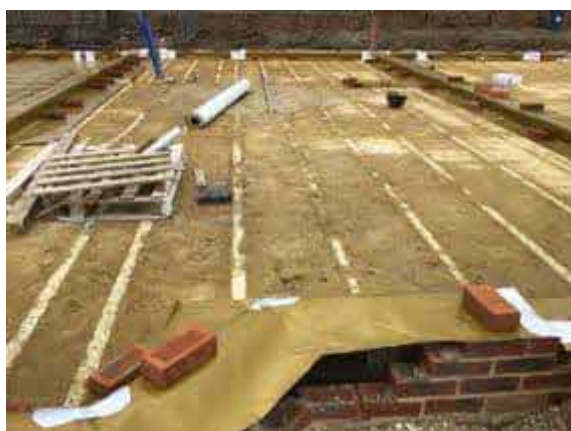
Plot 4 overview of installed membrane to the perimeters and party walls.
