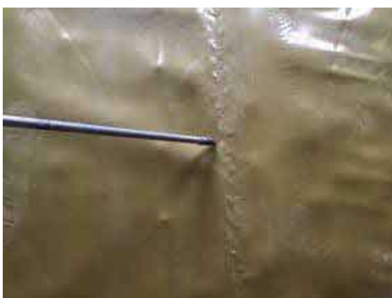
Air lancing all hand welded membrane laps to plot 64.
