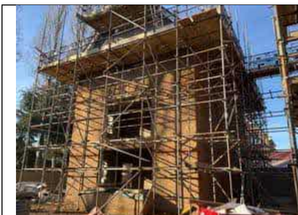
Plot 73 Overview where Visqueen HC Blok was installed.
