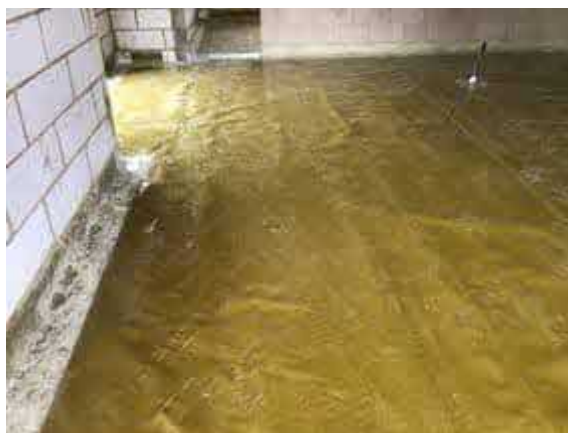
Plot 76 overview of installed membrane.
