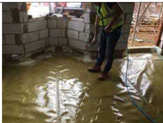
Air lance testing to Plot 10 lap joints.
