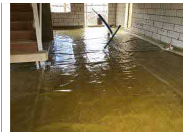
Plot 35 overview of installed Visqueen HC Blok Gas Barrier as an infill.
