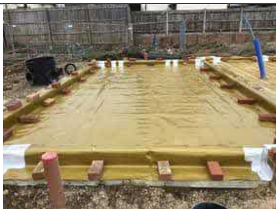
Plot 4 overview of installed membrane to the garage.
