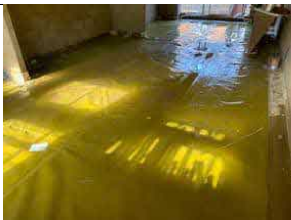
Plot 44 overview of installed membrane.
