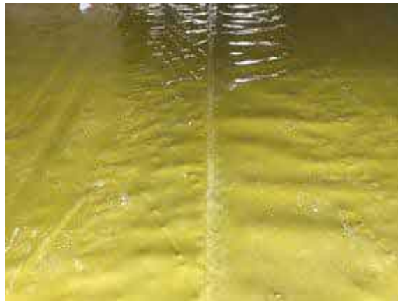
Hand welded membrane lap to plot 48.
