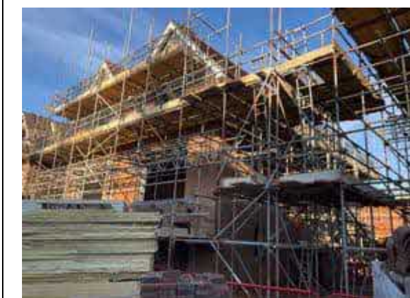
Plot 40 overview of where the installation took place.
