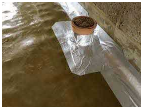
Plot 28 typical pipe penetration seal using SAGM.
