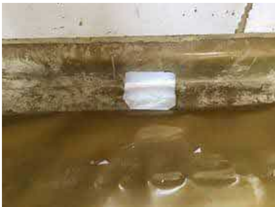
Plot 7 patch repair using SAGM.
