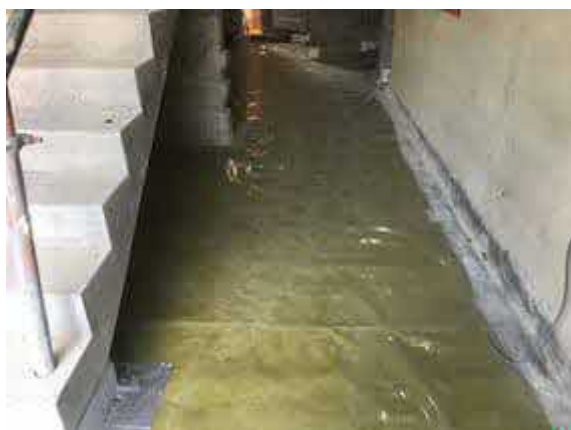
Over of installed membrane to apartment block c entrance lobby.
