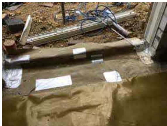
Plot 75 repaired damaged membrane using SAGM.
