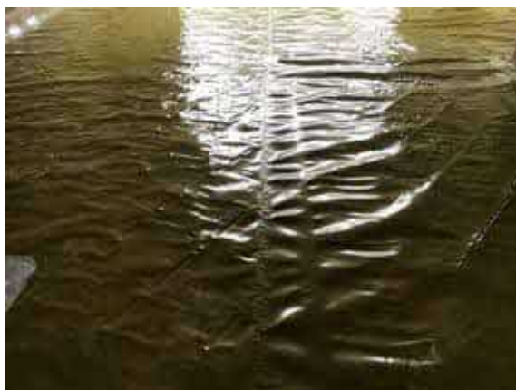
Plot 33 hand welded membrane lap.
