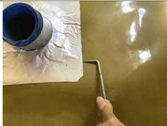
Pick testing all SAGM detailing to plot 67.
