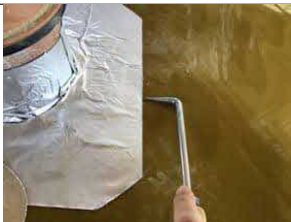
Plot 76 pick testing all SAGM detailing.
