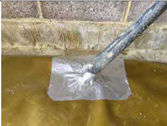
Pipe details within Plot 11 sealed with SAGM.
