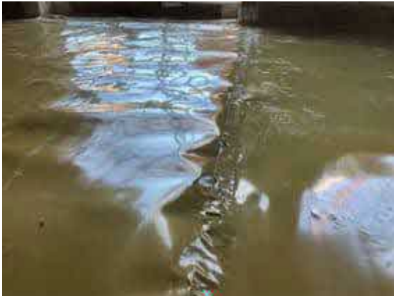
Plot 40. Hand welded membrane lap joint.
