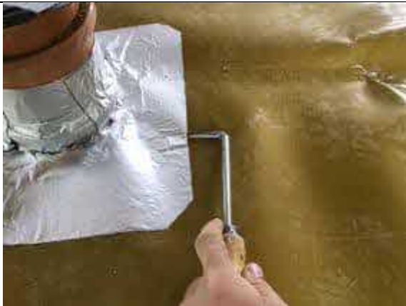
Pick testing all SAGM detailing.
