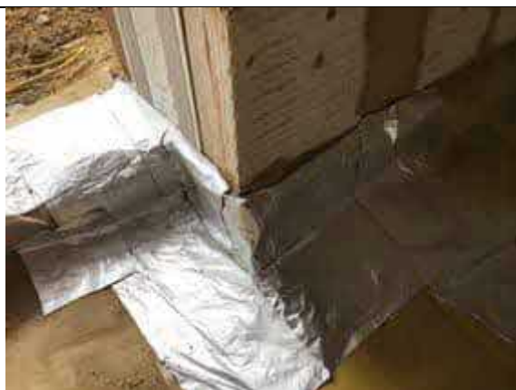
Plot 6 repaired door threshold detail using SAGM.
