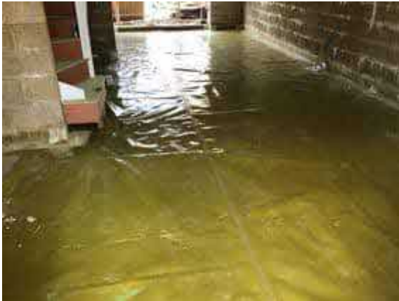
Overview of installed membrane to plot 49.
