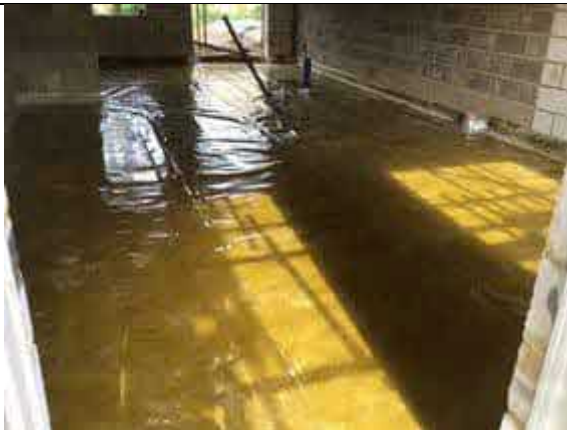
Plot 7 overview of installed membrane.
