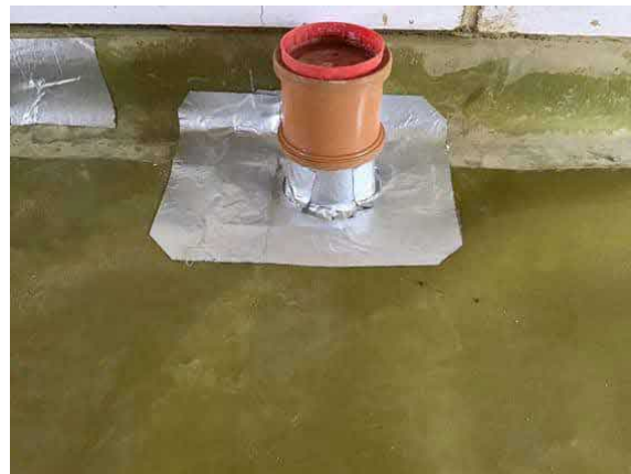
Typical pipe penetration seal using SAGM in plot 52.
