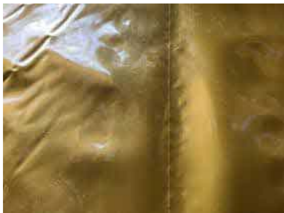
Plot 4 hand welded membrane lap.
