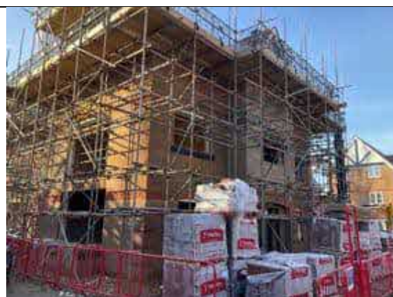
Plot 74 Overview where installation took place.
