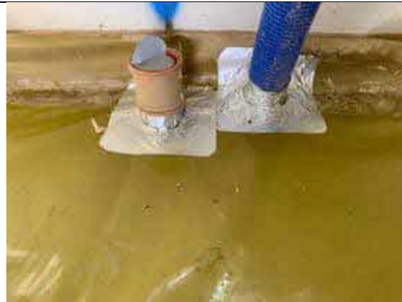
Plot 43 typical double pipe penetration seal using SAGM.
