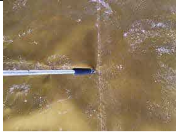
Air lancing all hand welded membrane laps.
