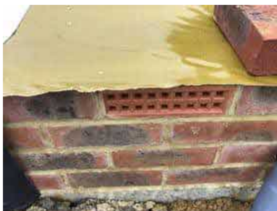
Plot 6 air brick in place.
