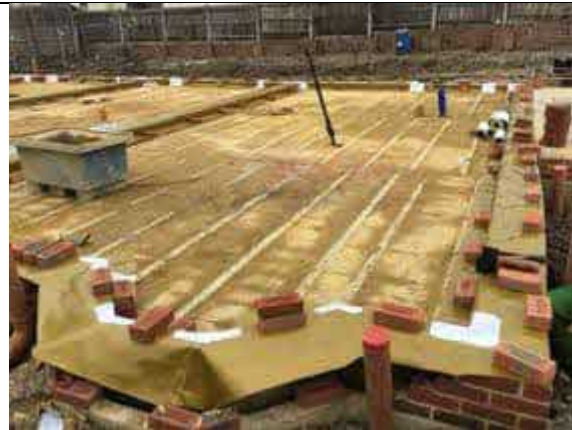
Plot 7 overview of installed membrane.
