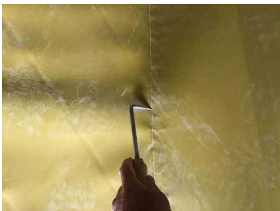
Pick testing all hand welded membrane laps.
