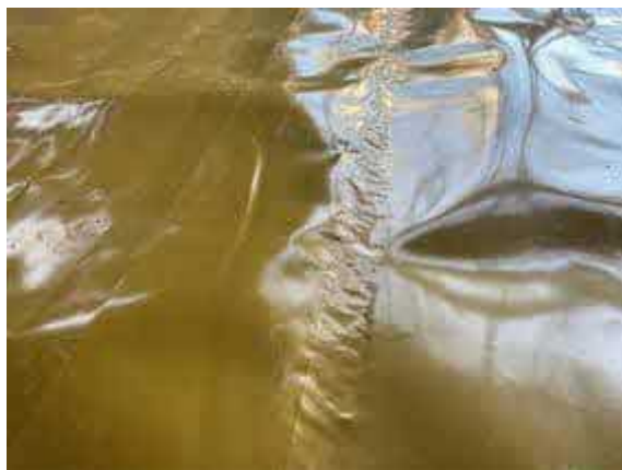
Plot 74. Hand welded membrane lap joint.
