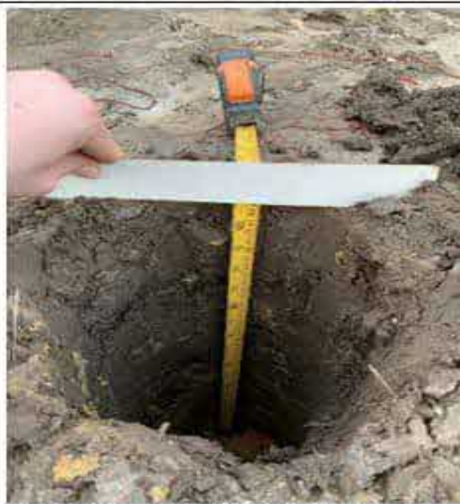
Photo 1: Plot 51 front garden showing depth to geotextile.
