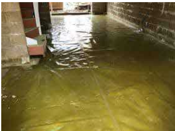
Overview of installed membrane to plot 49.
