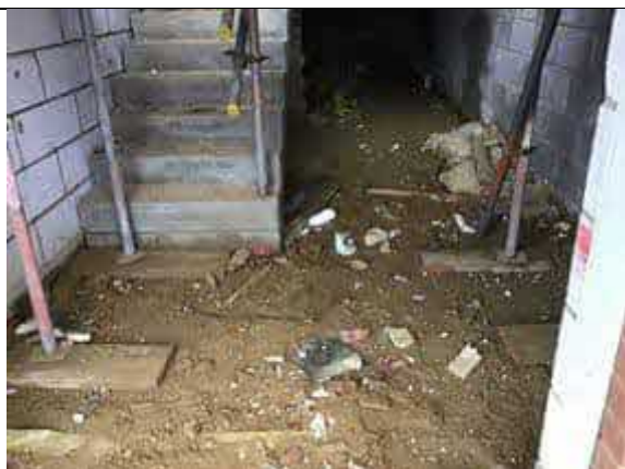
Incomplete stair lobby.
