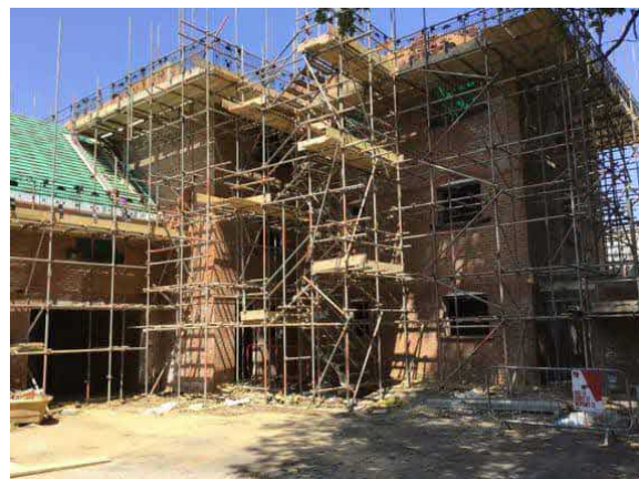
Overview of Apartment Block H. Plots 54-62.
