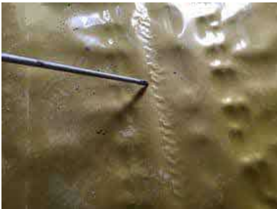
Plot 32 air lancing all welded membrane laps.
