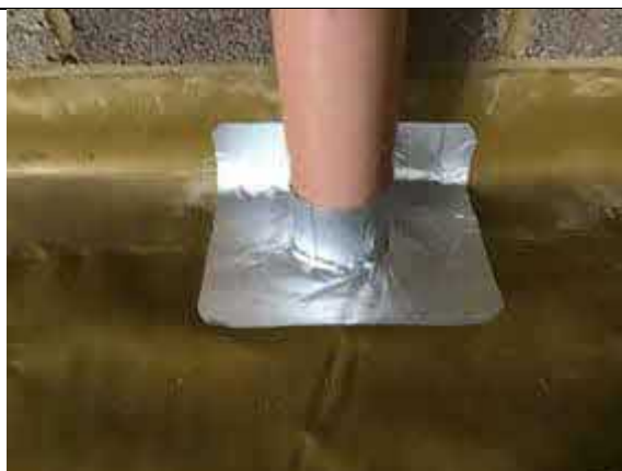
Typical pipe penetration seal using SAGM.
