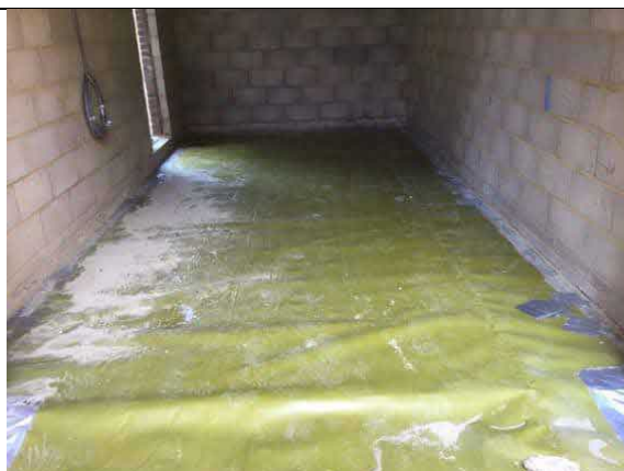
Overview of installed membrane to the garage, as an infill to plot 74.
