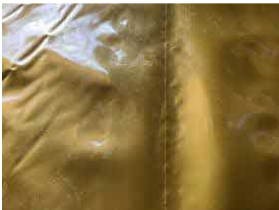
Plot 4 hand welded membrane lap.
