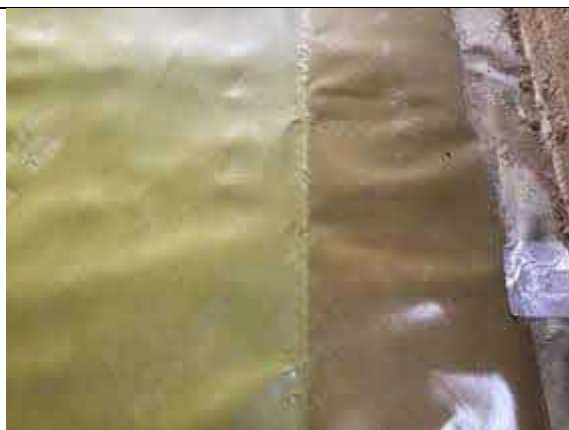
Hand welded membrane lap to plot 36.
