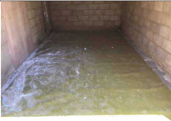
Overview of installed membrane to the garage, as an infill to plot 40.
