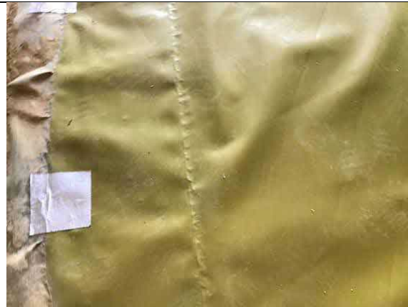
Hand welded membrane lap in garage plot 40.
