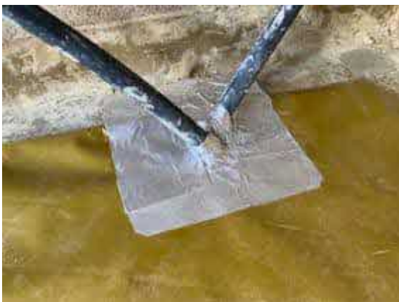
Plot 29 - Pipe penetration's sealed using SAGM.
