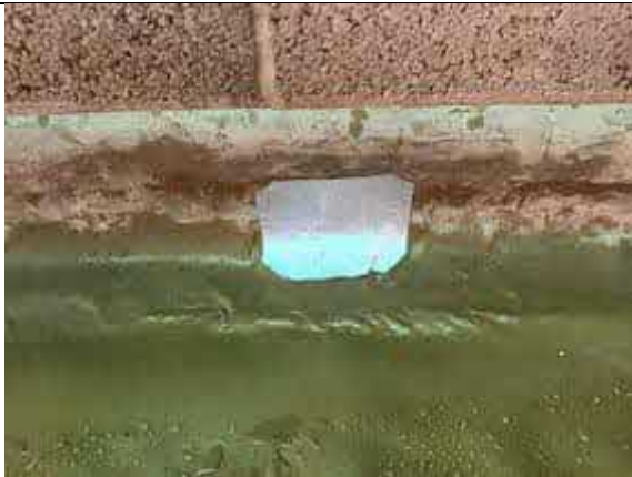
Plot 34 patch repair using SAGM to damaged perimeter membrane.
