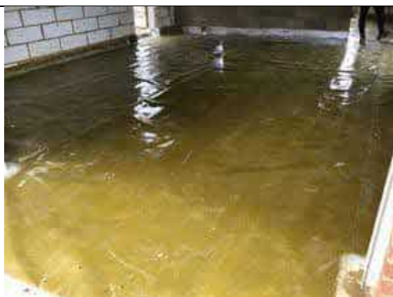
Overview of installed membrane.
