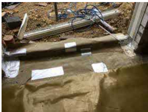
Plot 75 repaired damaged membrane using SAGM.
