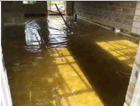
Plot 7 overview of installed membrane.
