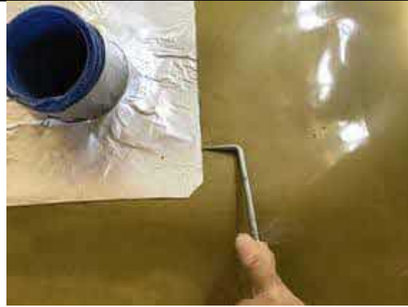
Pick testing all SAGM detailing to plot 67.
