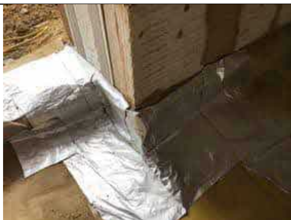
Plot 6 repaired door threshold detail using SAGM.
