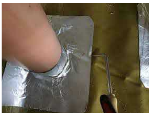
Pick testing all SAGM detailing.
