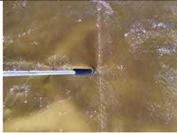
Air lancing all hand welded membrane laps.
