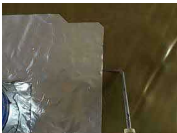
Pick testing all SAGM detailing to plot 64.
