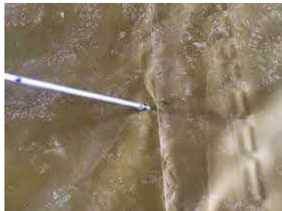
Plot 7 air lancing all welded membrane laps.
