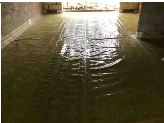
Hand welded membrane lap in plot 51.
