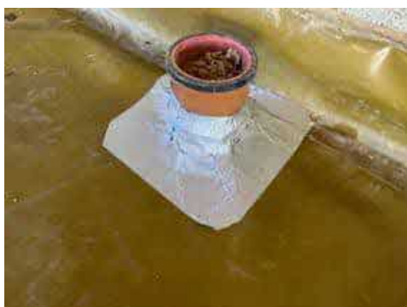
Plot 73. Typical pipe penetration sealed using SAGM.
