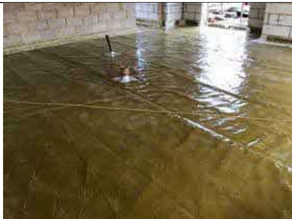
Plot 75 overview of installed membrane.
