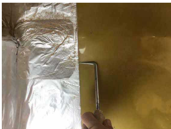
Pick testing all SAGM detailing.
