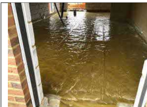
Overview of installed membrane to plot 27.
