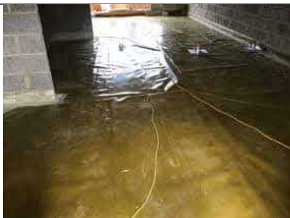
Plot 6 overview of installed membrane.
