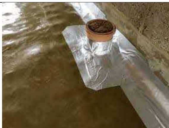
Plot 28 typical pipe penetration seal using SAGM.
