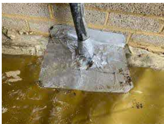
Plot 32 garage. Typical pipe penetration sealed using SAGM.
