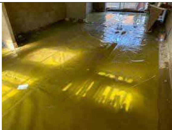
Plot 44 overview of installed membrane.
