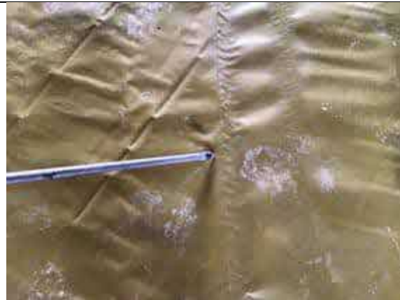
Plot 34 air lancing all welded membrane laps.
