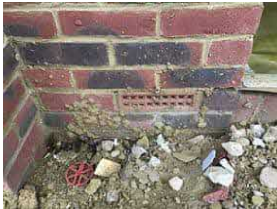
Air brick in place to plot 41.
