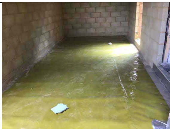
Overview of installed membrane to the garage, as an infill to plot 70.
