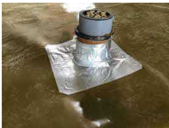
Typical pipe penetration seal using SAGM.
