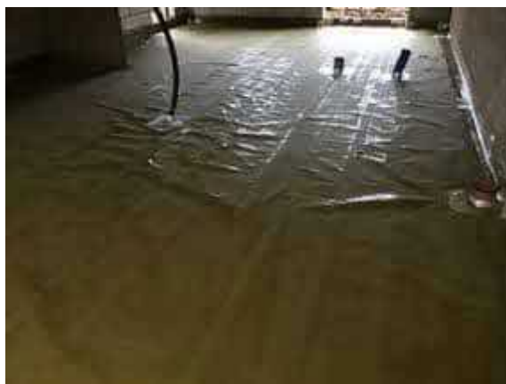
Overview of installed membrane to plot 39.
