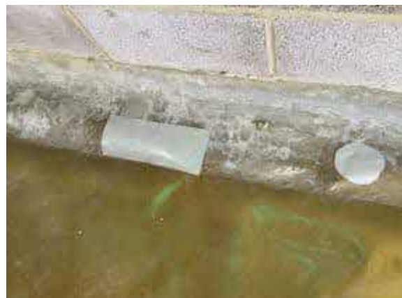
Plot 4 patch repair using SAGM.
