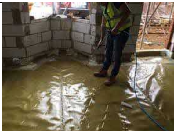
Air lance testing to Plot 10 lap joints.
