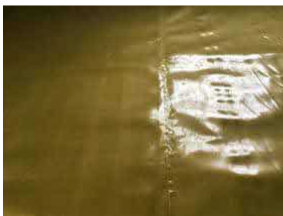
Hand welded membrane lap.
