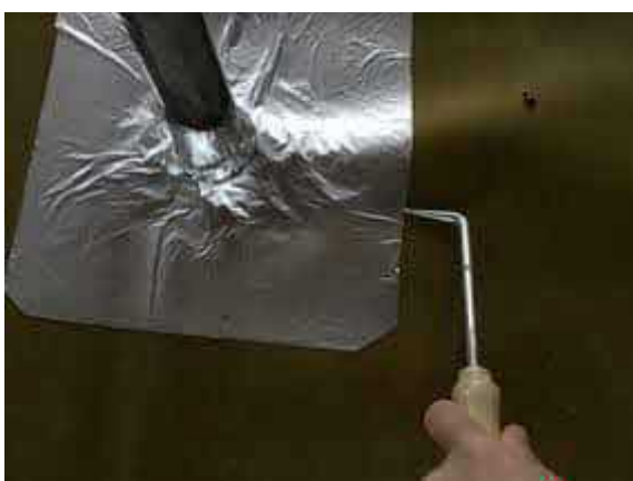
Pick testing all SAGM detailing to plot 38.
