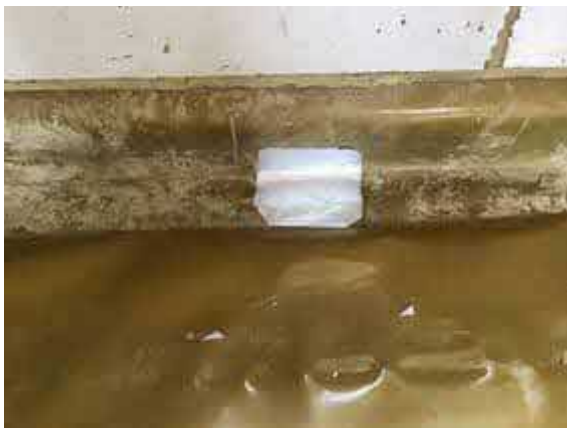
Plot 7 patch repair using SAGM.
