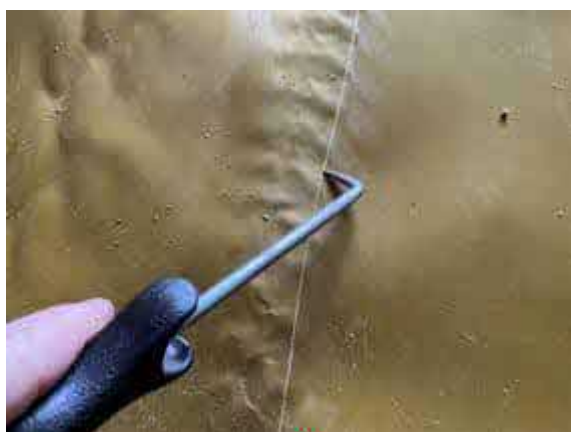
Plot 32 garage. Pick testing along hand welded lap joint.
