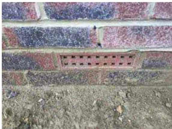
Air brick in place at the time of our inspection.
