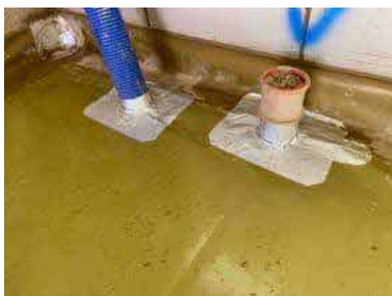
Plot 44 typical double pipe penetration seal using SAGM.
