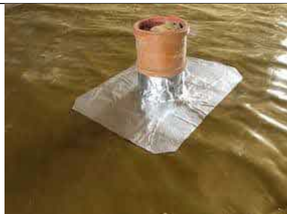
Plot 33 typical pipe penetration seal using SAGM.
