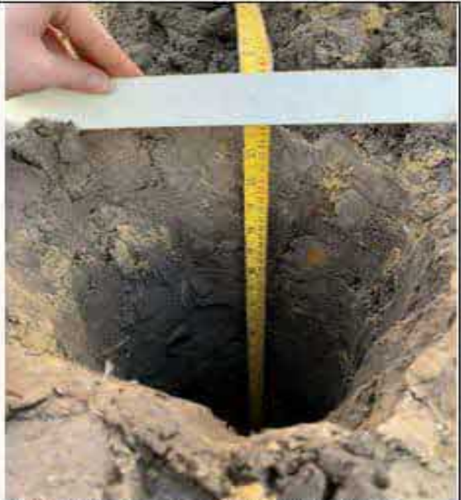
Photo 2: Plot 53 front garden showing depth to geotextile.
