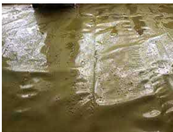
Hand welded membrane lap in plot 38.
