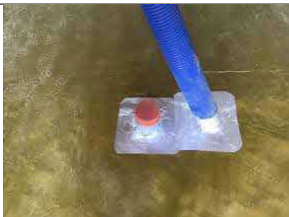
Plot 9 pipe penetrations sealed using SAGM
