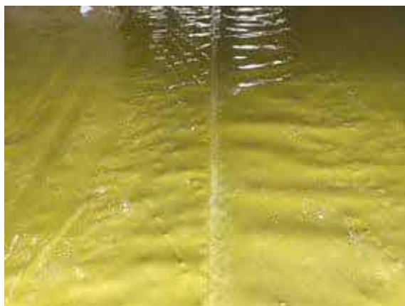
Hand welded membrane lap to plot 48.
