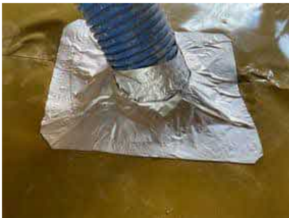
Plot 40. Typical pipe penetration sealed using SAGM.
