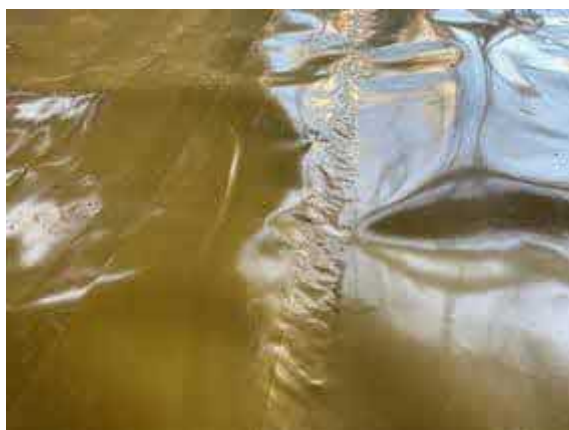
Plot 74. Hand welded membrane lap joint.
