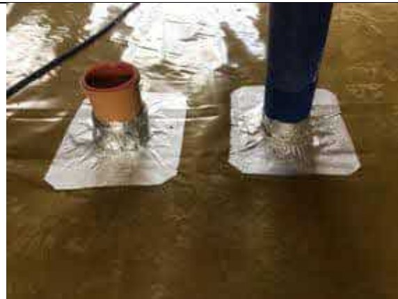
Plot 7 typical double pipe penetration seal using SAGM.
