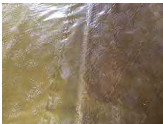
Plot 35 hand welded membrane laps.
