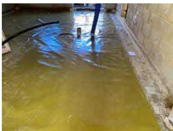
Plot 45 overview of installed membrane.
