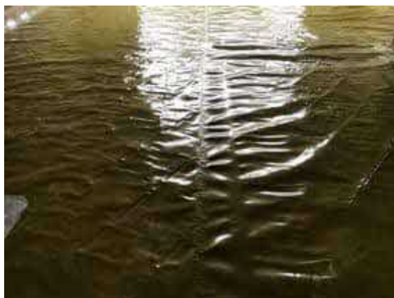
Plot 33 hand welded membrane lap.
