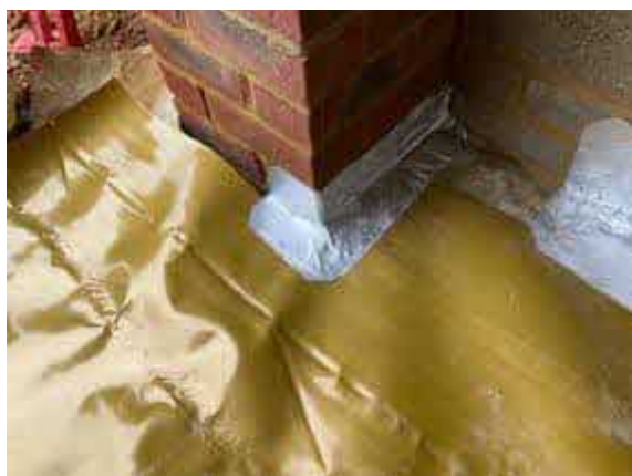
Plot 35 garage. Corner detailing sealed using SAGM.
