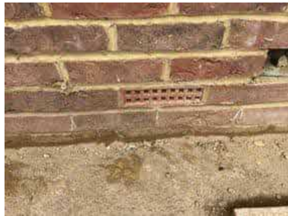
Plot 32 air brick in place at the time of our inspection.
