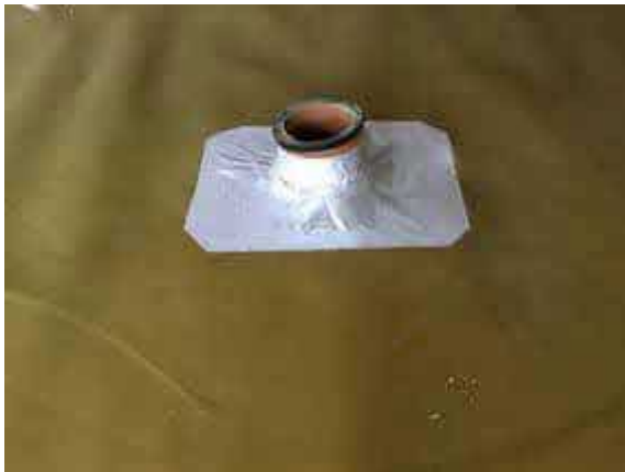
Typical pipe penetration seal to plot 41.
