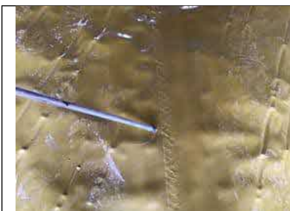
Plot 27 air lancing all weld laps.
