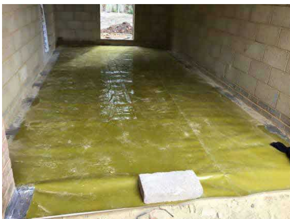
Overview of installed membrane in garage plot 67.
