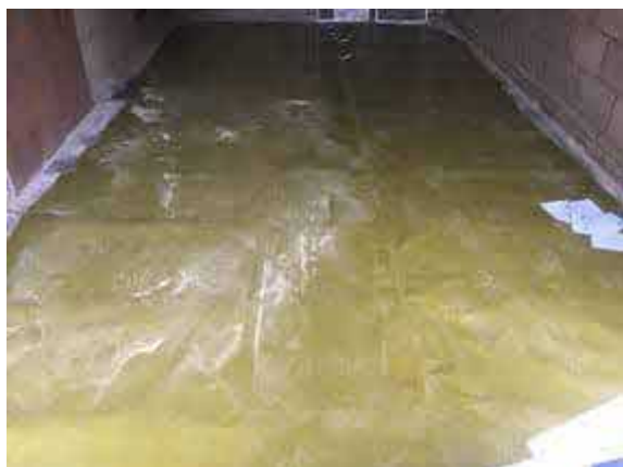
Overview of installed membrane to garage area to plot 38.
