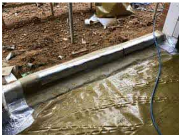
Repaired damaged to the door threshold due to follow on trades using SAGM.
