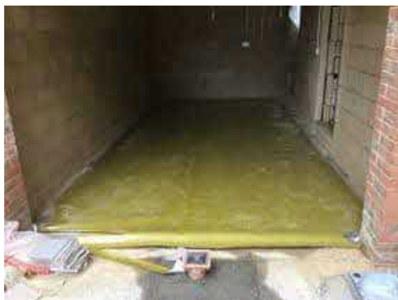
Overview of installed membrane to garage area to plot 39.
