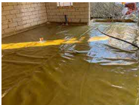
Plot 74. Overview of installation of Visqueen HC Blok gas barrier.
