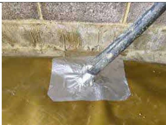
Pipe details within Plot 11 sealed with SAGM.
