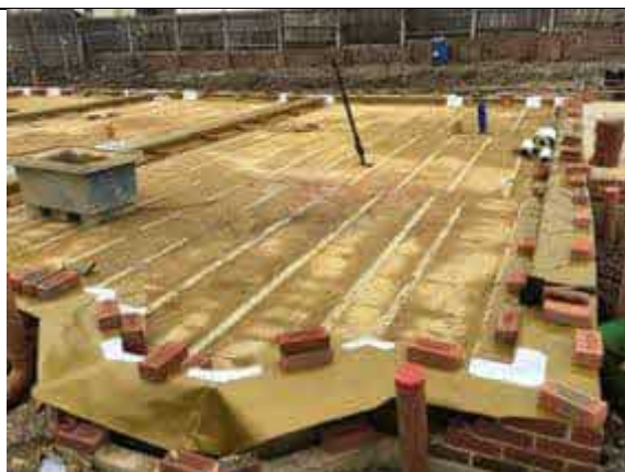
Plot 7 overview of installed membrane.
