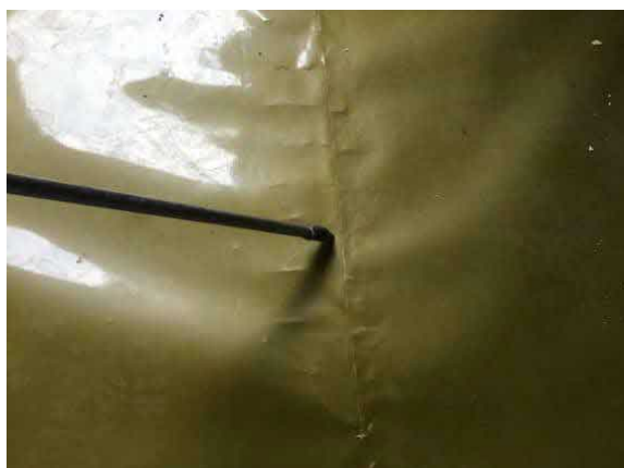
Air lancing all hand welded membrane laps.
