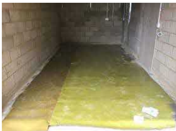
Overview of installed membrane to garage area in plot 37.
