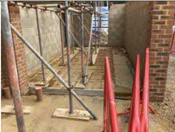
Plot 35 attached garage incomplete at the time of our inspection.
