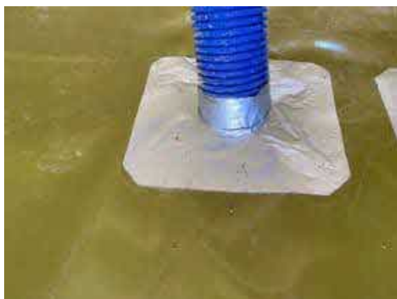
Plot 45 typical pipe penetration seal using SAGM.
