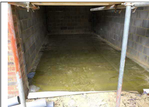
Overview of installed membrane in garage plot 63.
