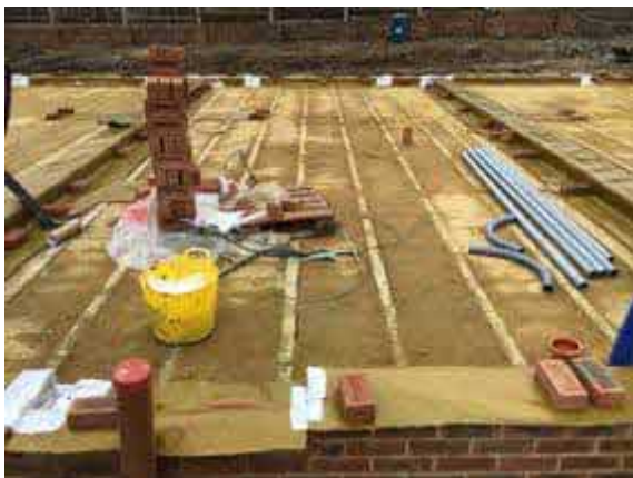
Plot 6 overview of installed membrane.
