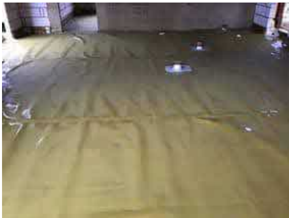
Overview of installed membrane to plot 41.
