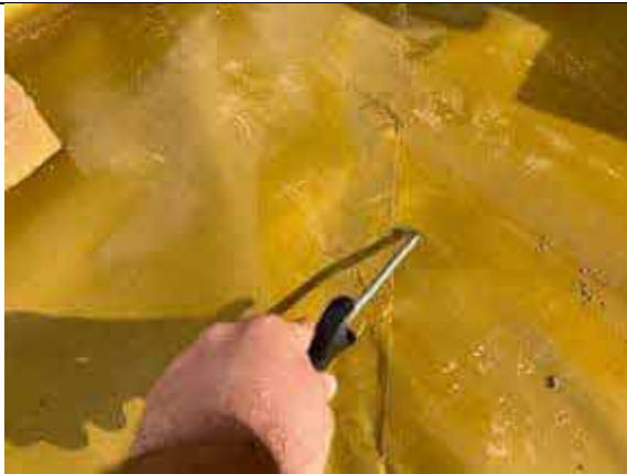
Plot 63 FOG Unit - Pick test upon a successfully hand welded lap joint.
