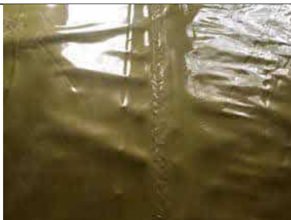
Hand welded membrane lap to plot 64.
