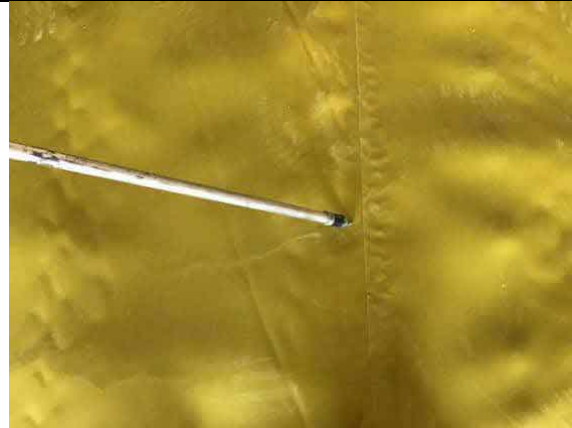
Air lancing all hand welded membrane laps in apartment block H.
