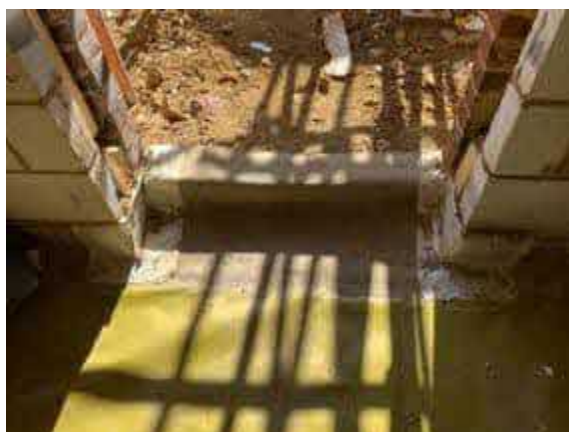
Plot 45 sealed door threshold detail using SAGM.
