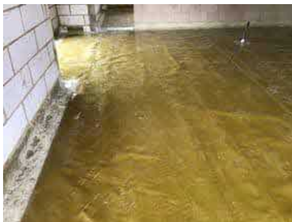
Plot 76 overview of installed membrane.
