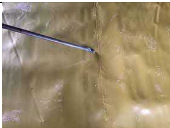
Air lancing all welded membrane laps.
