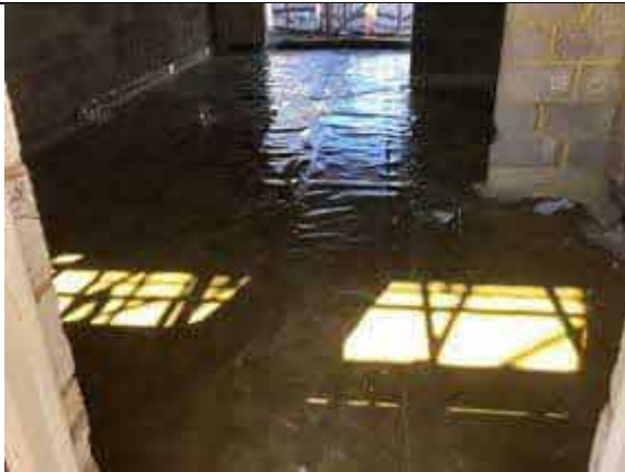
Plot 5 overview of installed membrane.
