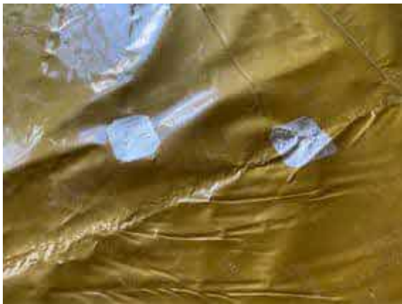
Plot 30 - Patch repairs using SAGM.
