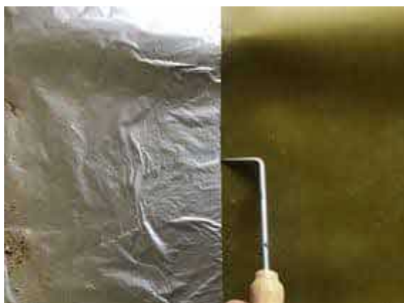
Pick testing all SAGM patches to damaged perimeter membrane to plot 37.
