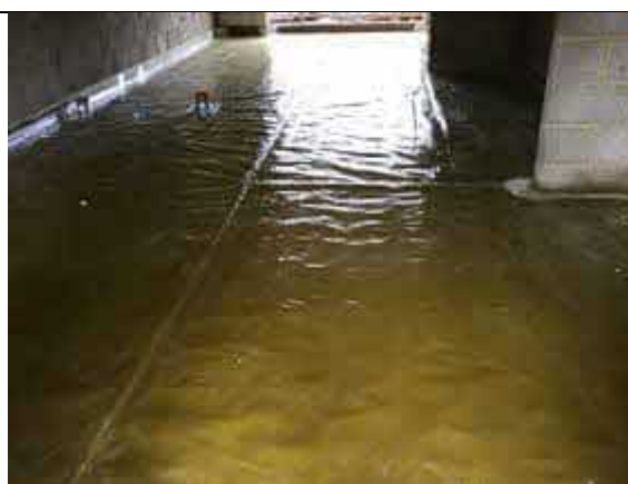
Overview of installed membrane to plot 28.
