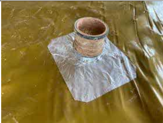
Plot 72. Typical pipe penetration sealed with SAGM.
