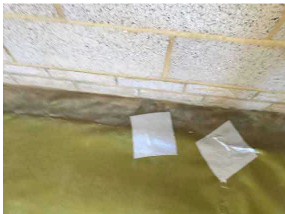
Patch repairs using SAGM to damaged membrane.
