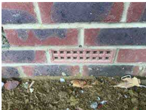
5no air bricks per plot were in place at the time of our inspection.
