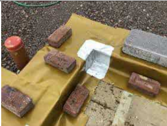
Plot 73 typical corner seal using SAGM.
