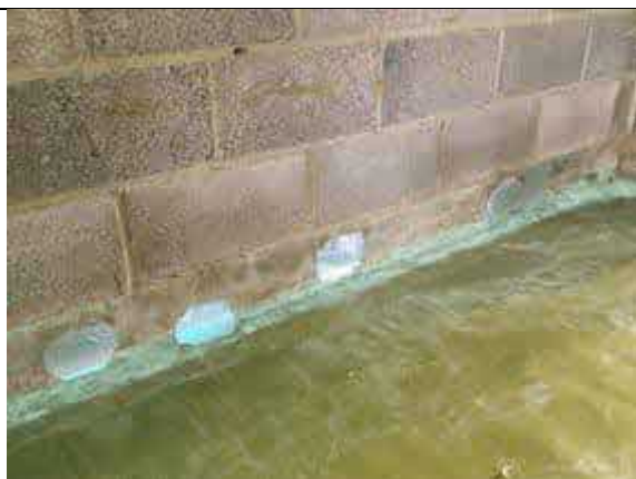
SAGM patches applied prior to inspection to the perimeter membrane within Plot 10.
