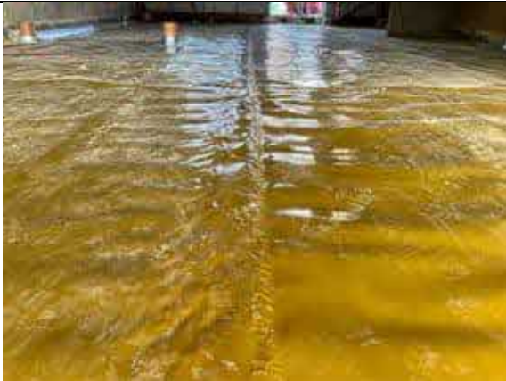
Plot 29 - Successfully hand welded membrane lap joint.
