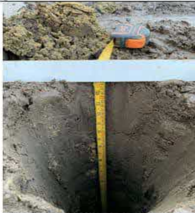
Photo 3: Plot 52 rear garden showing depth to geotextile.
