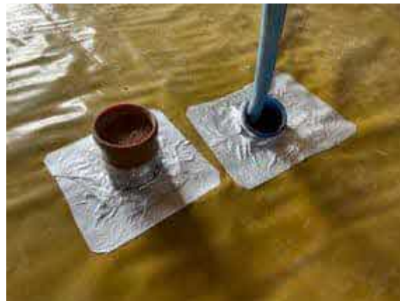
Plot 30 - Typical pipe penetration's sealed using SAGM.
