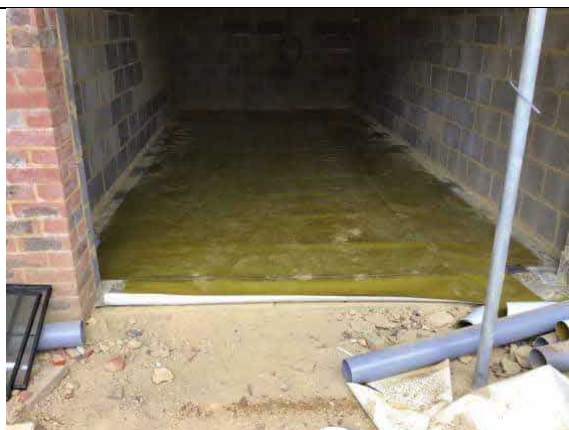
Overview of installed membrane in garage plot 64.
