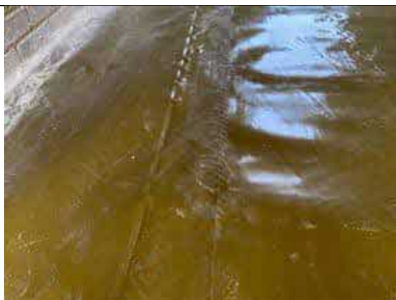
Plot 35 garage. Overview of a hand welded membrane lap joint.
