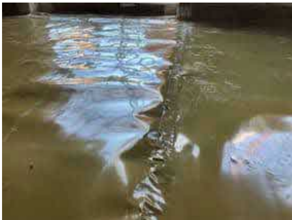
Plot 40. Hand welded membrane lap joint.
