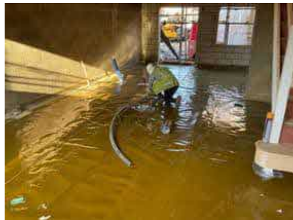
Plot 40. Overview of installation of Visqueen HC Blok gas barrier.
