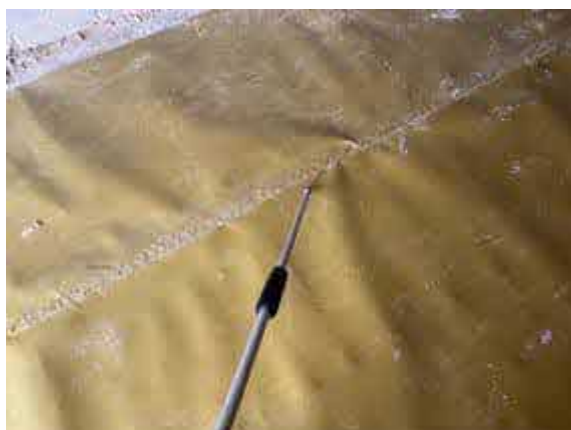
Plot 30 garage. Air lance integrity test upon welded lap joint.
