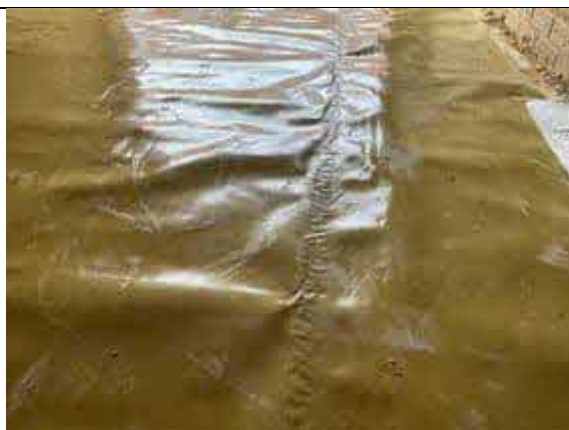
Plot 30 garage. Overview of a hand welded membrane lap joint.
