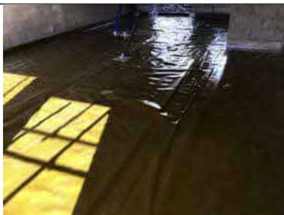
Plot 3 overview of installed membrane.
