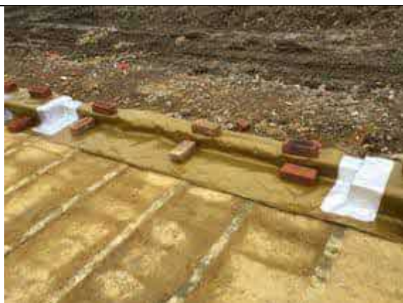
Plot 6 typical door threshold seal using SAGM.
