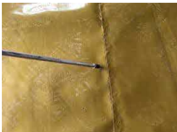
Air lancing all welded membrane laps.
