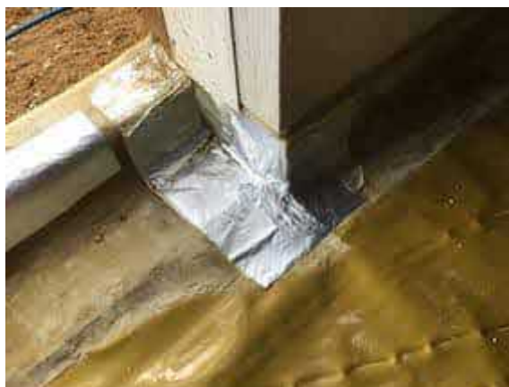
Sealed corner detail using SAGM.
