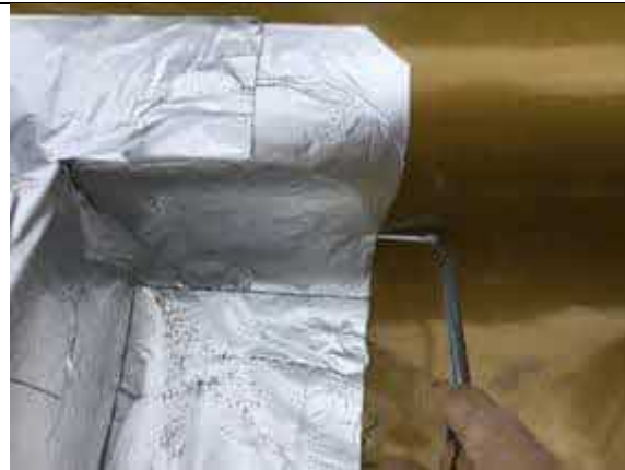
Plot 74 pick testing all SAGM detailing.
