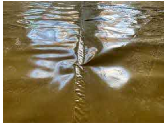
Plot 30 - Hand welded membrane lap joint.
