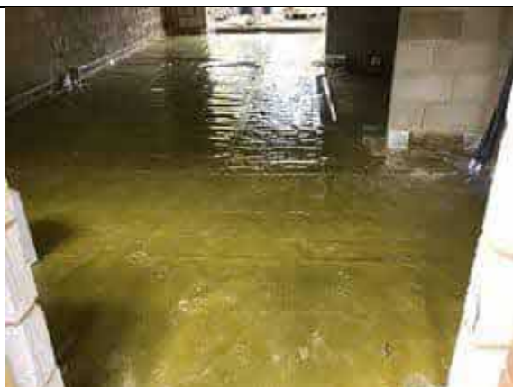
Overview of installed membrane to plot 48.
