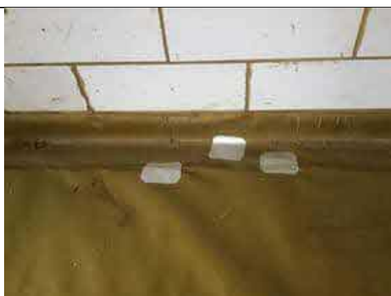
Patch repairs using SAGM to plot 36.
