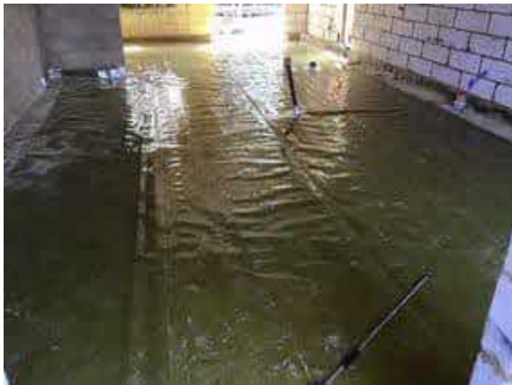
Overview of installed membrane to plot 67.
