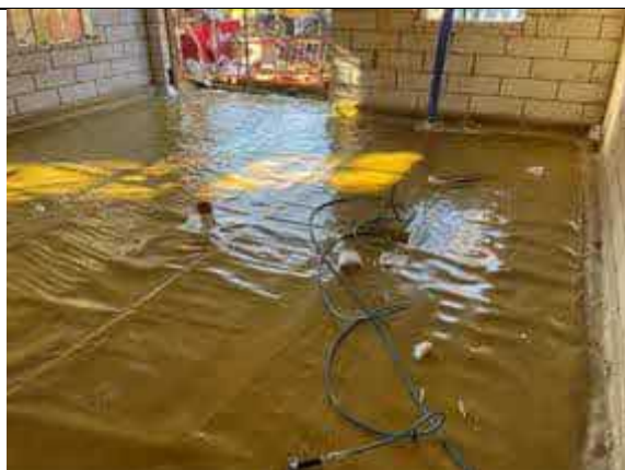
Plot 73. Visqueen HC Blok infill installation.
