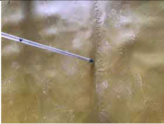
Air lancing all hand welded membrane laps to plot 66.
