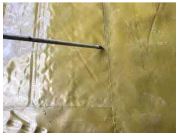
Plot 75 air lancing all weld laps and SAGM detailing.
