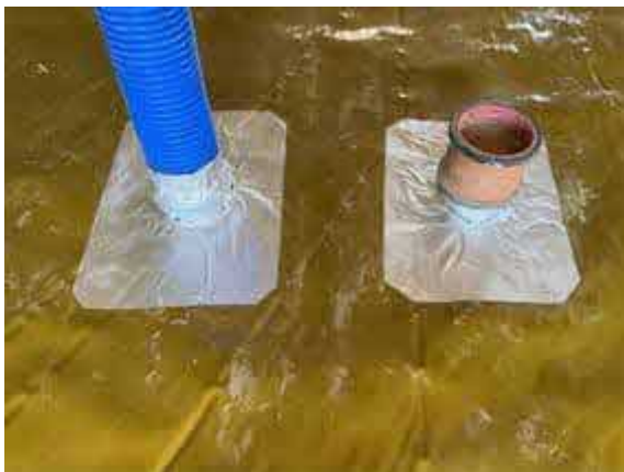
Plot 70. Typical pipe penetration's sealed using SAGM.
