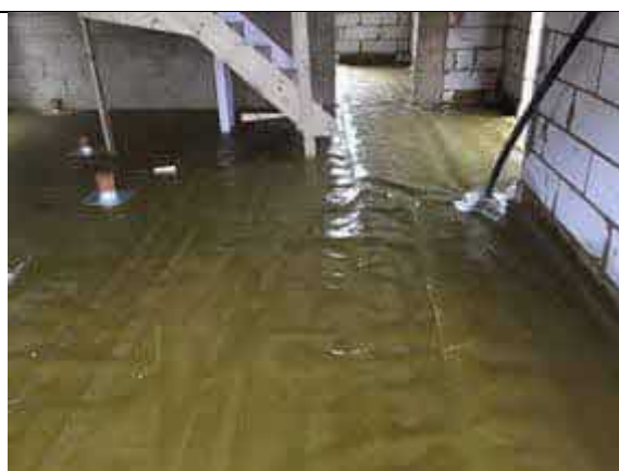
Overview of installed membrane to plot 36.
