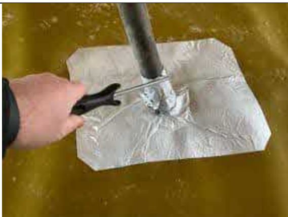
Plot 70. Pick test conducted upon sealed pipe penetration.
