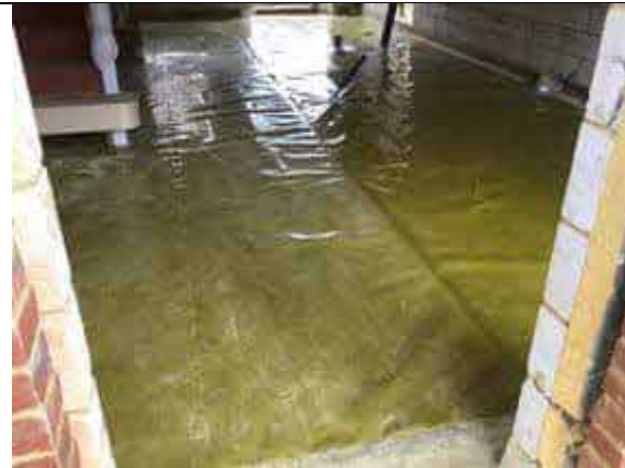
Overview of installed membrane to plot 50.
