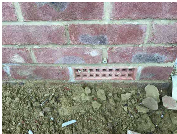
Air brick in place at the time of our inspection to plots 51-53.
