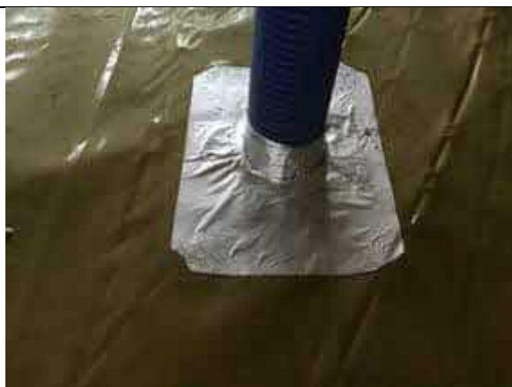
Typical pipe penetration seal using SAGM to plot 37.
