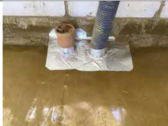
Plot 5 typical double pipe penetration seal using SAGM.
