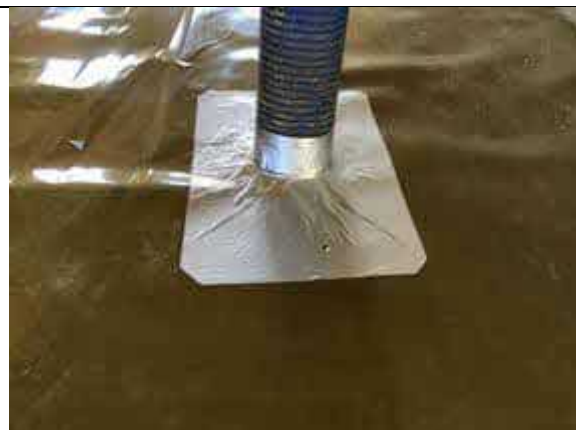
Plot 4 typical pipe penetration seal using SAGM.
