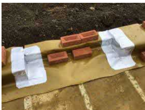
Plot 7 typical door seal using SAGM.
