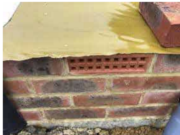
Plot 6 air brick in place.
