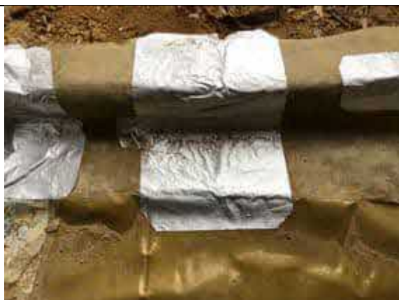
Plot 27 patch repair using SAGM to damage caused by follow on trades.
