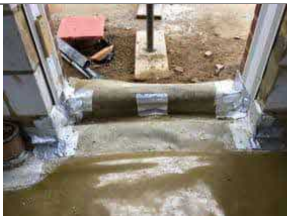
Door threshold seal using SAGM.
