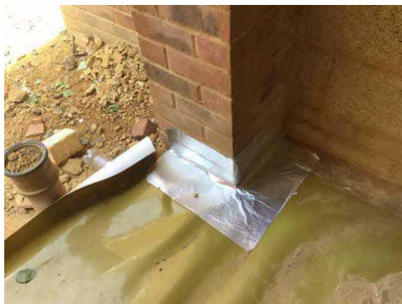
Sealed front of garage using SAGM.
