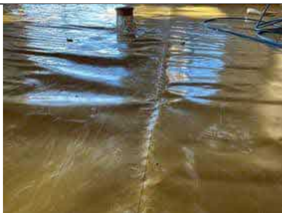
Plot 73. Hand welded membrane lap joint.
