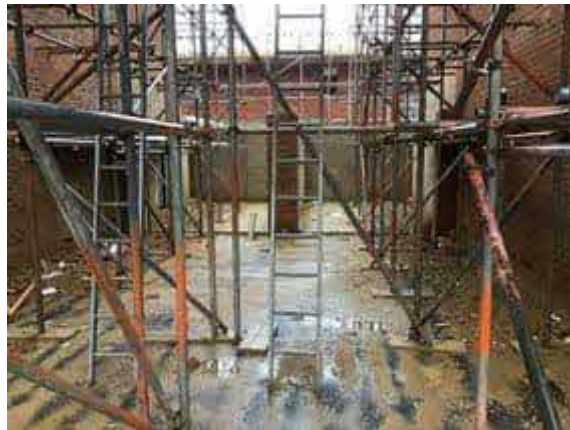
Scaffolding in place in all garages.
