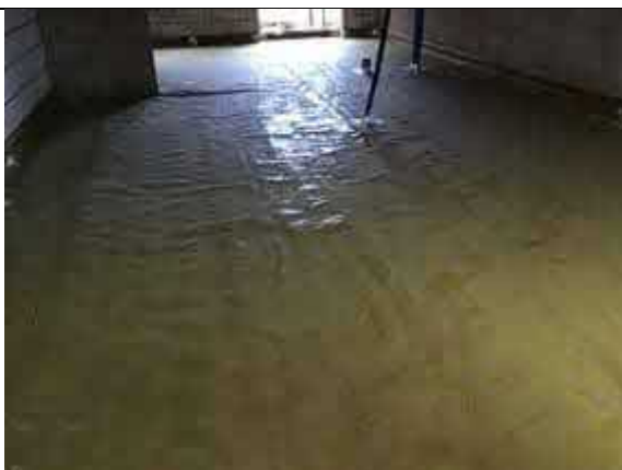
Overview of installed membrane to plot 37.
