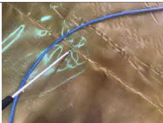
Plot 9 hand welded joint being air lanced
