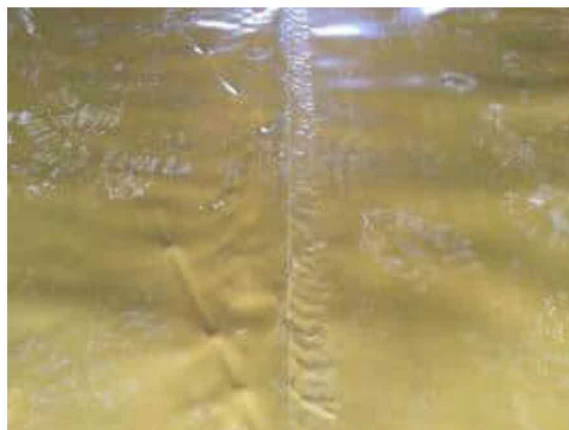
Overview looking down the hand welded lap joint.
