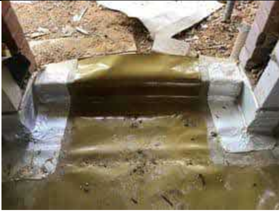
Sealed door threshold using SAGM.
