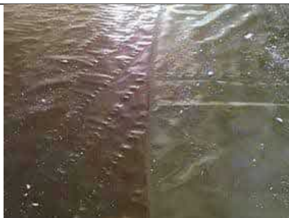
Hand welded membrane lap to plot 65.
