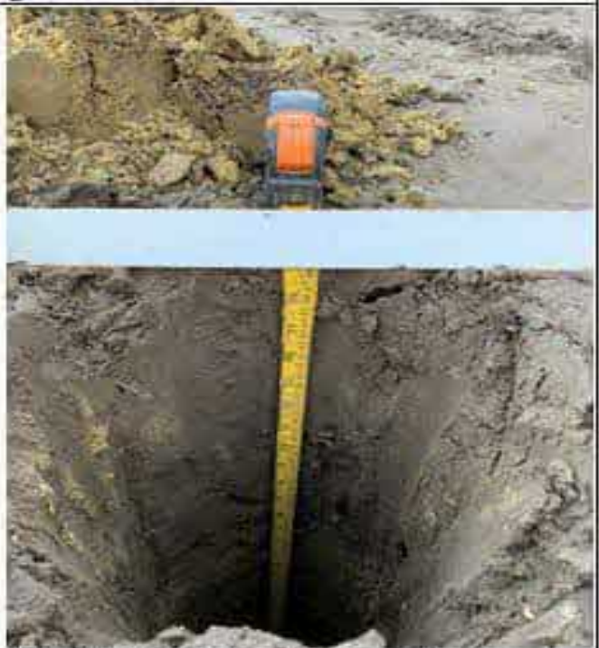
Photo 4: Plot 53 rear garden showing depth to geotextile.
