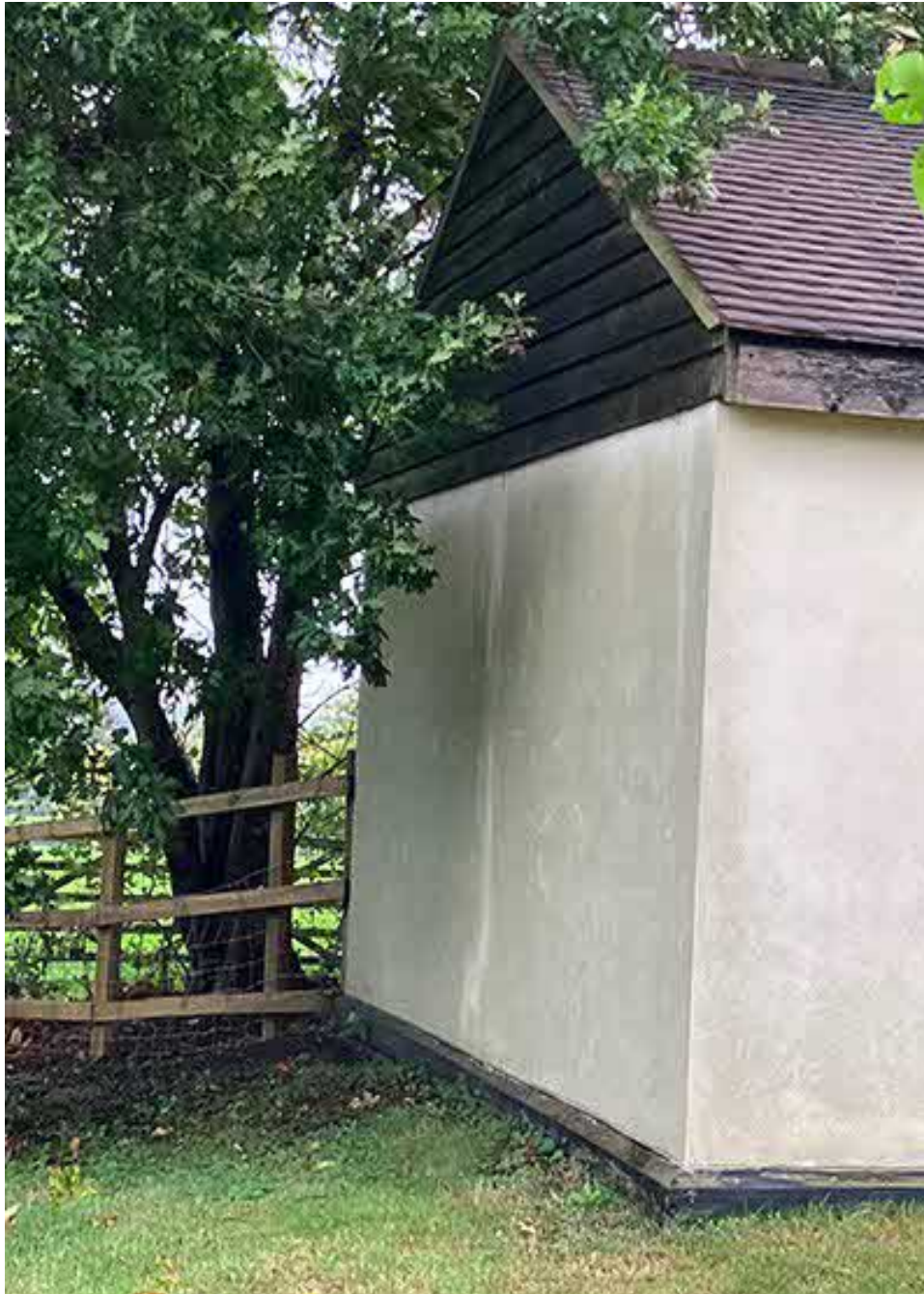
Above: View of side of outbuilding (Structure 3)
