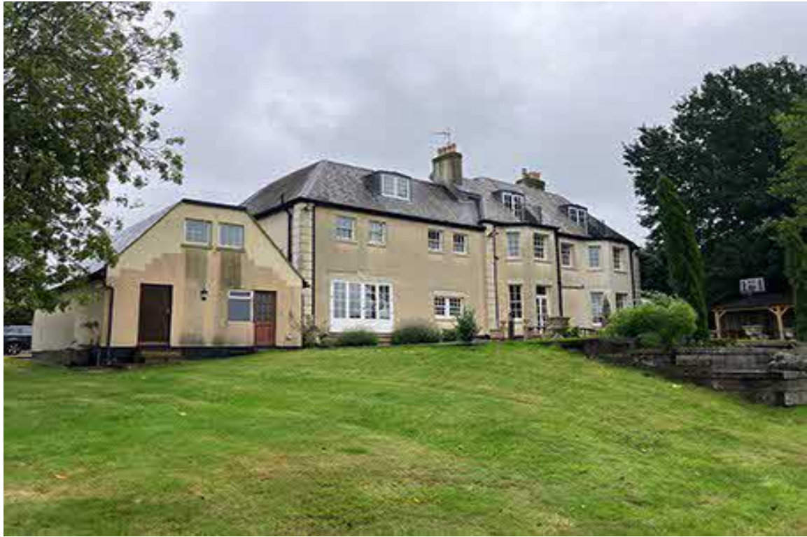
Above: View of rear of house and garage
