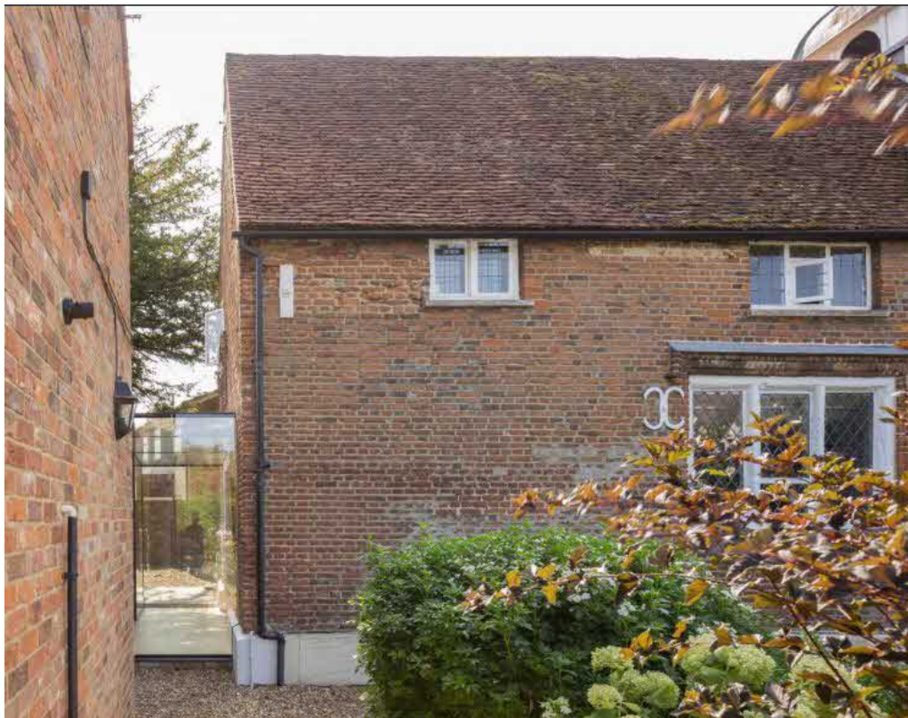
Above: Stewart & Stewart previous project near Ware – minimally detailed glazed link between Grade II* Listed Building & new extension.
