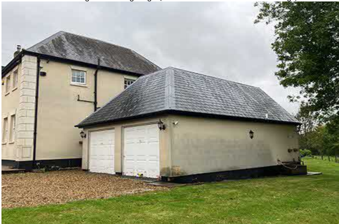
Below: View of existing detached garage (Structure 1 on associated drawings)
