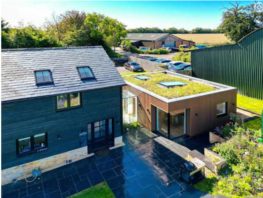
Above: Stewart & Stewart previous project near Hitchin – minimally glazed link connecting main house to ‘home-schooling’ extension
