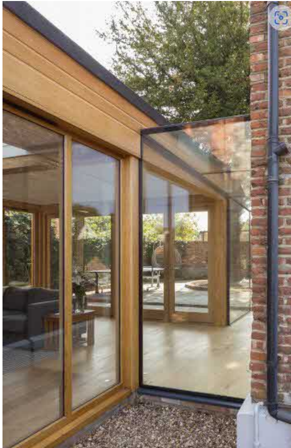
Above: Stewart & Stewart previous project near Ware – minimally detailed glazed link between Grade II* Listed Building & new extension.
