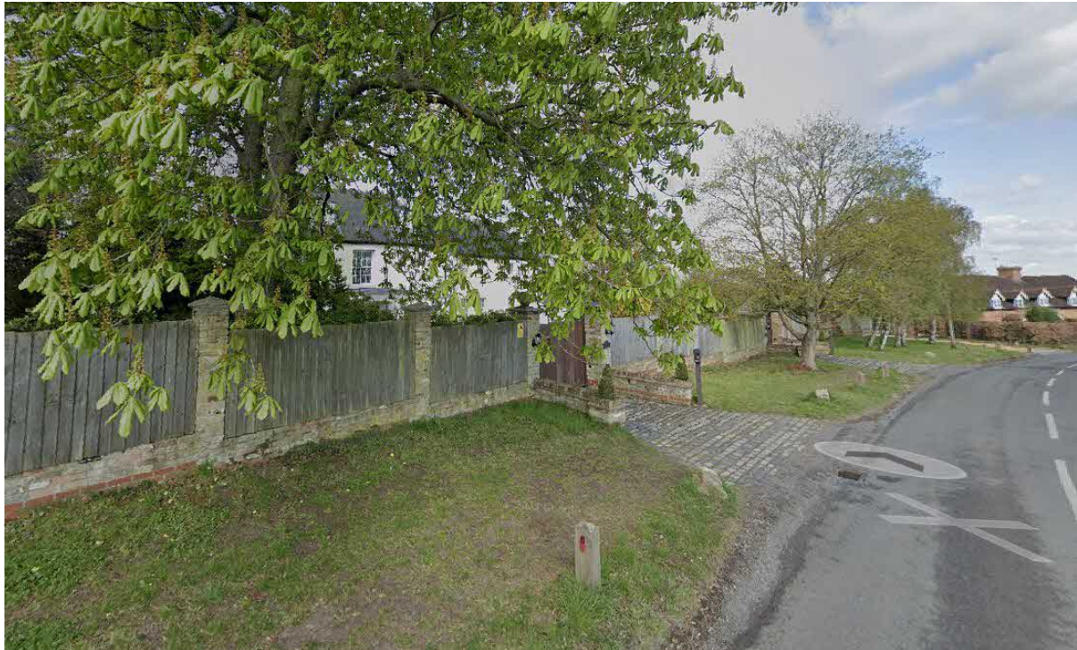
View above: Taken from highway of front boundary.
