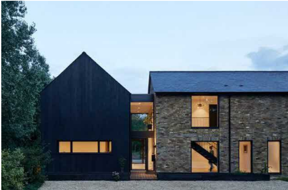
Above: Example of glazed link connected to contrasting clad structures – i.e. brick & dark stained timber cladding.
