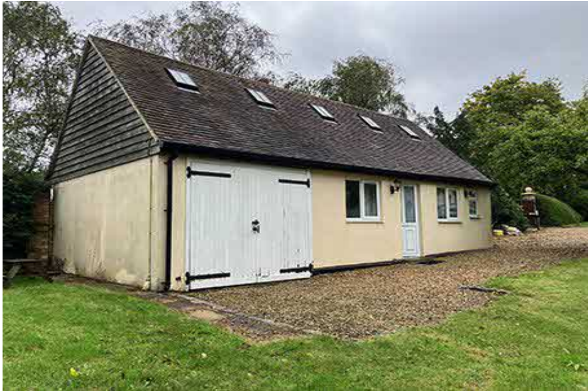
Above: View of front of the garage/annexe (Structure 2 on the associated drawings)
