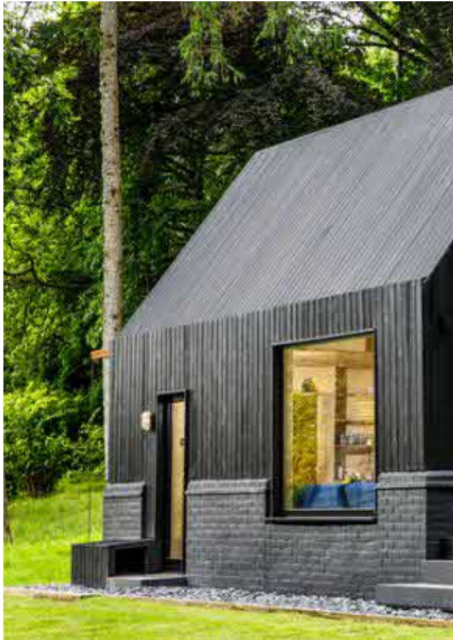
Above: Example of dark stained timber cladding walls & continuous roof finishes
