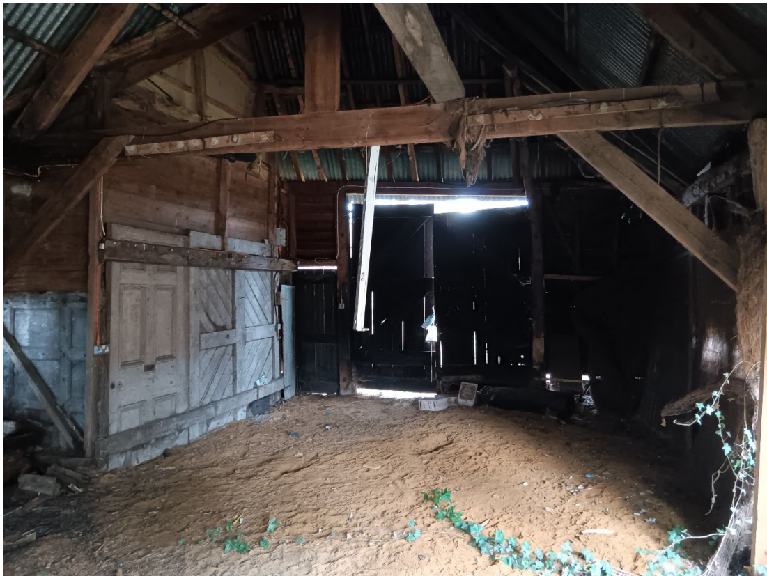
Interior of barn
