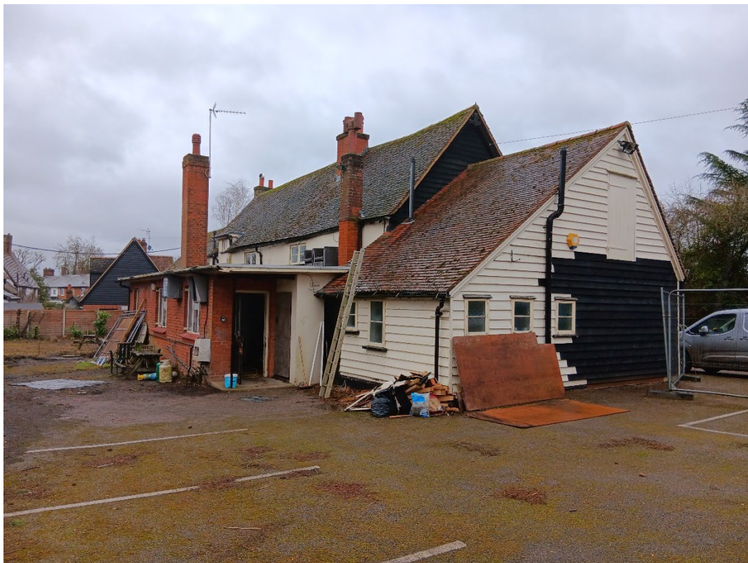
Rear of public house
