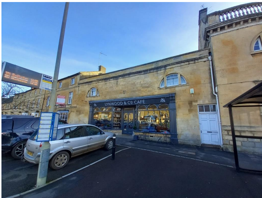
Above: North wing of The Corn Exchange.
