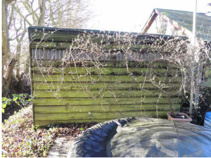
Photo 7: North-western elevation of the garage
