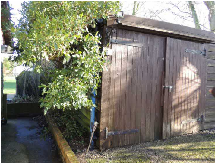
Photo 8: South-western elevation of the garage
