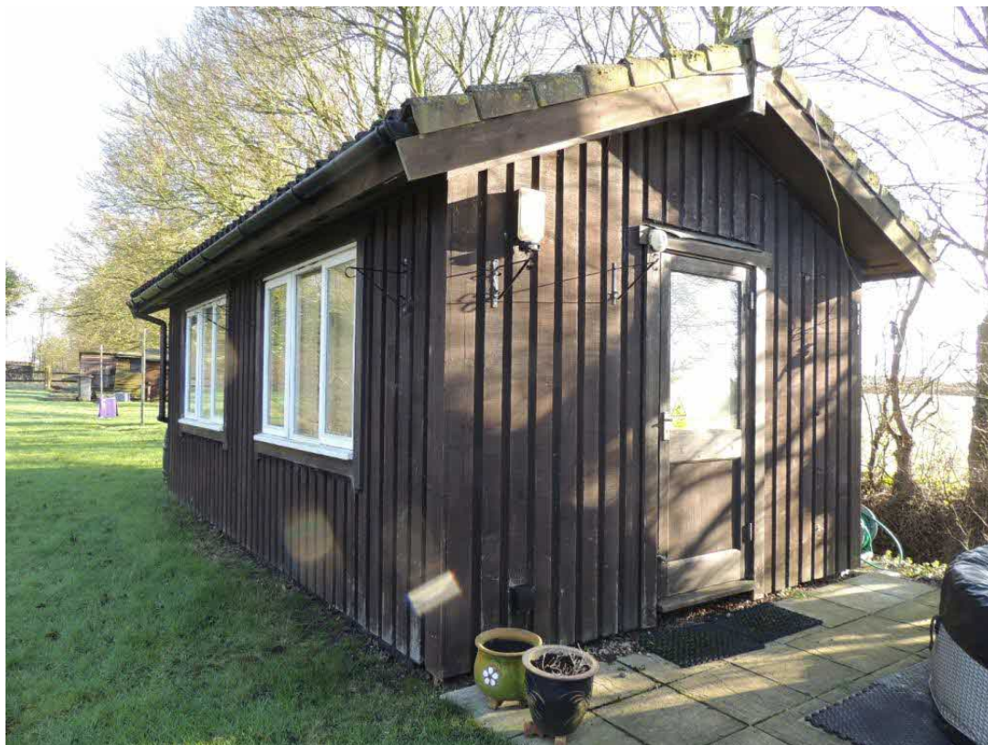
Photo 1: South-western (gabled) and north-western elevations of the office. The proposal is to demolish and replace the office and garage with a residential annexe
