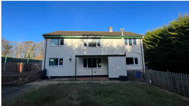
View to rear of building as existing.
