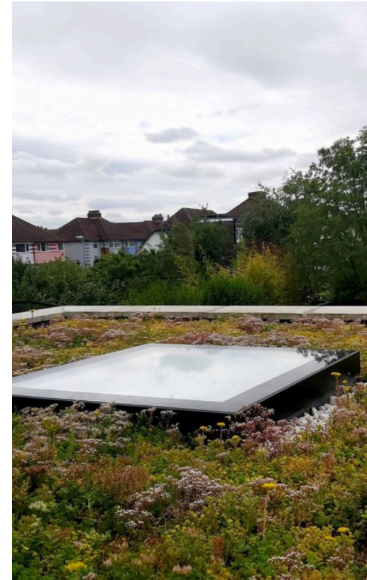
Example of flat rooflights and sedum coverings as proposed for the rear extension.
