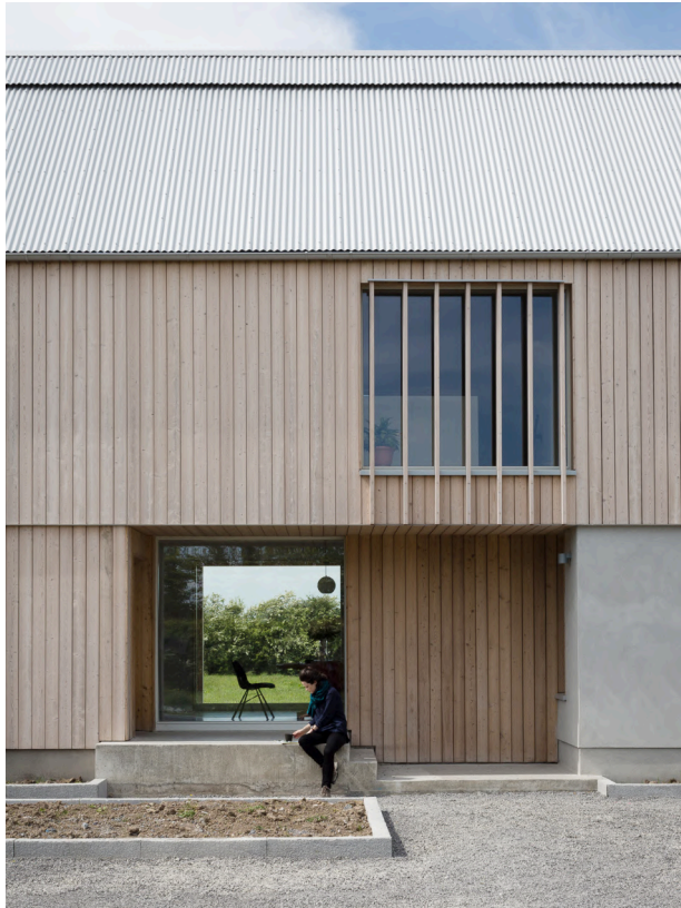
Example of close boarded vertical timber cladding as proposed for the rear extension, left unfinished and allowed to mellow and weather down naturally.
