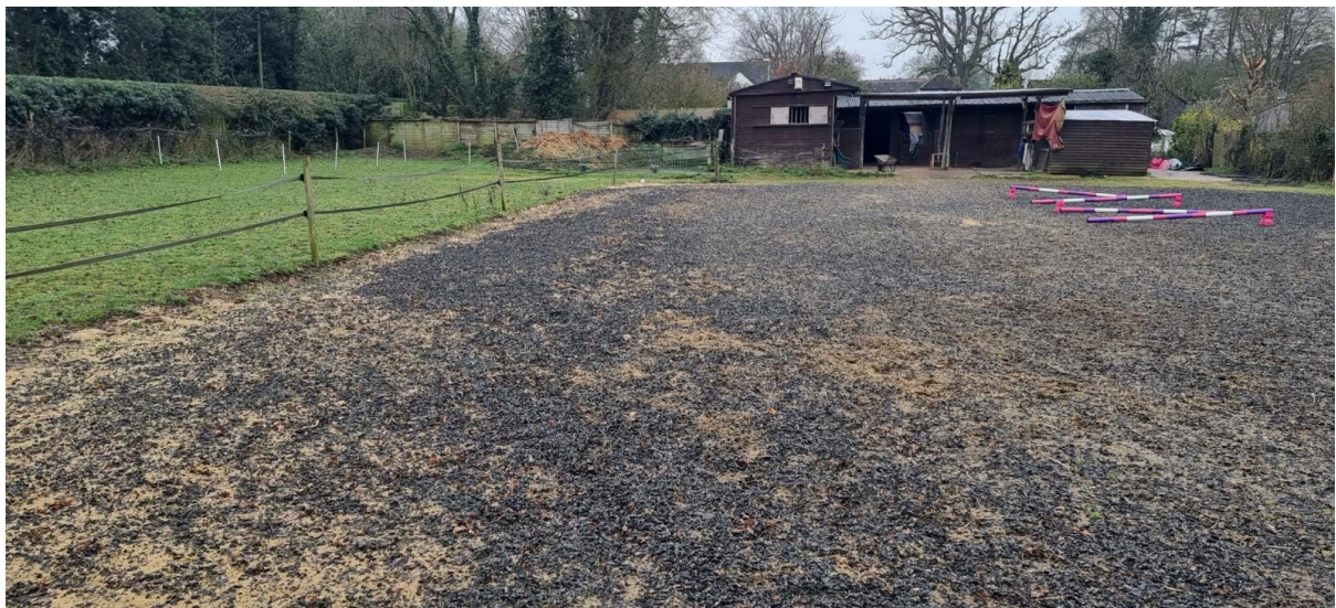
Image 3: original stable building and riding arena on the site, taken prior to the works being undertaken
