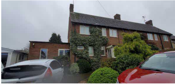
1 Front – north aspect
