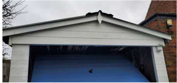
10 Garage north aspect
