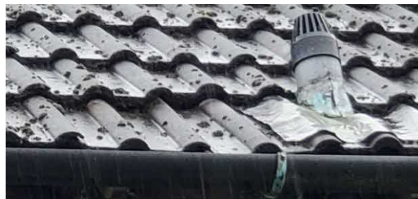
6 Gaps to tiles near flue on north aspect
