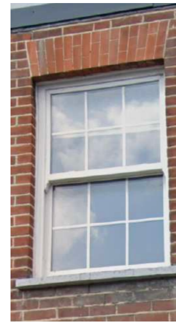
SASH WINDOWS - 6 OVER 6 FORMATION
