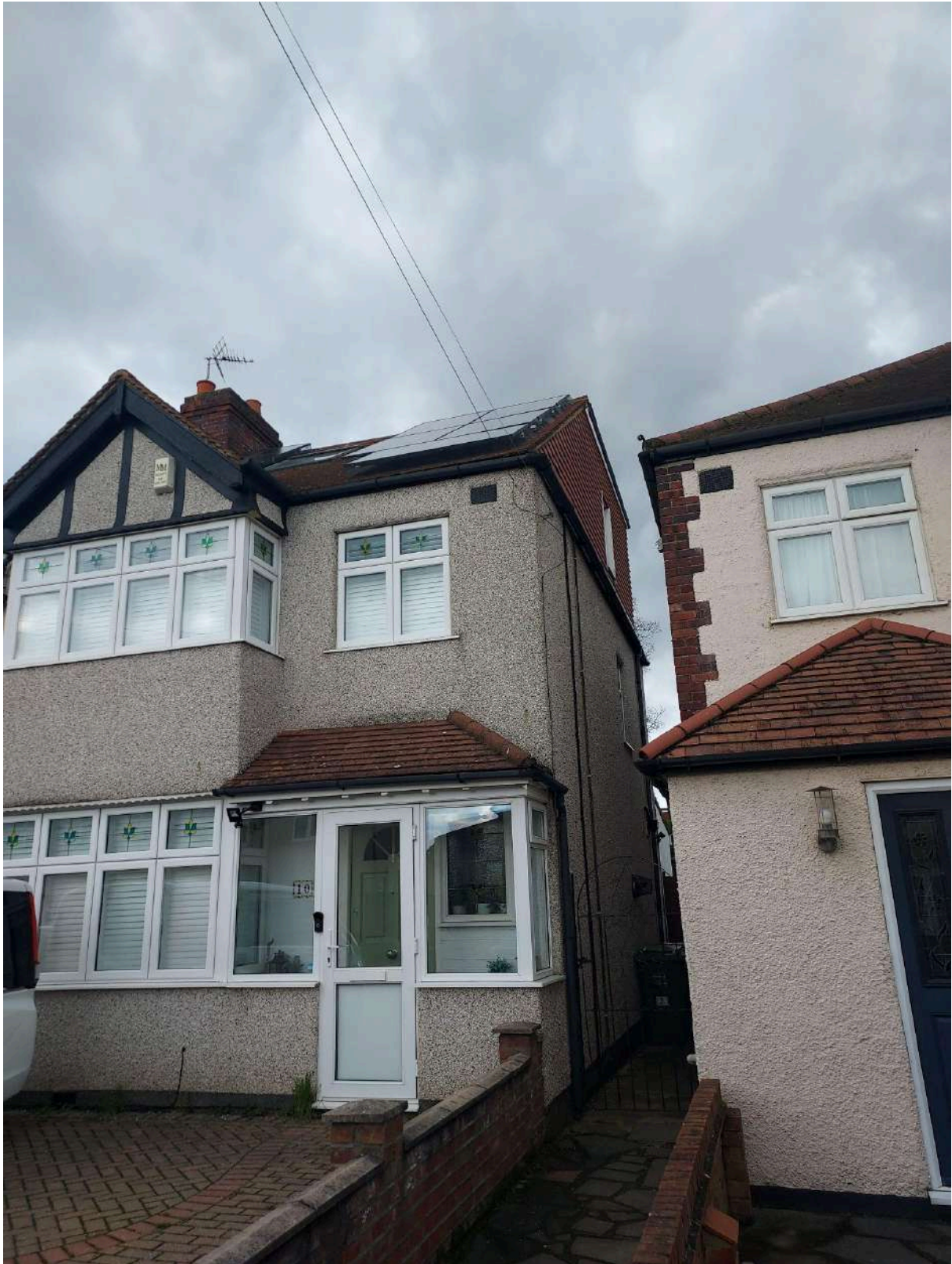
10 Buxton Crescent-Terraced house Hip to gable with full width rear dormer
