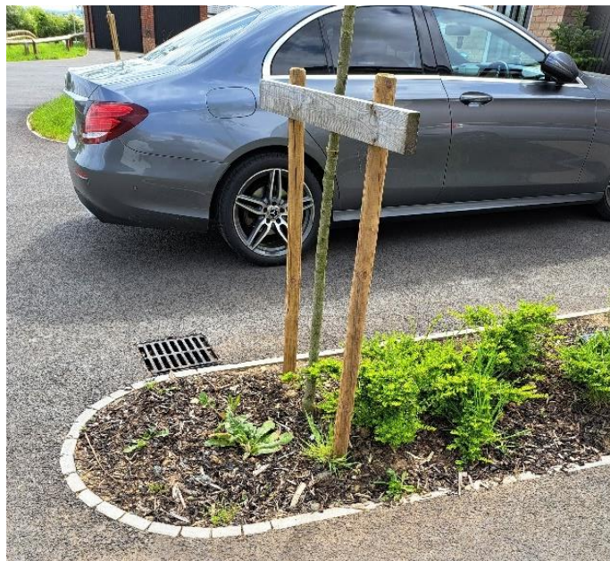
Figure 4 Poor planting practices to avoid: Restricted rooting volumes, impermeable surfacing and planting trees near underground services/drainage runs
