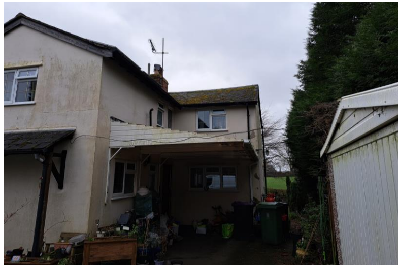
Figure 5: external of main building
