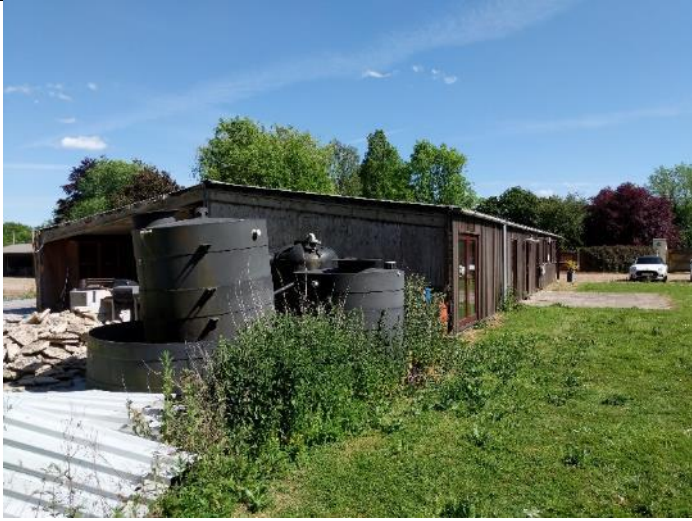
Photo 1 Former offices – south and west elevations
