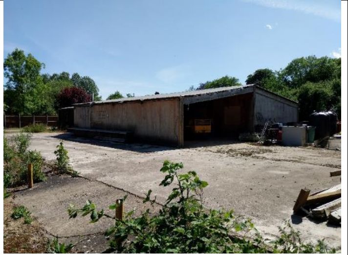
Photo 2 Former offices – north and west elevations
