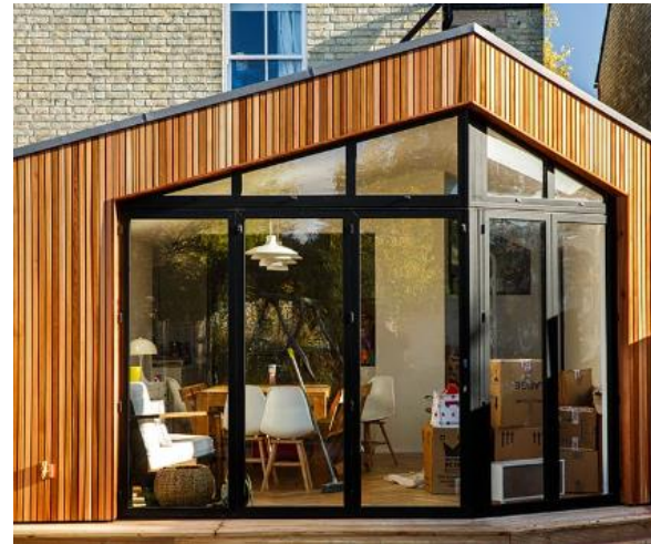
Figures 2 & 3 – Single storey vertically clad extensions.
