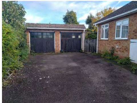
Photo 3 – View along eastern edge of garage and pathway
