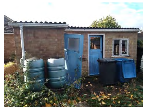
Photo 5 – View of the north side of the garages
