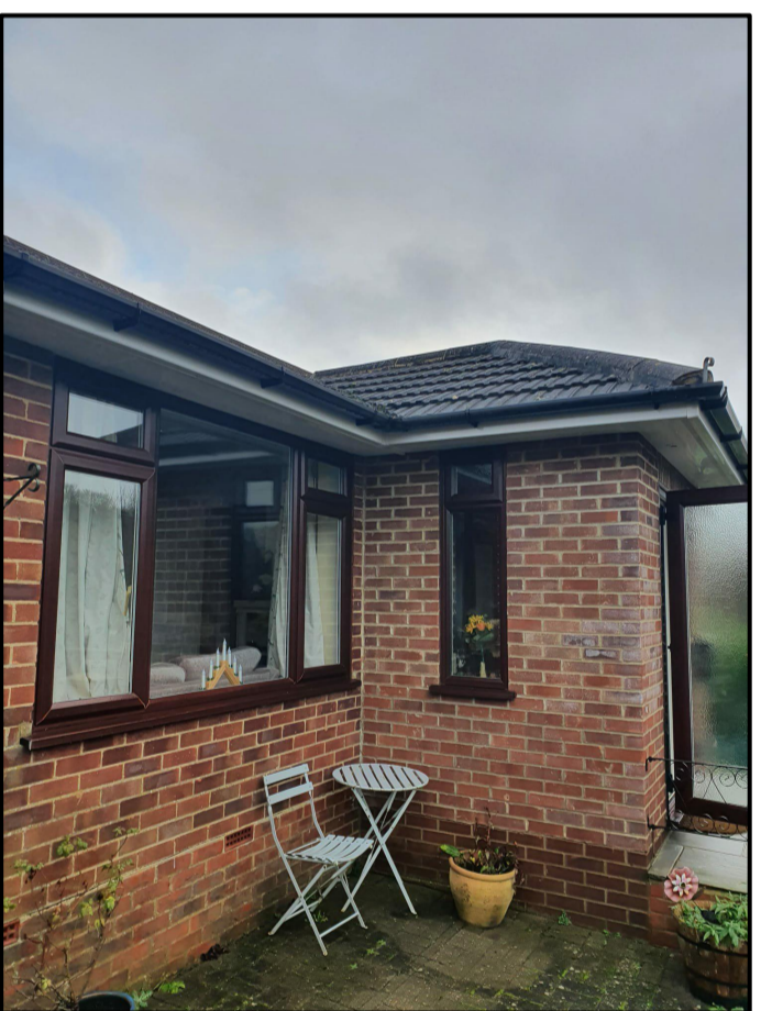
SIDE OF HOUSE LOOKING SOUTH/EAST
