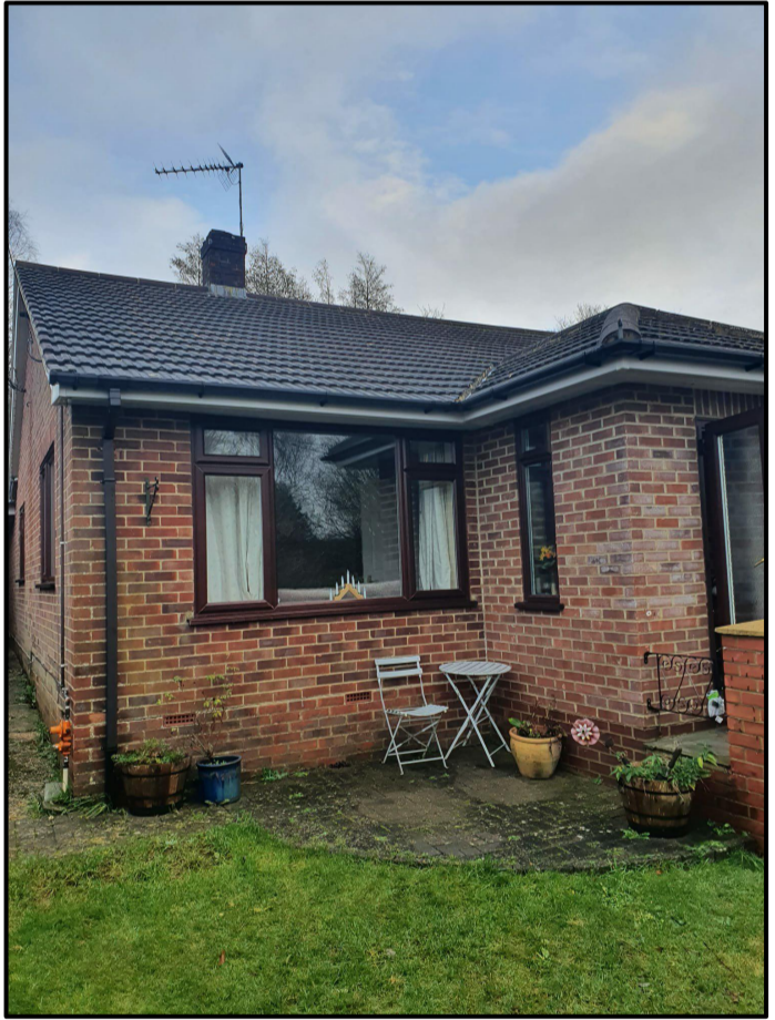
FRONT OF HOUSE LOOKING NORTH/EAST
