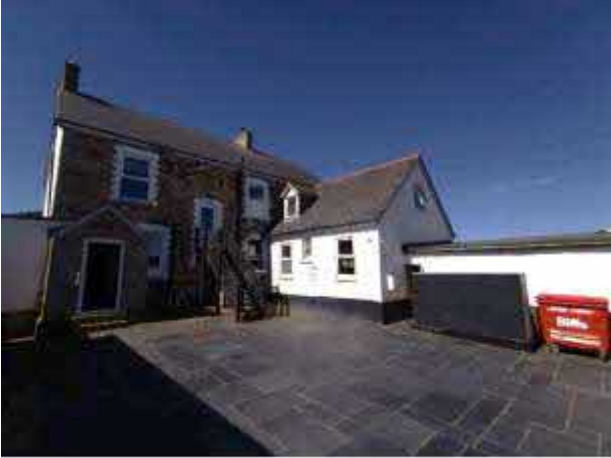
Photo 3. Showing the building from the North
