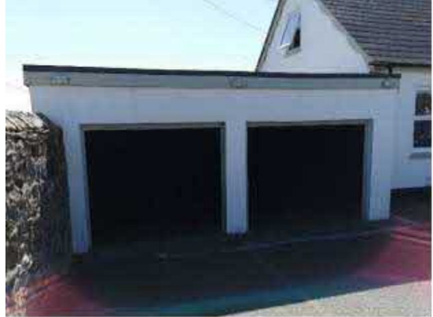
Photo 4. Showing the building from the West
