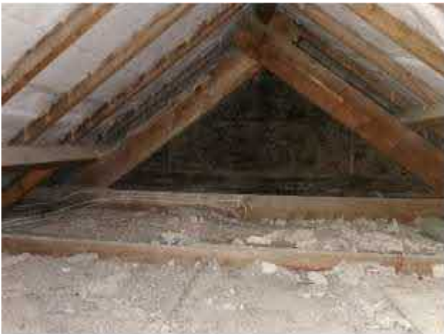
Photo 5. Showing the roof void over the main part
