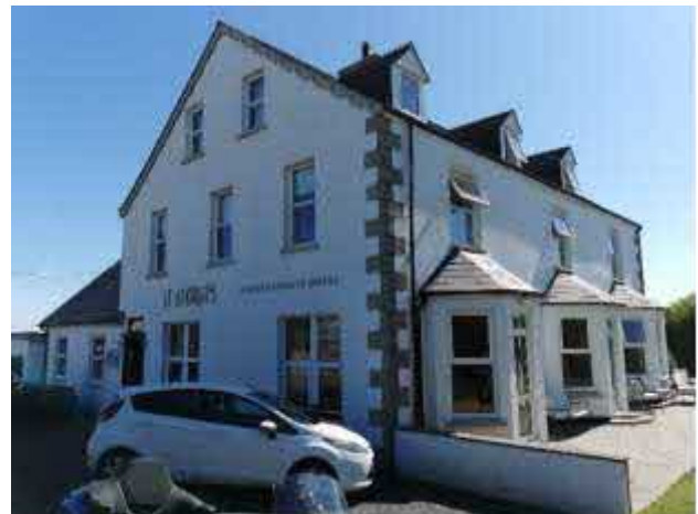
Photo 2. Showing the building from the West
