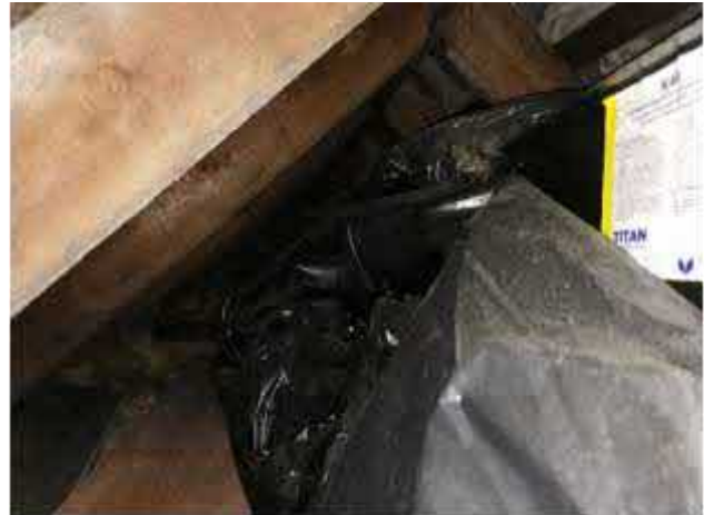
Photo 6. Showing the roof void over the annex of the building
