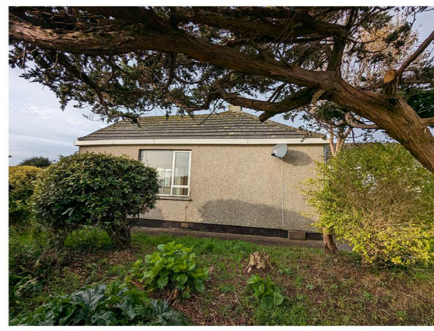
05 Photo: Side Elevation - East View
