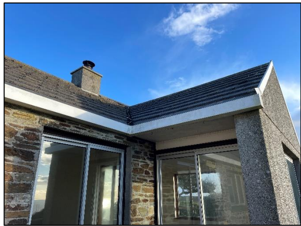
Figure Soffits and gables well sealed
