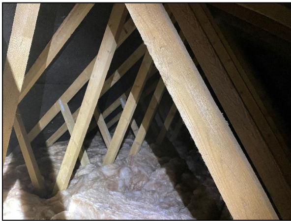
Figure 3 Interior of roof void
