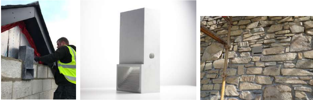
Photograph 6. Green and Blue' bat block and built in woodstone bat box `.
