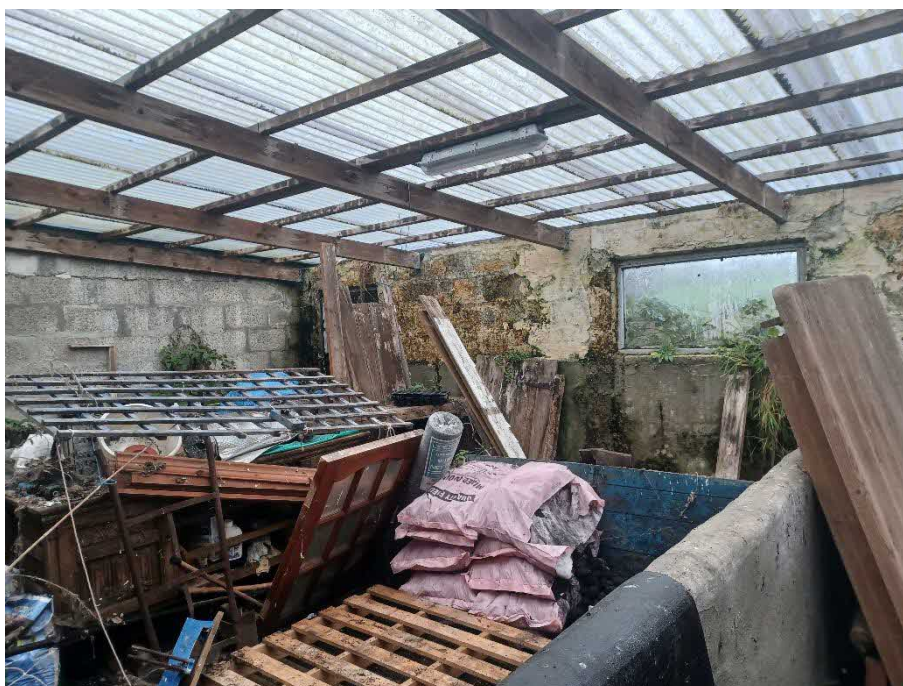
Figure 7: View of interior of Barn 2.
