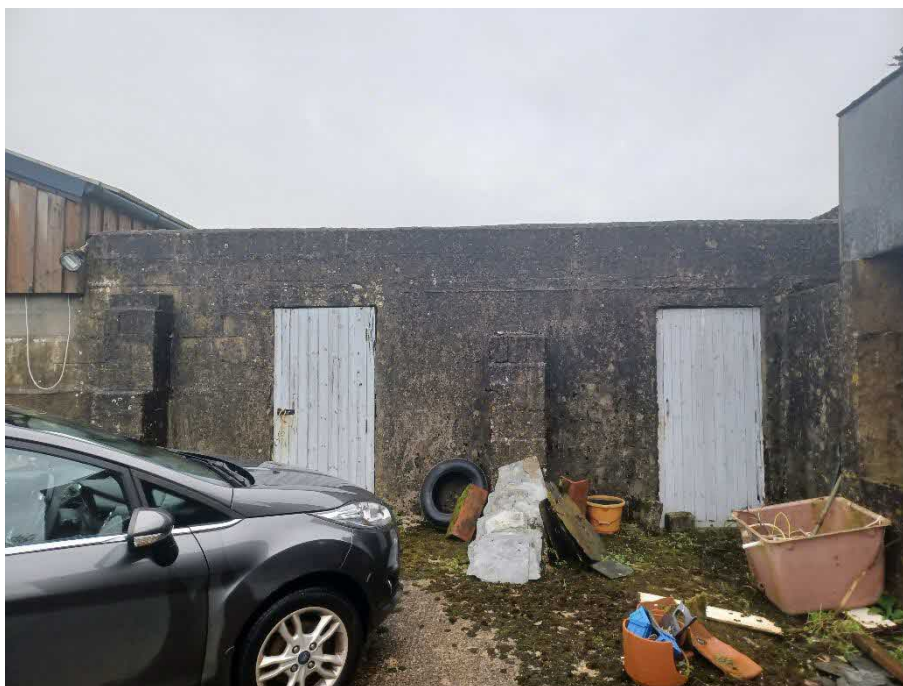
Figure 5: View of the west elevation of Barn 2.
