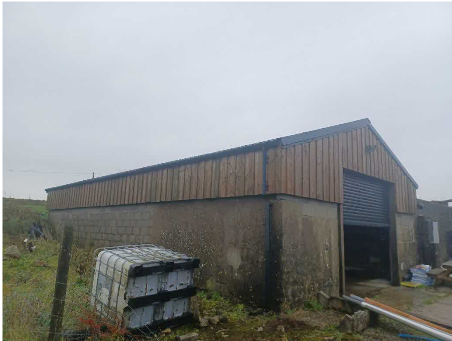
Figure 2: View of the north and west elevations of Barn 1.
