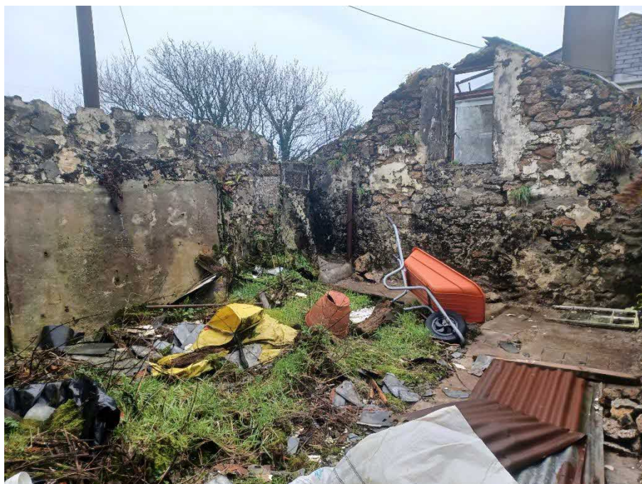
Figure 10: View of the western interior of Barn 3.
