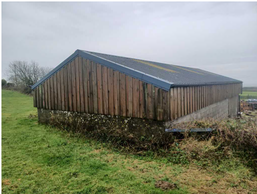
Figure 3: View of the north and east elevations of Barn 1.
