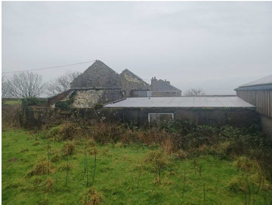
Figure 6: View of the east elevation of Barn 2.
