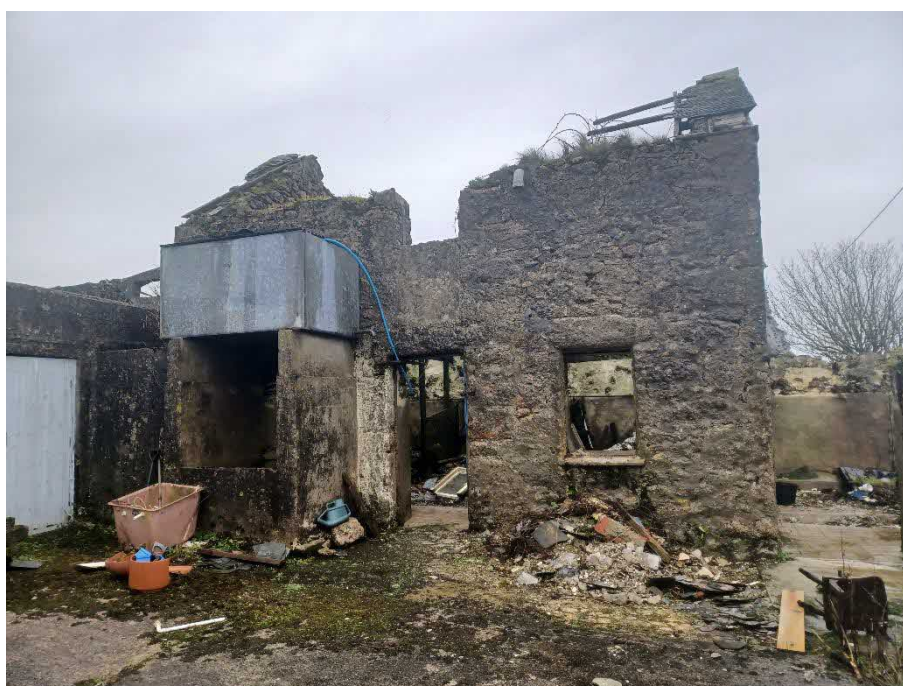
Figure 9: View of the north elevation of Barn 3.
