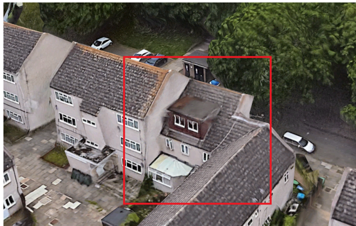
Fig. 3: No. 52 Poplar Place - Poor Example of a Rear Dormer Extension
