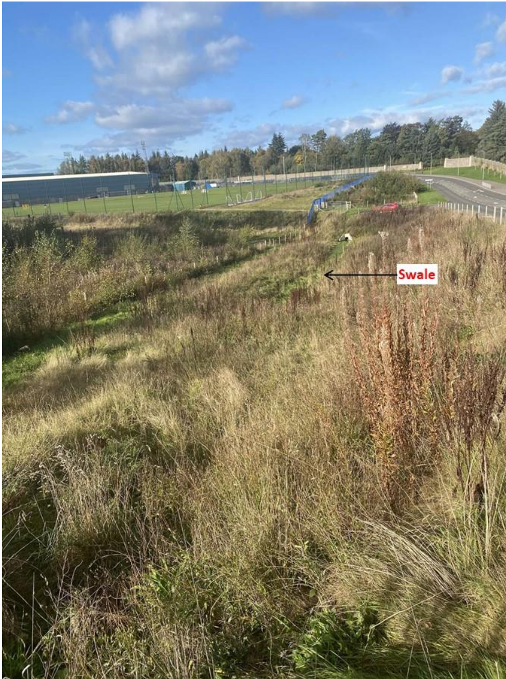
Photo 2: View looking north along edge of new road, showing swale and low point on road near to access to sports centre
