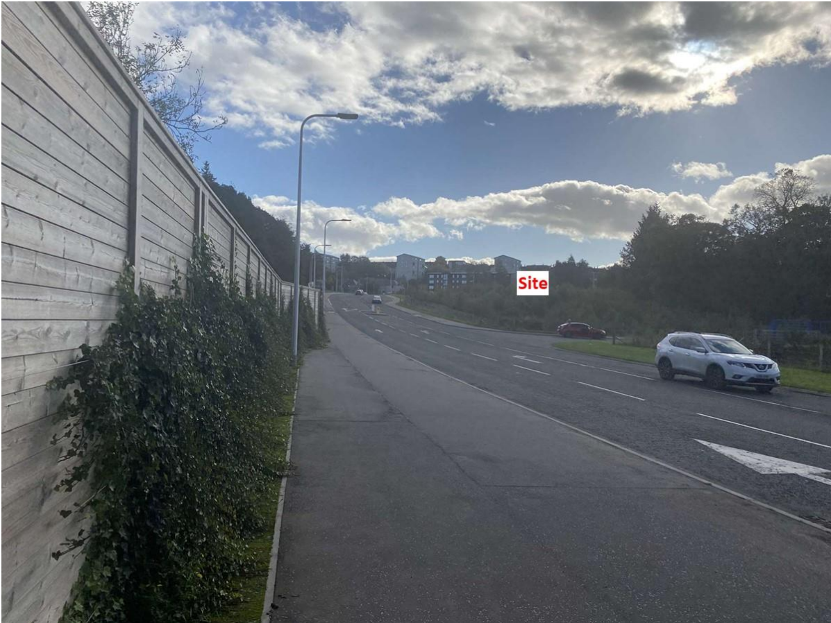
Photo 1: View south along new road, with site in distance
