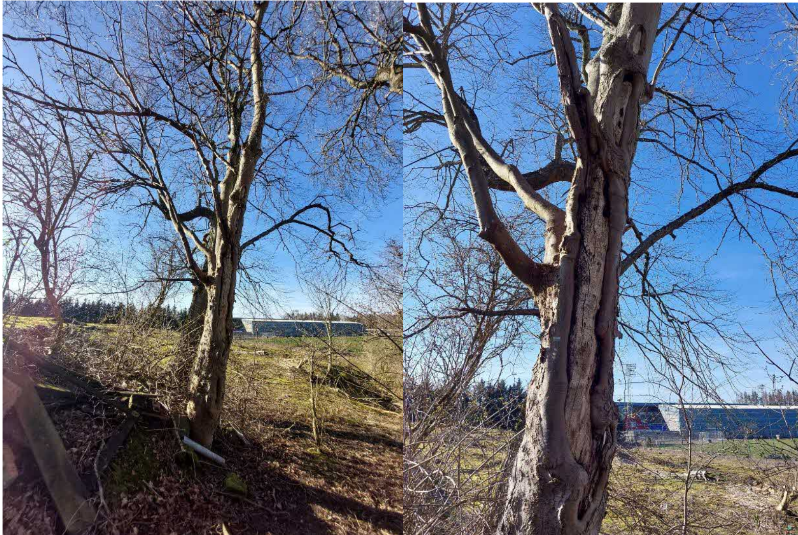
Photo 12 – Tree 5248 crack one eastern side of trunk
