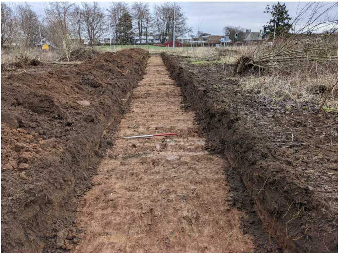
Plate 1 Typical post-excavation view of trench
