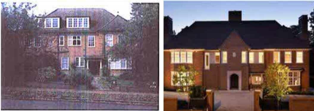
Comparison of works completed at No. 62 The Bishops Avenue (Jersey House)
