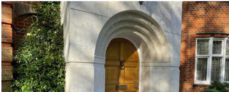
The existing porch
