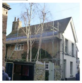
The roof covering is unfortunately now at the end of its useful life. The battens are completely rotten as seen within the roof structure and there is no underfelt. Continuous patch repairs have been carried out but due to the extent of rot to the battens complete recovering of the roof is necessary as during high winds, tiles are frequently dislodged and blown into the street below.
