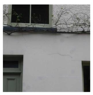
It is anticipated that the repairs to the cracking will be carried out using helical (twisted) stainless steel rods which can be concealed in the mortar joints and then be unseen. The extent of the cracking can be assessed once the render has been removed, in small areas to be agreed with the Conservation Officer of Dover District Council.
