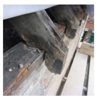
The proposal is to strip all the existing Kent Peg tiles and to salvage as many as possible. The roof will then be recovered with a modern underfelt, tanalised battens and then recovered with Kent Peg tiles.
