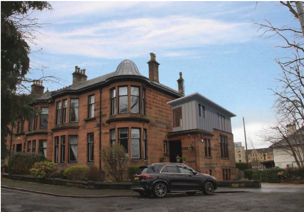
VIEW FROM HUGHENDEN DRIVE
