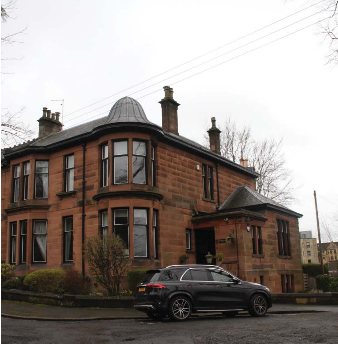
EXISTING HOUSE VIEWED FROM HUGHENDEN DRIVE
