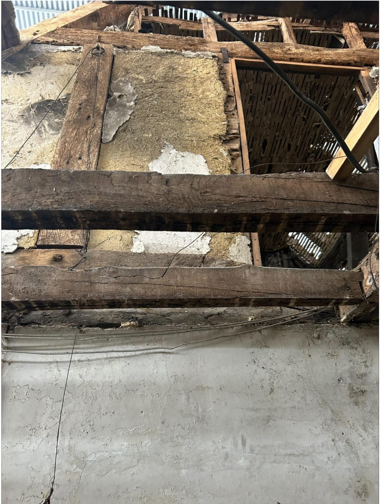
Loft room – re use daub on existing laths & new laths to head panels.
