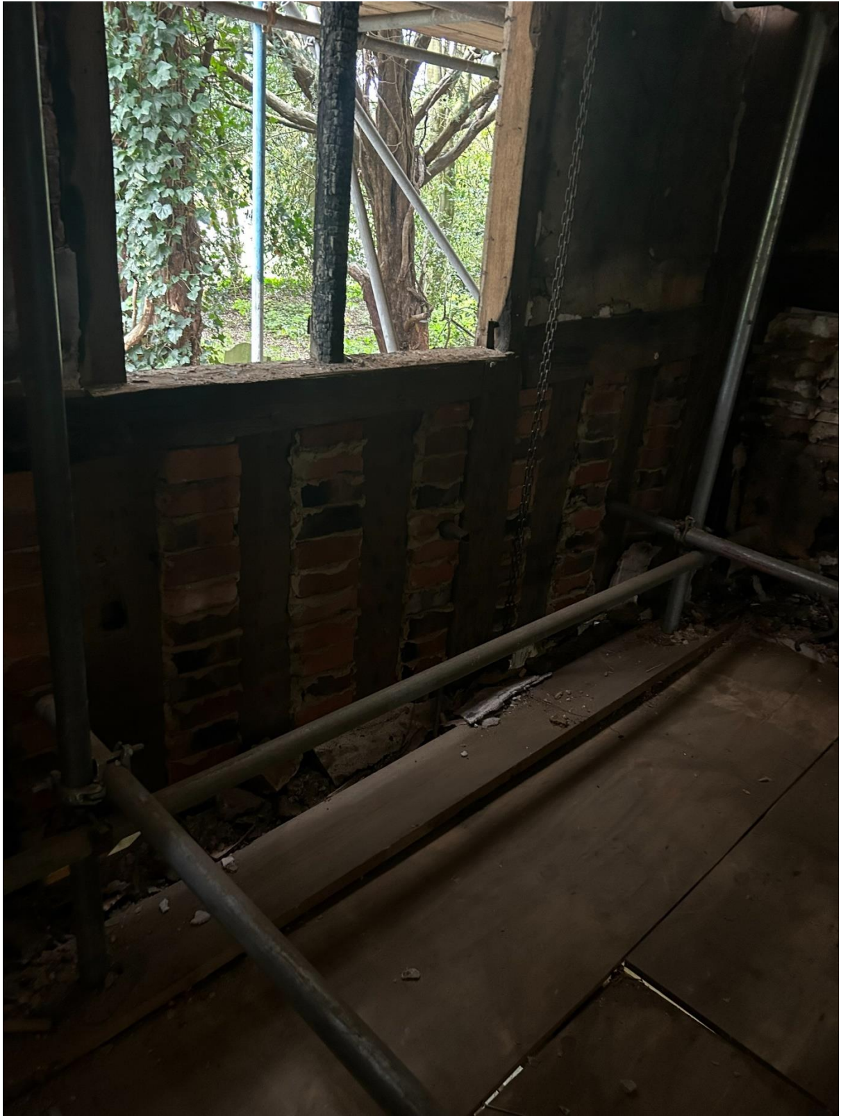
Daub to be reuse/new daub to the window walls.
