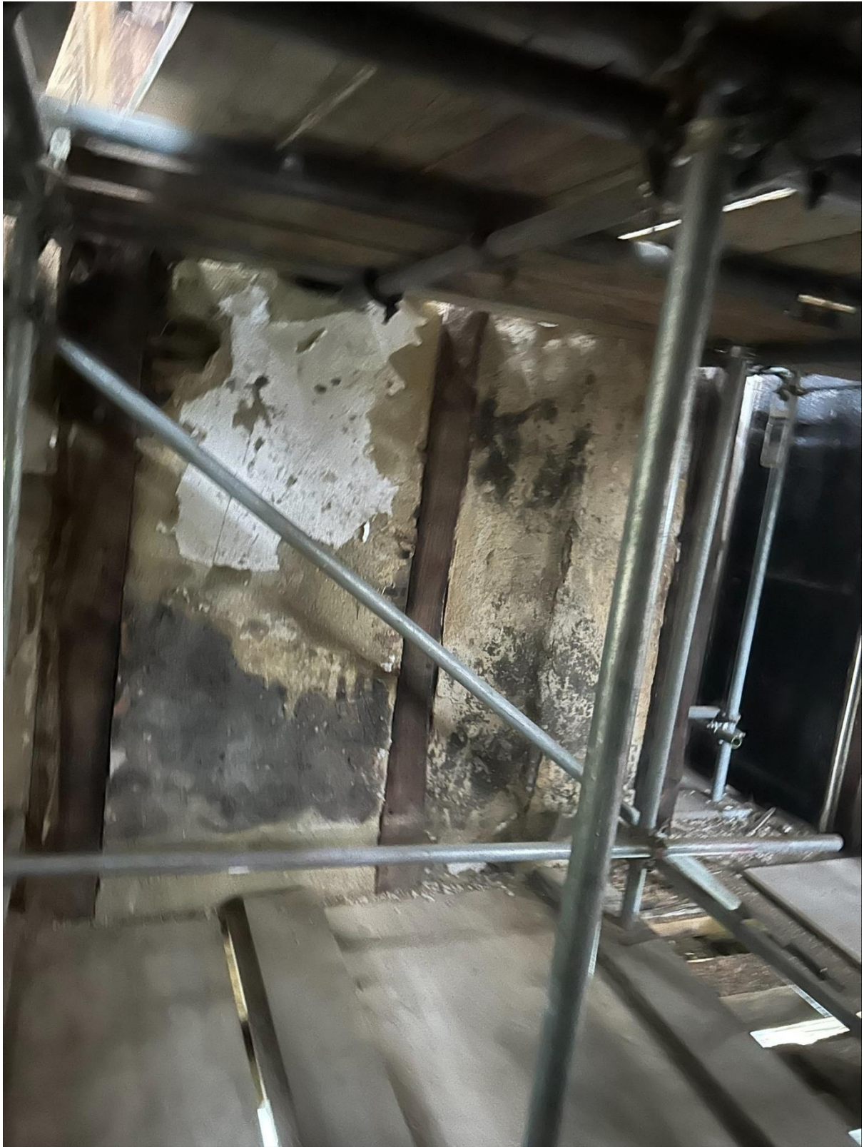
Daub removed and reused to the partition wall panels.
