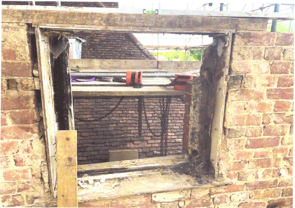
Structural opening left for W5
