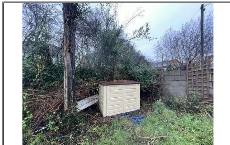
Photo OE/1702/1057/R2/P17 – Electrical box for supply to the site at southwest corner of the site.
