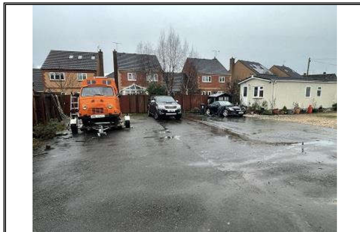
Photo OE/1702/1057/R2/P05 – View into the site from gated access from Alexander Road looking east, and residential housing beyond.
