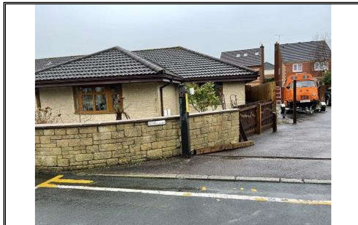
Photo OE/1702/1057/R2/P02 – Bungalow adjacent to the northern boundary of the site.
