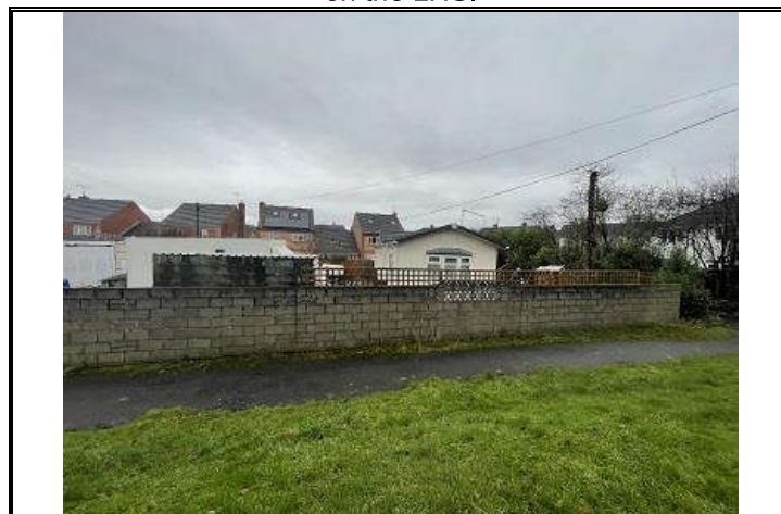
Photo OE/1702/1057/R2/P29 – View of southern section of western external brickwork boundary wall.
