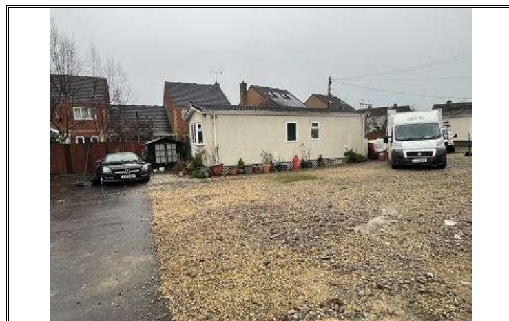
Photo OE/1702/1057/R2/P12 – View of 22a static caravan and transition from tarmac to rock fill surface dressing.
