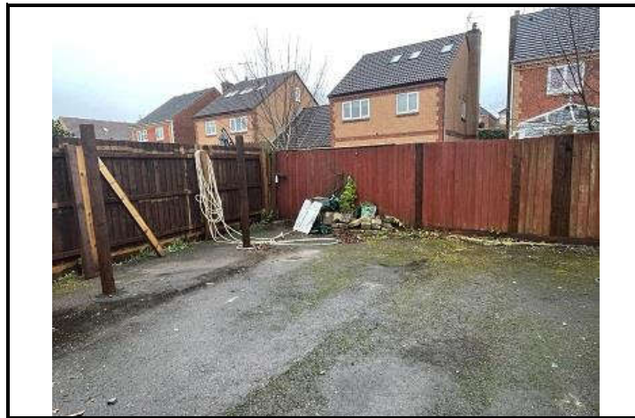
Photo OE/1702/1057/R2/P07 – Northeast corner of the site and residential housing beyond .
