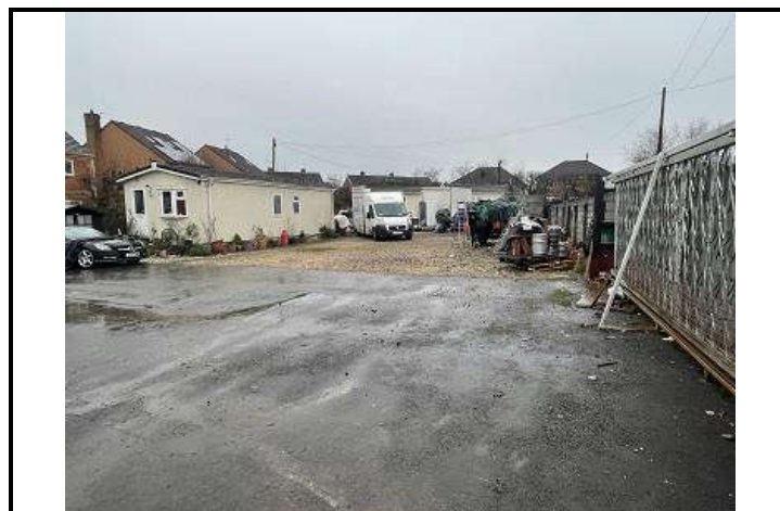
Photo OE/1702/1057/R2/P06 – Look south down the site from gated access.
