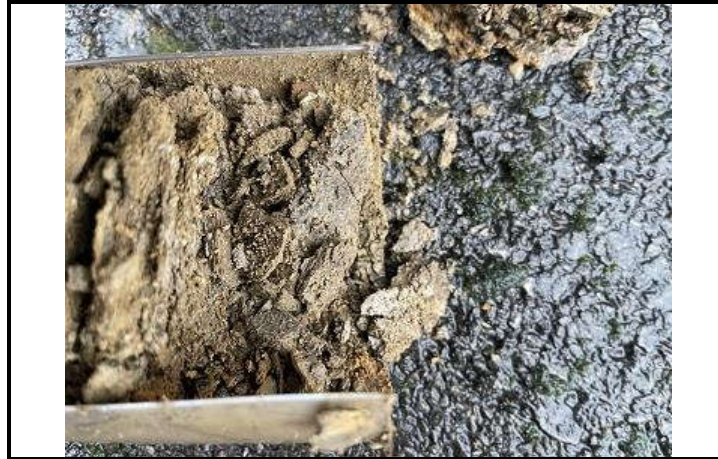
Photo OE/1702/1057/R3/P19 – Window Sample WS2 – Drilling core at 1.6m bgl – Very stiff weathered Mudstone.
