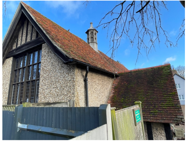
Photograph 2: Front and side elevations of the property.
