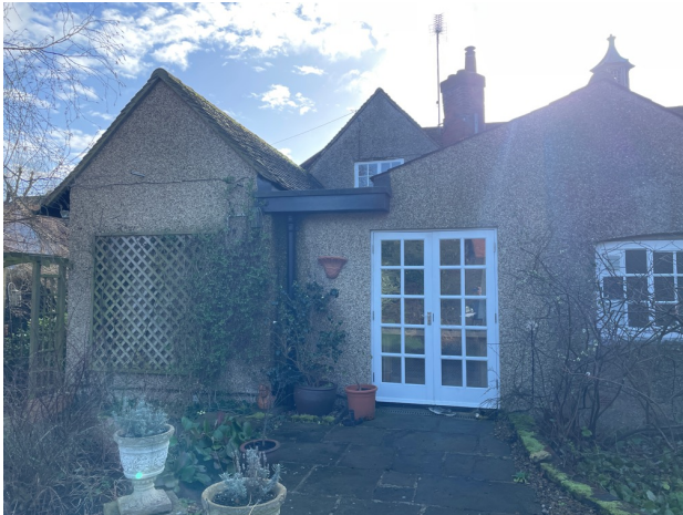
Photograph 3: Rear elevation of the property.
