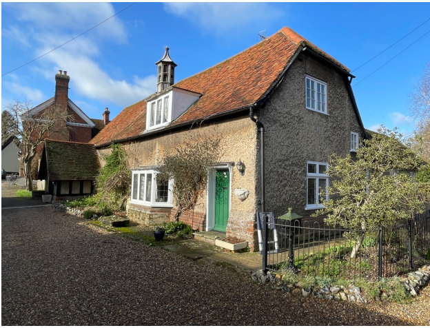
Photograph 1: Front and side elevations of the property.
