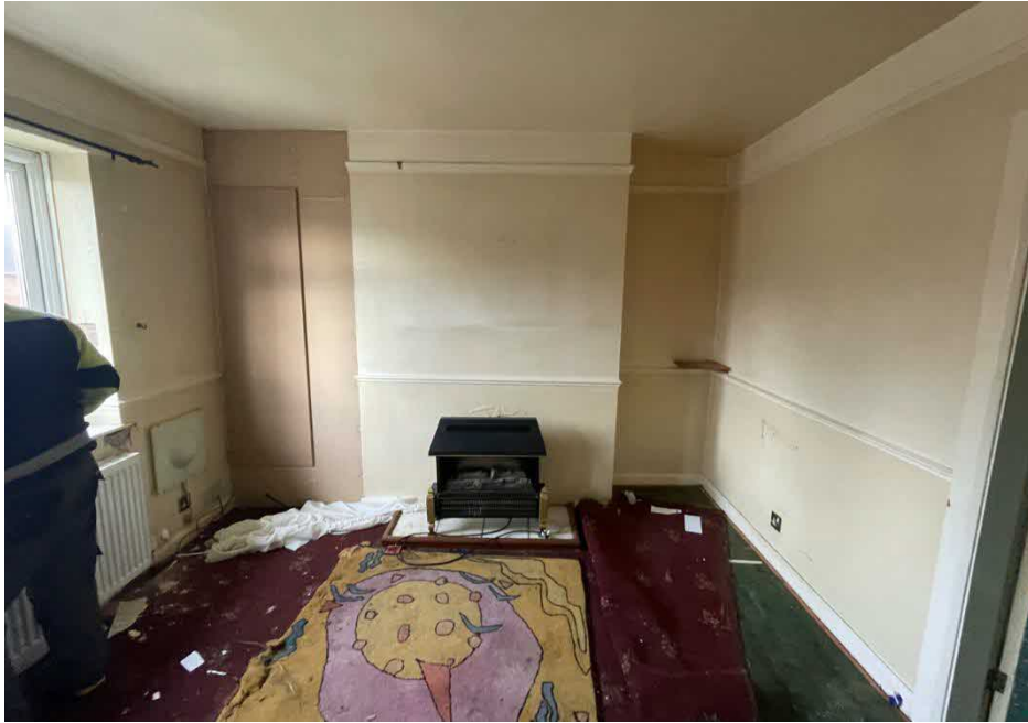
Photograph 9. First Floor Living Area
