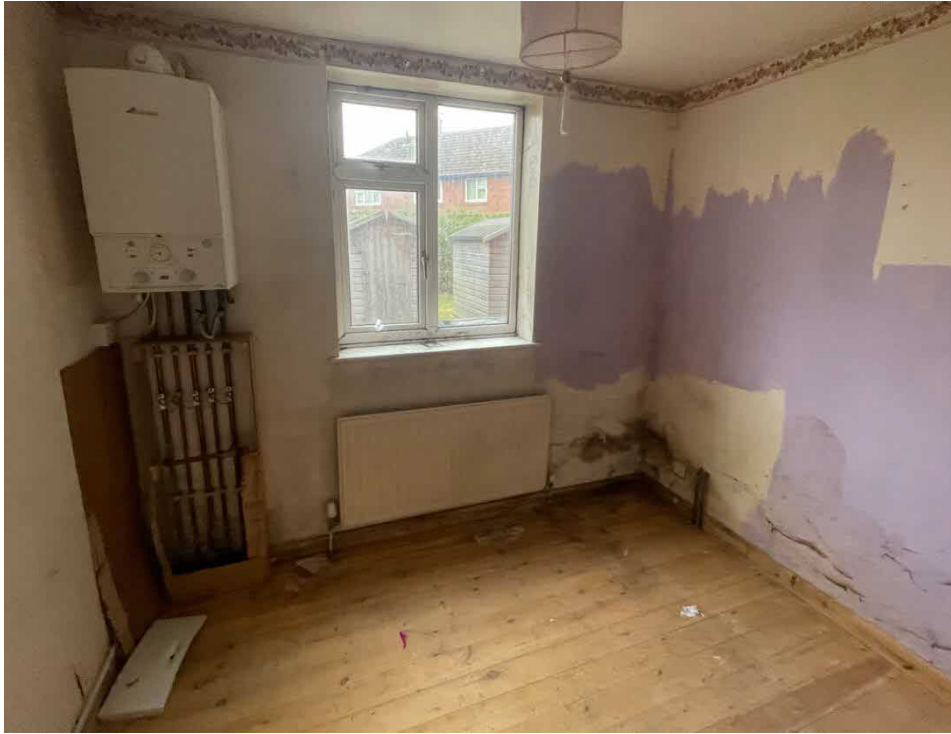
Photograph 3. Ground Floor Bedroom Facing Rear
