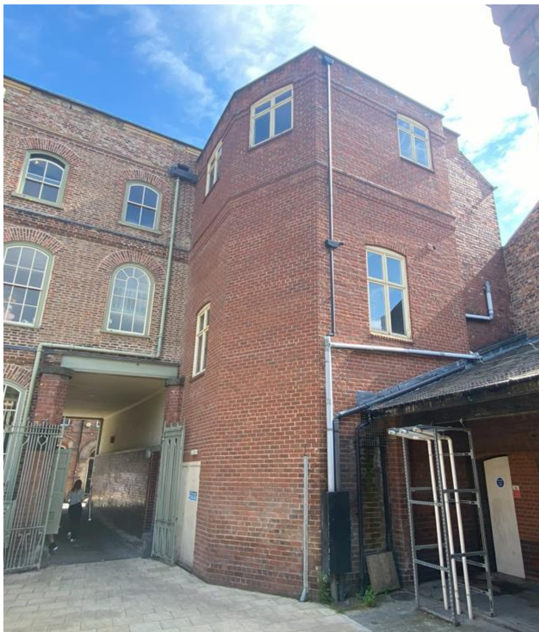
Extension to the rear of 18 Lendal The lean to and fire exit within the lean to form part of the former post office demise wrapping around the back of the premises.
