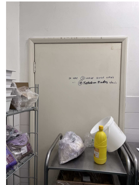
01. NON LOADBEARING WALLS REMOVED
