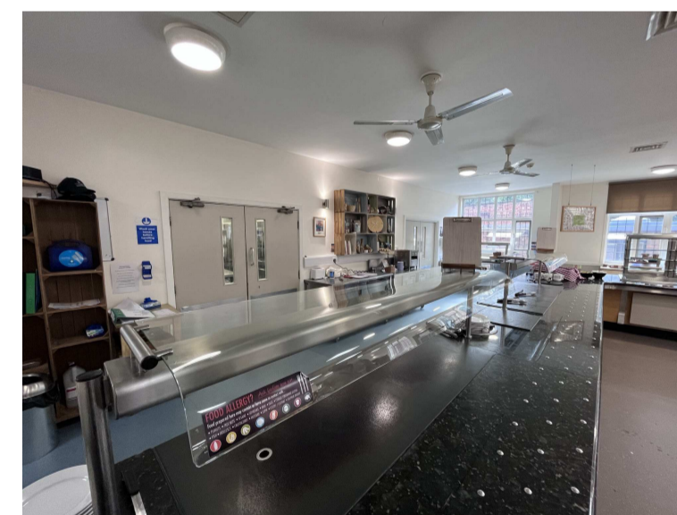
03. EXISTING PARTITION BETWEEN KITCHEN AND SERVERY REMOVED
