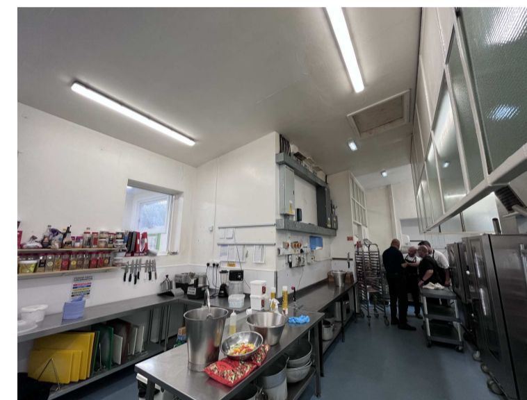
02. NON LOADBEARING WALL REMOVED
