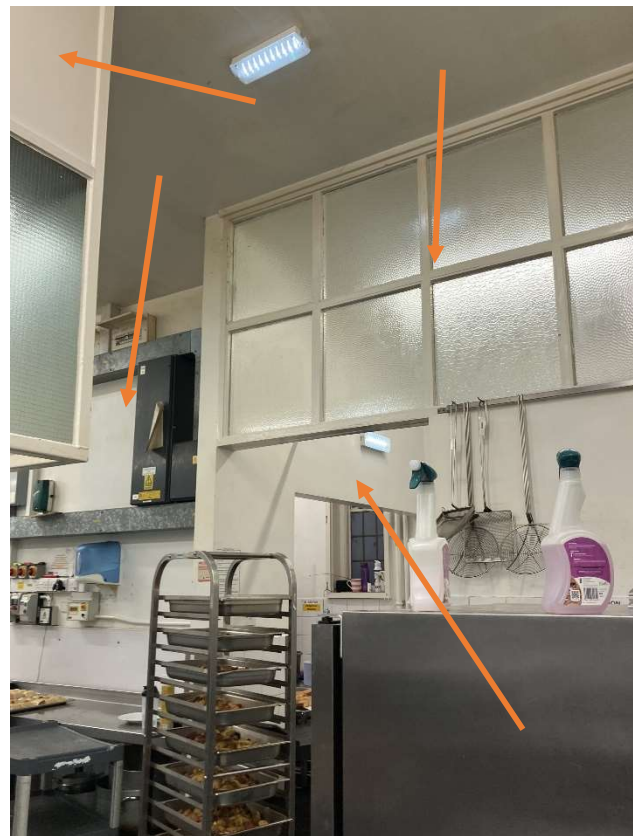
MASONRY WALLS/HIGH LEVEL GLAZED SCREENS TO BE REMOVED (arrowed)
