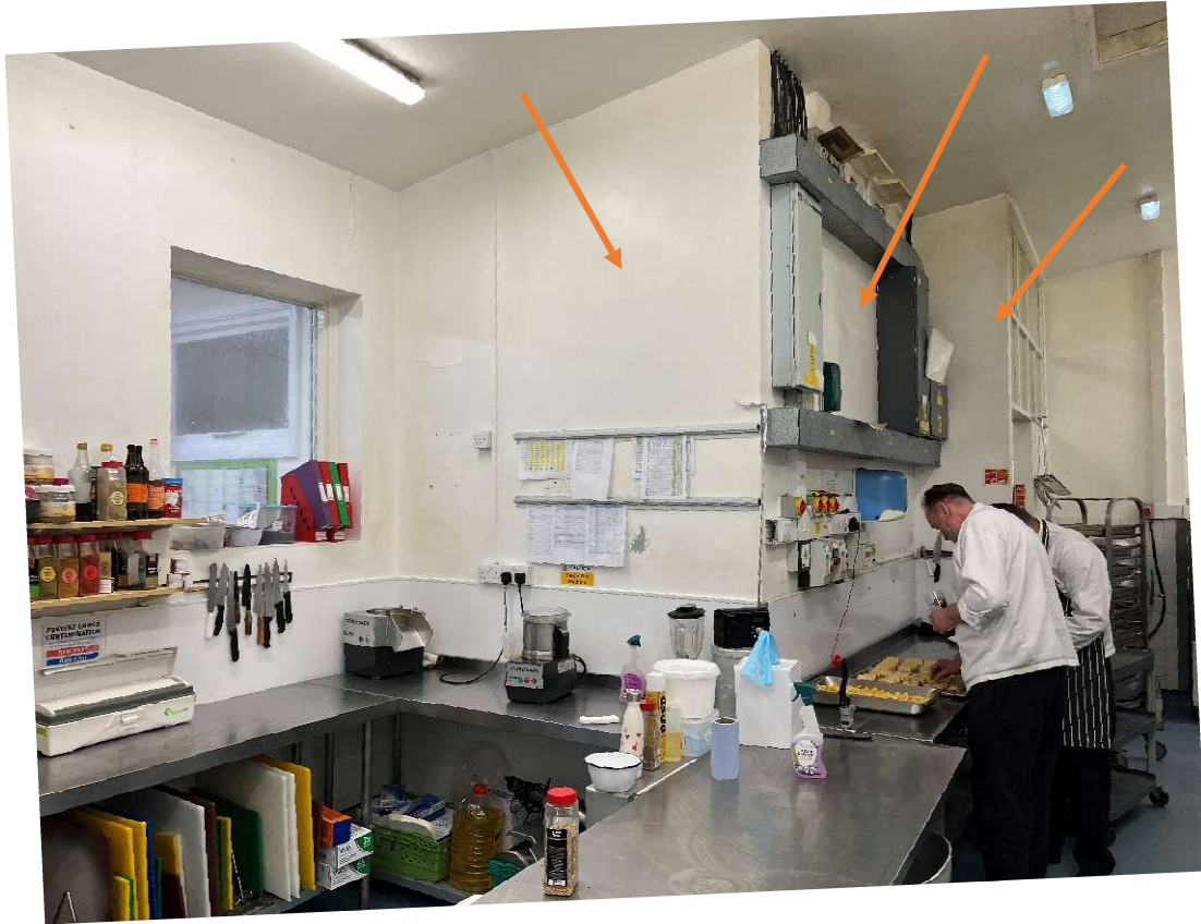
MASONRY WALLS TO BE REMOVED (arrowed); WALL TO LEFT HAS WINDOW INTO ROOM WHICH ABUTS EAST WALL OF SCHOOL HOUSE; WINDOW WILL BECOME PART OF EXTENDED DINING AREA
