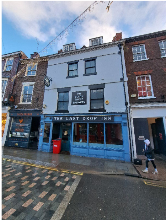
Existing Street frontage
