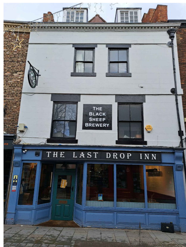
Signage as Existing
